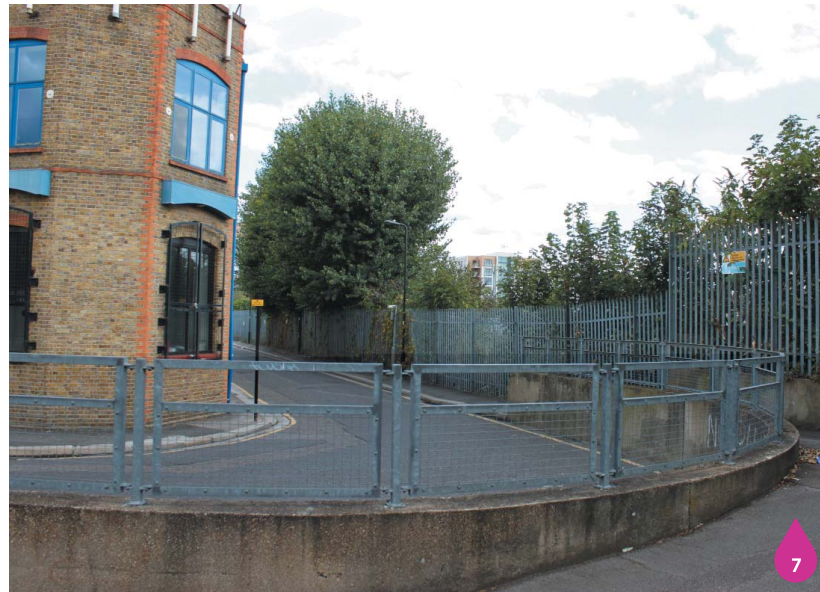
Figure 6.10: Northern corner of the proposed site
