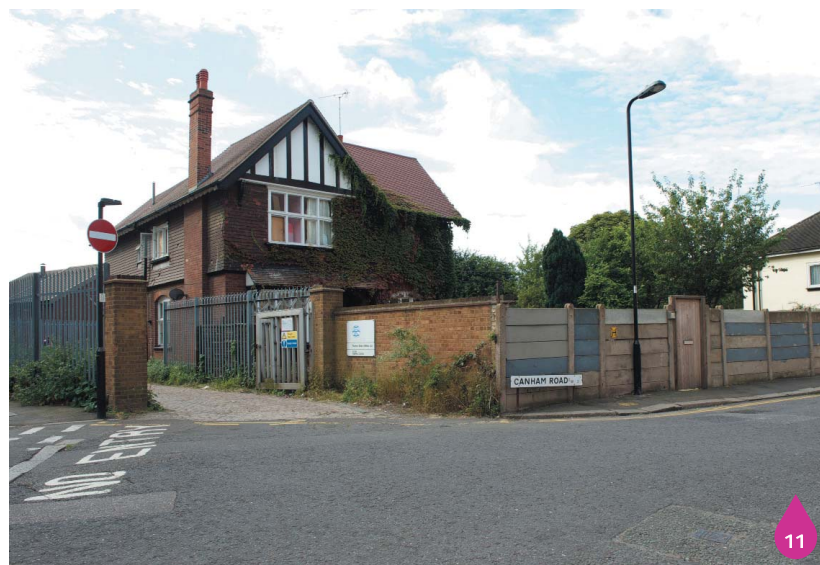
Figure 6.14: Existing entrance to storm tank site
