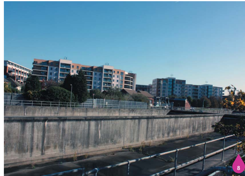
Figure 6.11: Storm tanks with Warple Way beyond
