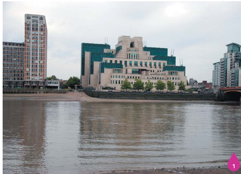
Figure 18.3: Existing site upstream of Vauxhall Bridge
