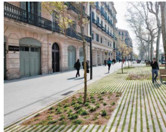
Figure 18.64: Permeable natural stone paving
