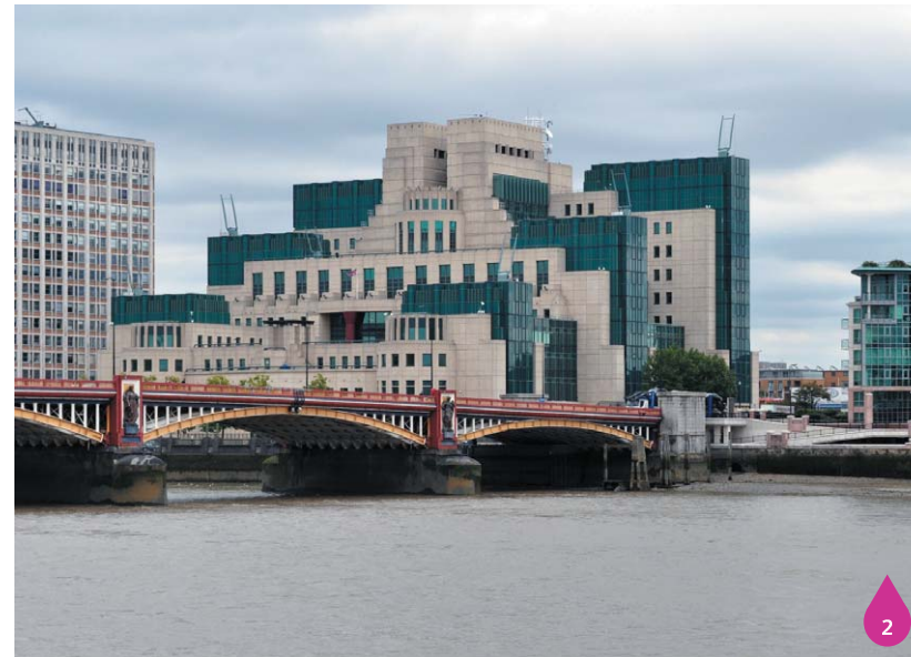
Figure 18.4: Existing site downstream of Vauxhall Bridge
