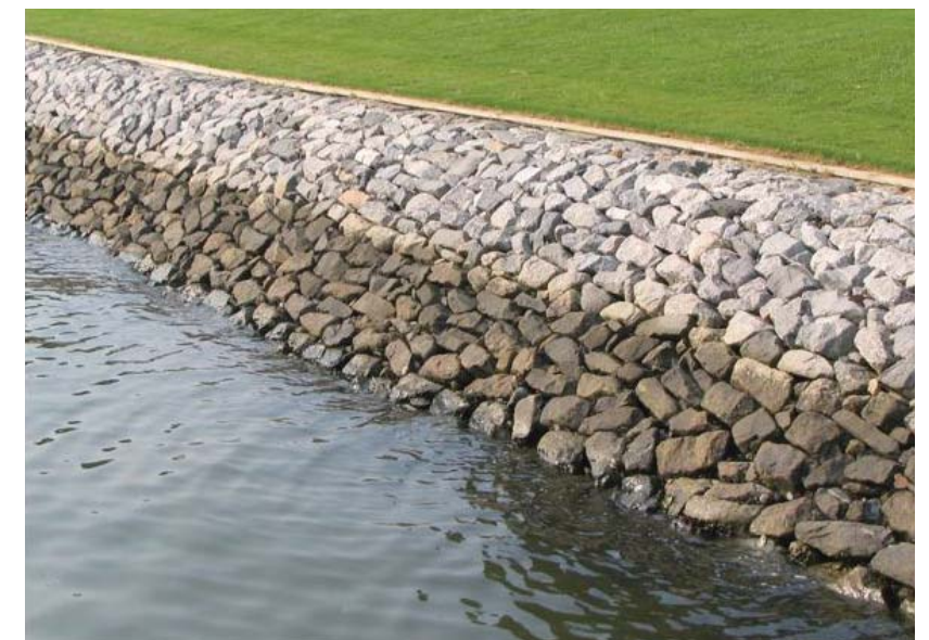
Figure 18.48: Example of 'rip rap' scour protection
