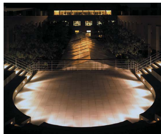
Figure 18.55: Example of recessed wall luminaires
