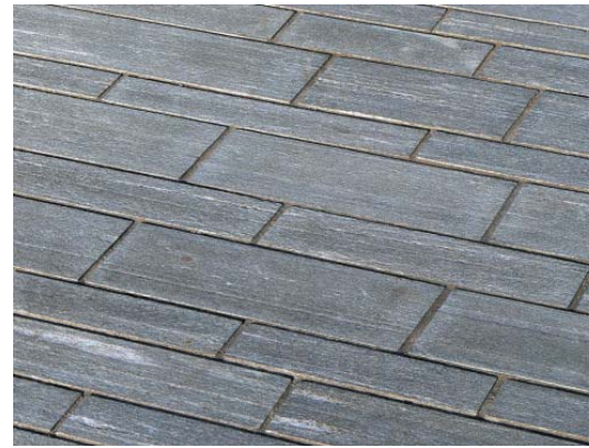
Figure 18.62: Example of natural stone paving
