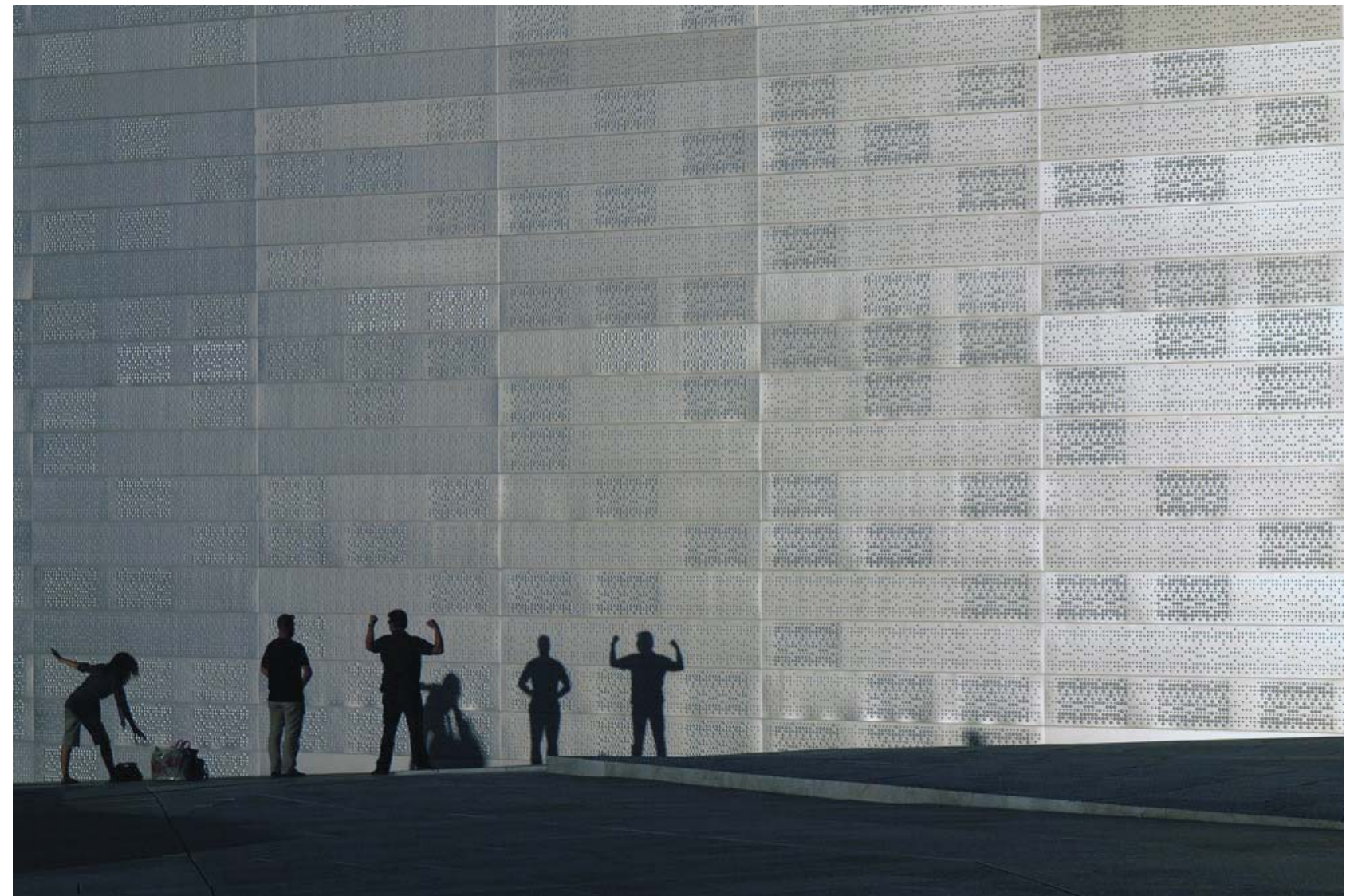
Figure 20.43: Example of a perforated metal screen
