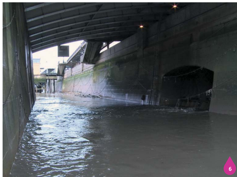
Figure 20.8: Fleet Main CSO outfall under Blackfriars Bridge
