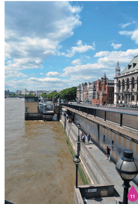
Figure 20.14: Paul's Walk towards Blackfriars Millennium Pier
