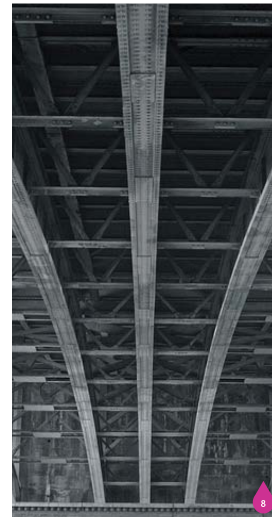
Figure 20.10: Underside of Blackfriars Bridge
