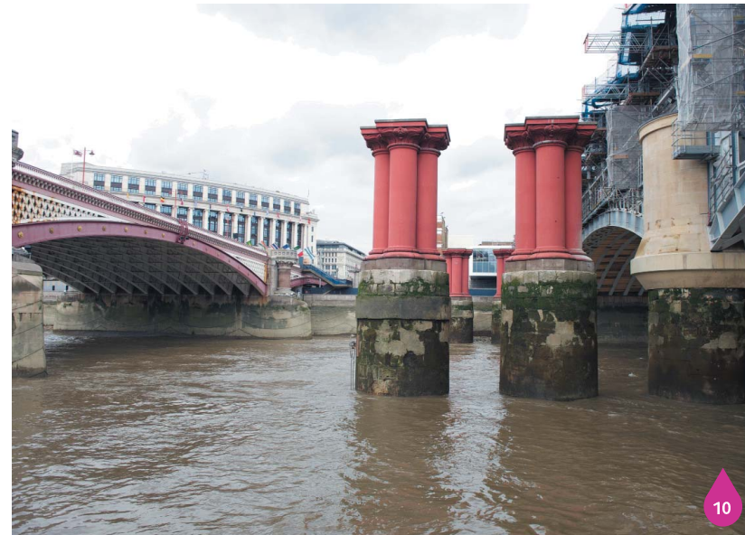
Figure 20.13: Blackfriars Bridge from River Thames looking northwest
