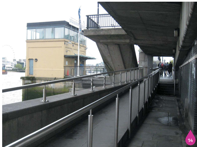
Figure 20.17: Paul's Walk underneath Victoria Embankment
