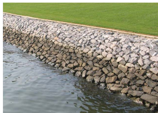
Figure 20.57: Example of 'rip rap' wall
