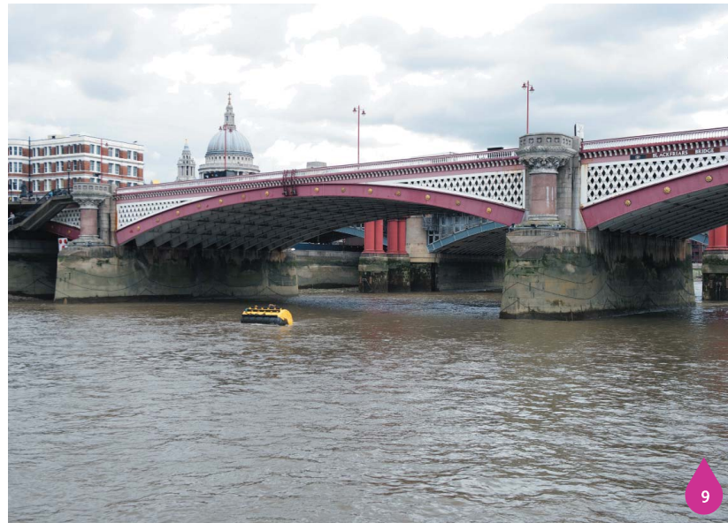
Figure 20.12: Blackfriars Bridge from the River Thames looking northeast
