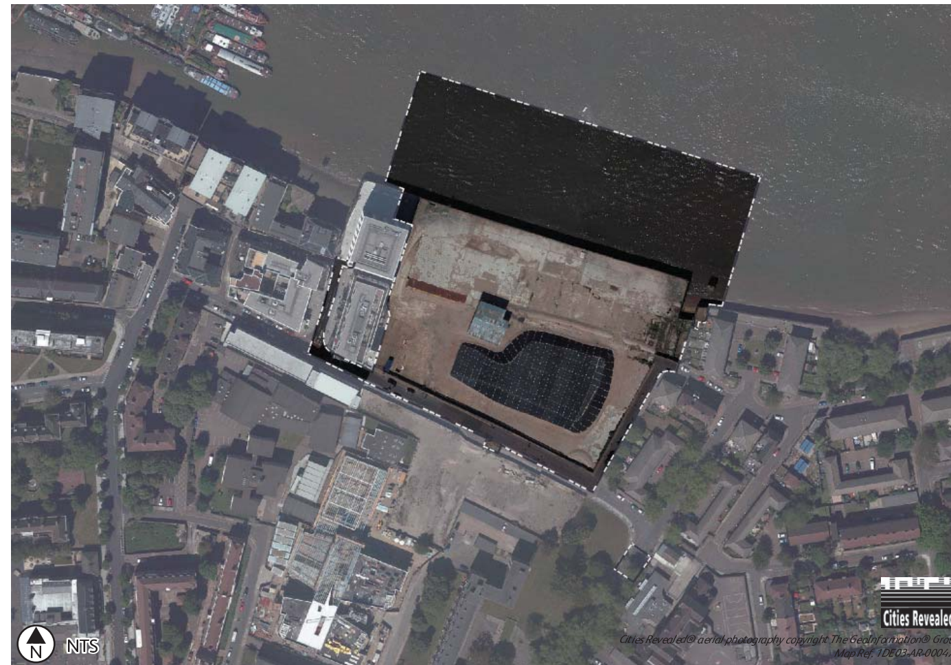
Figure 22.1: Aerial photograph of the existing Chambers Wharf site with LLAU indicated
