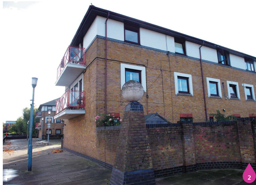
Figure 22.4: View east of Fountain Green Square
