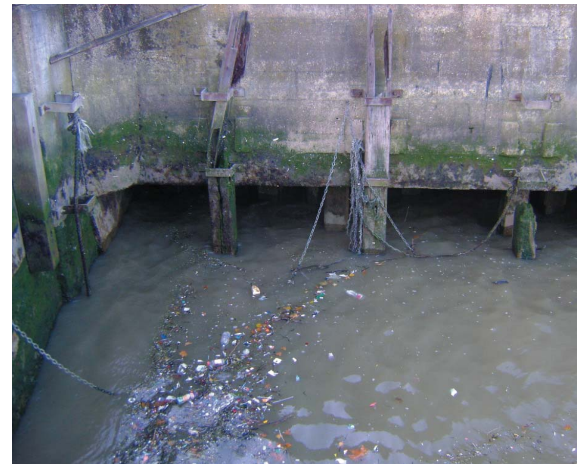
Figure 22.31: Existing Chamber's Wharf river wall/jetty
