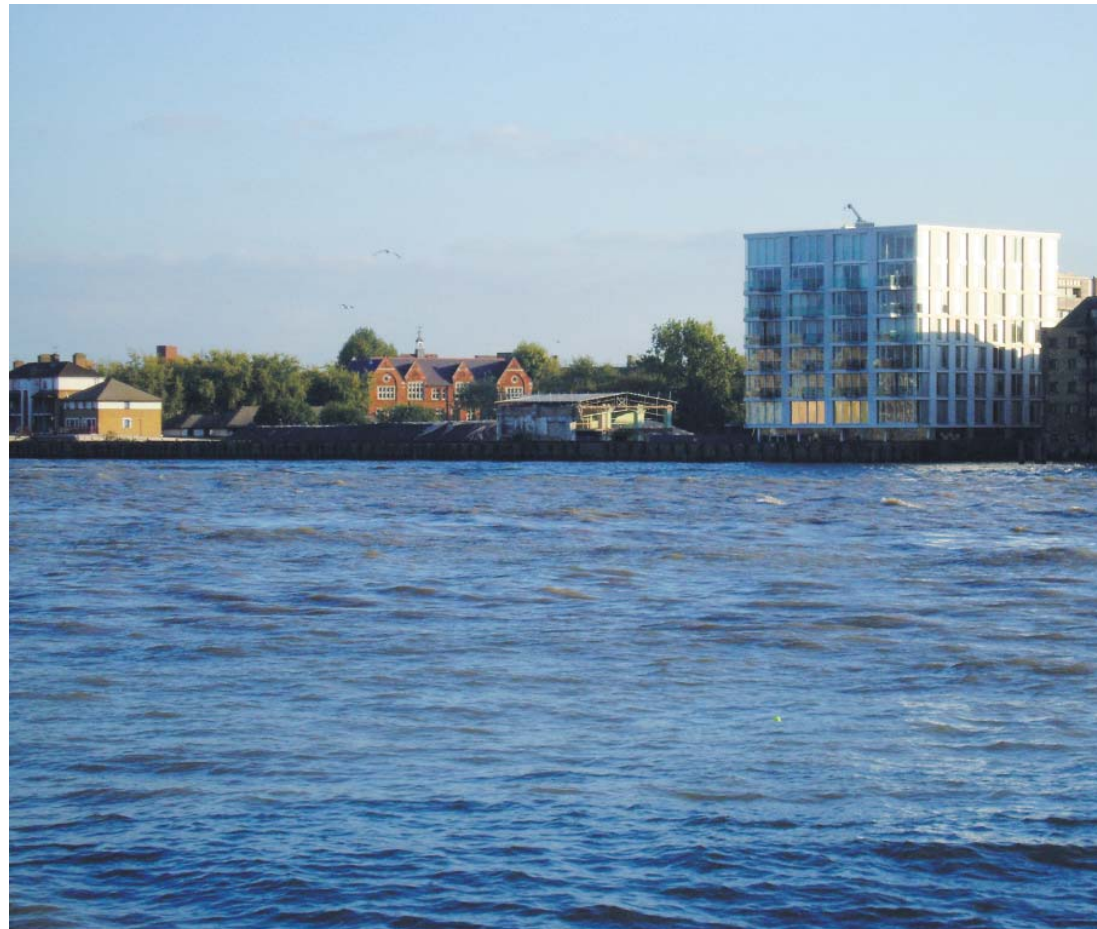
Figure 22.28: Existing Chamber's Wharf site foreshore
