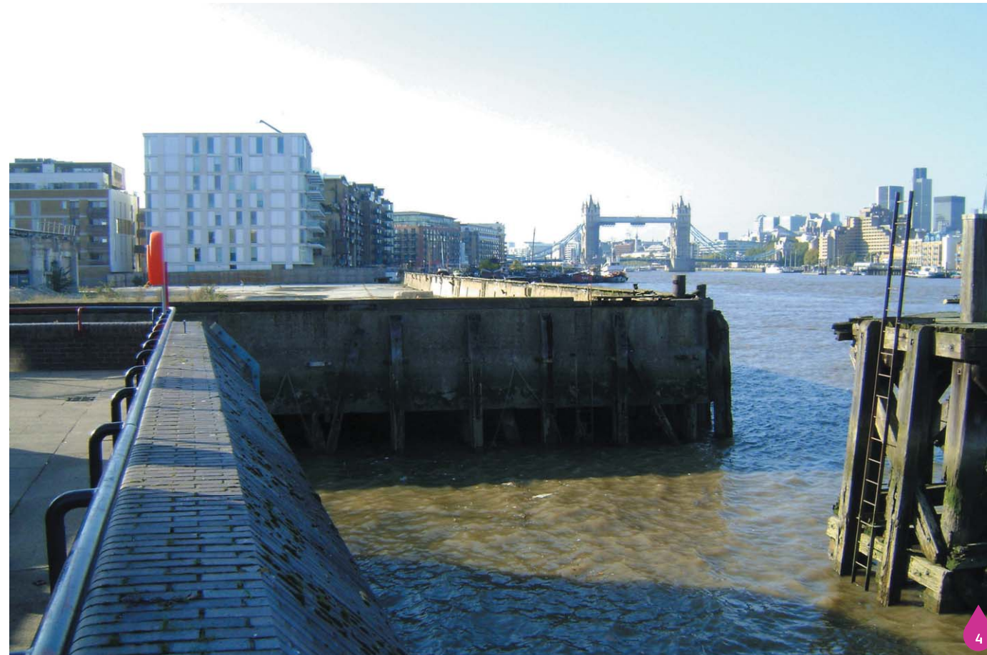
Figure 22.6: Existing river wall and jetty
