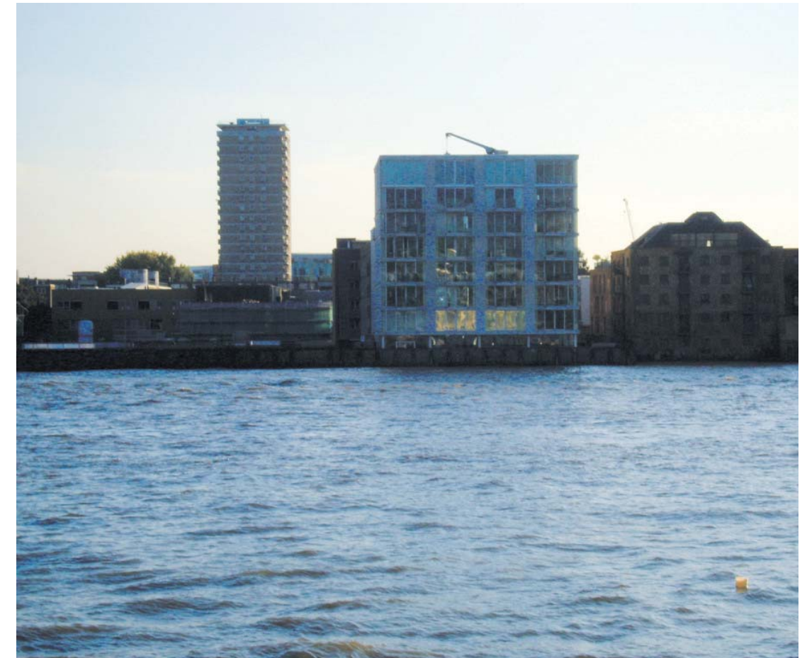
Figure 22.39: Existing Chamber's Wharf site foreshore
