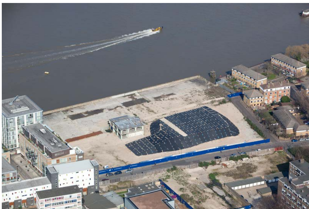
Figure S.1 Aerial photograph of Chambers Wharf
