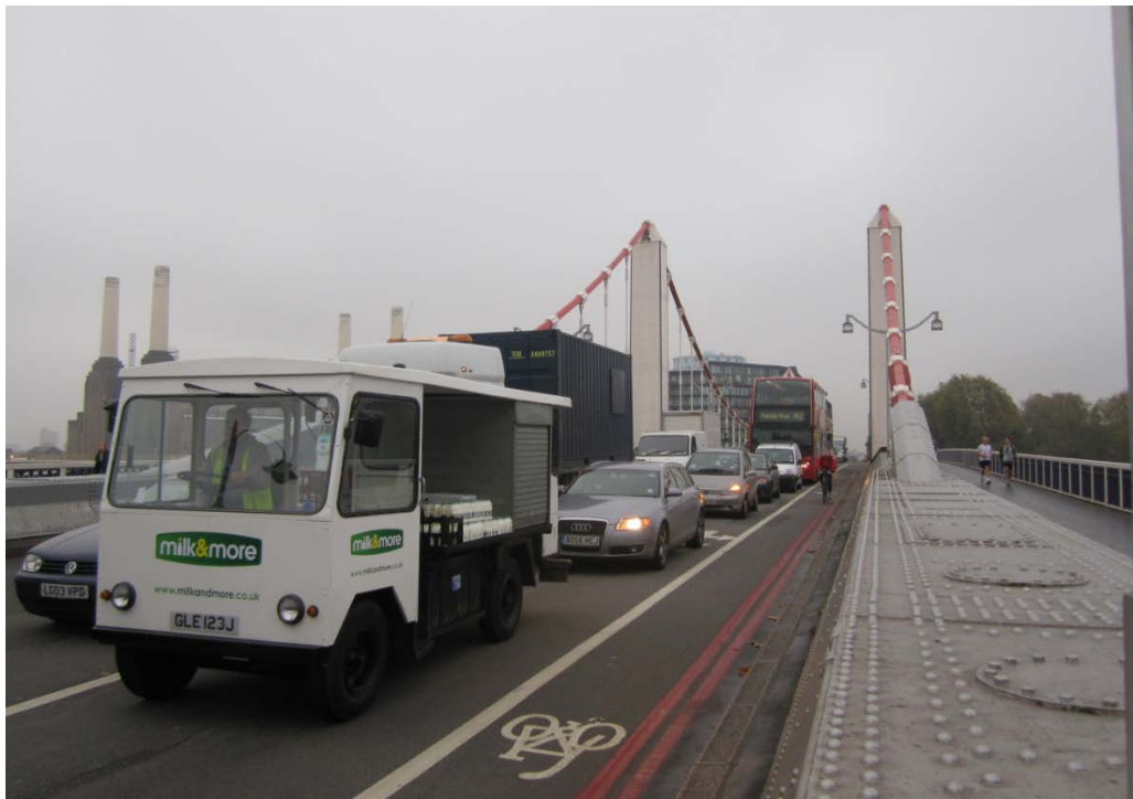
Plate 13.4.3 Cycle lane south facing along Chelsea Bridge (A3216)
