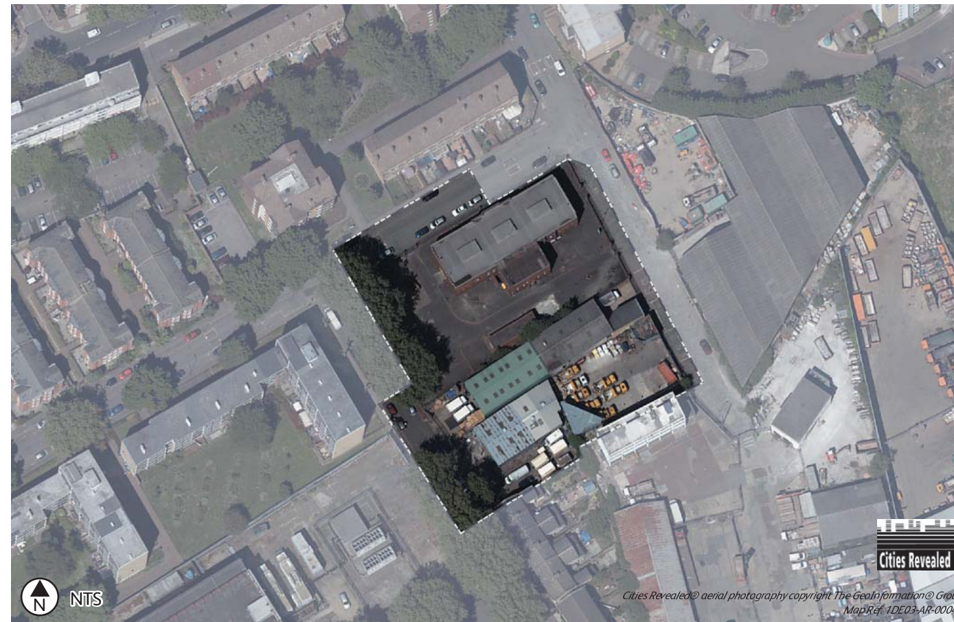
Figure 24.1: Aerial photograph of the existing Earl Pumping Station site with LLAU indicated
