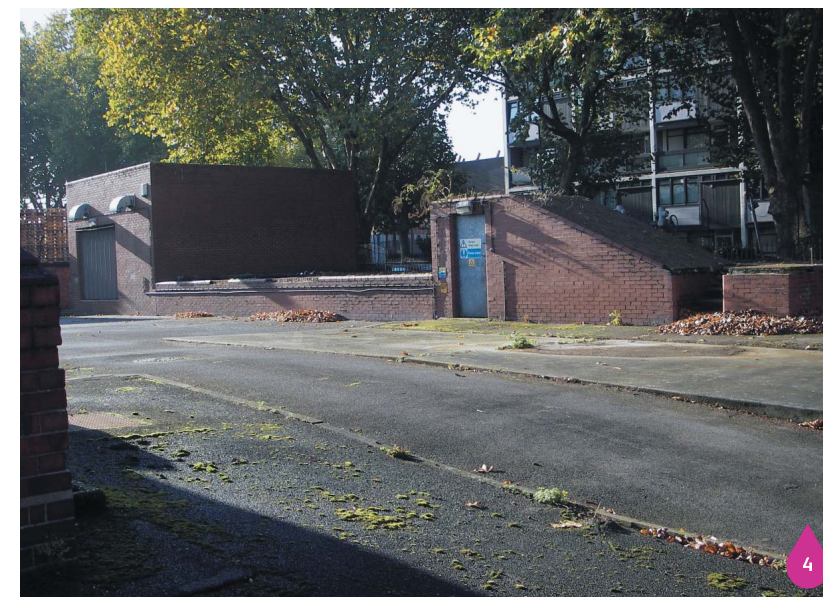
Figure 24.6: Existing site looking South
