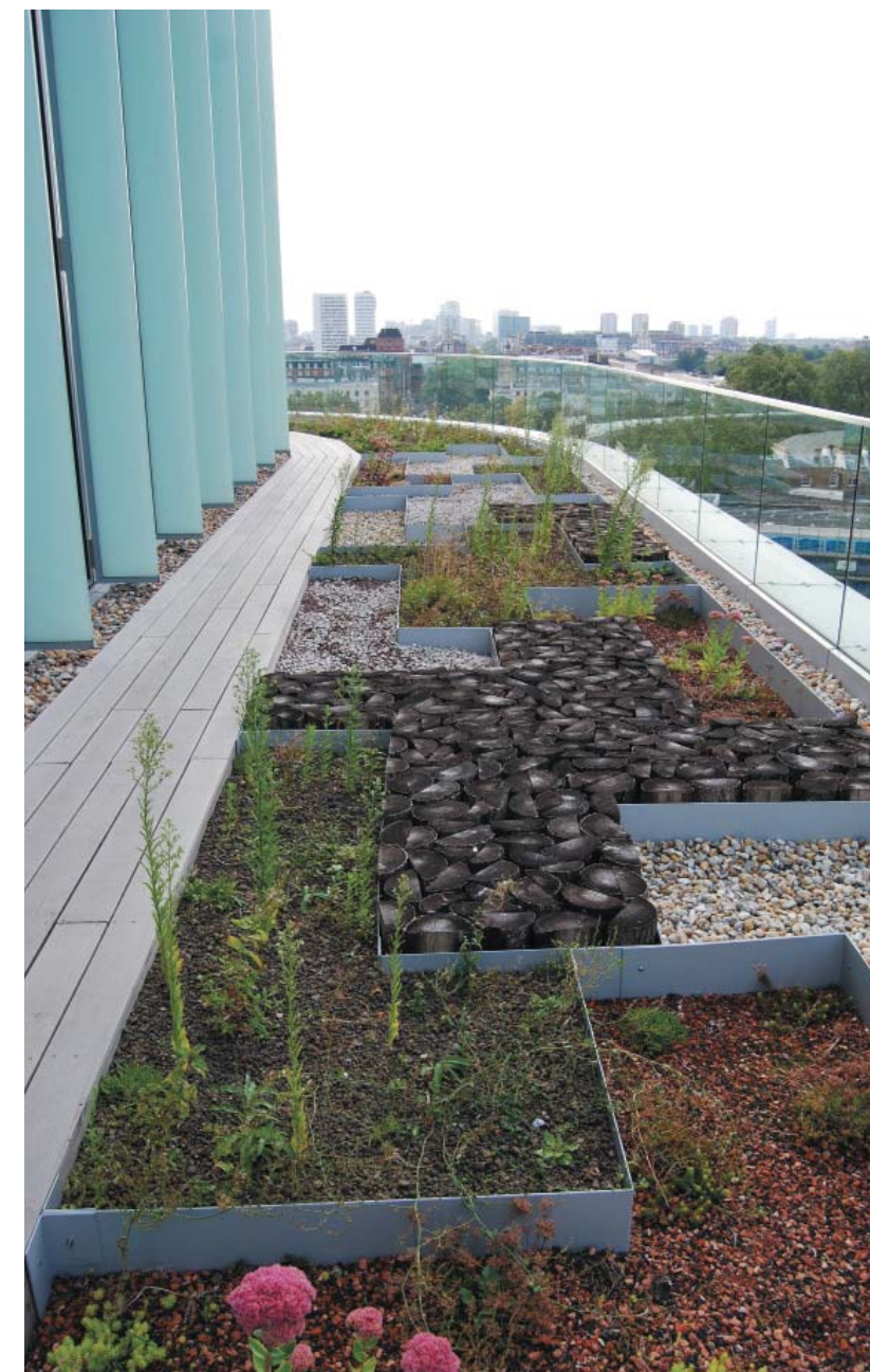
Figure 24.37: Example of a brown roof showing a 'tray system'
