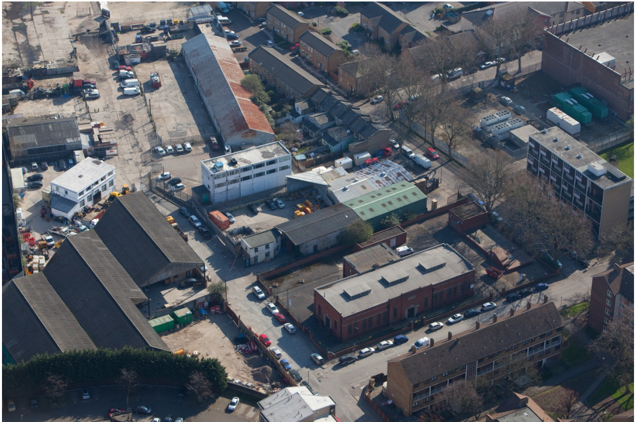
Figure U.1 Aerial photograph of Earl Pumping Station
