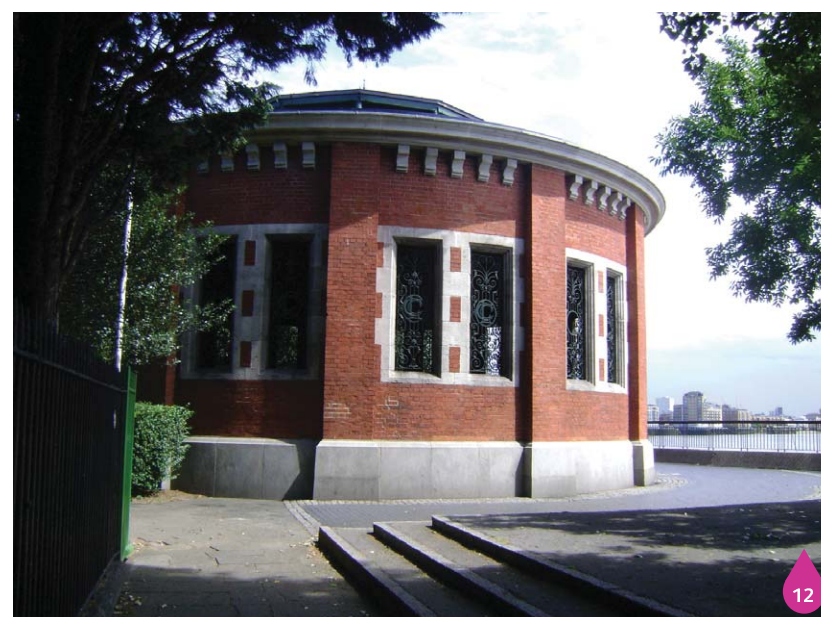
Figure 23.15: View of Rotherhithe ventilation shaft
