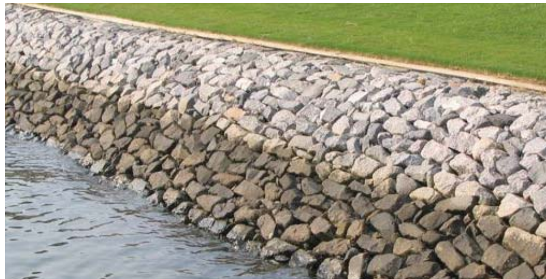
Figure 23.44: Example of 'rip rap scour protection'
