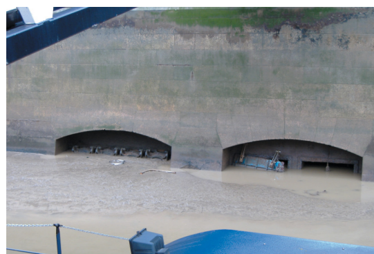
Figure 19.56: Existing Regent Street CSO (right) and abandoned Whitehall Place CSO (left)
