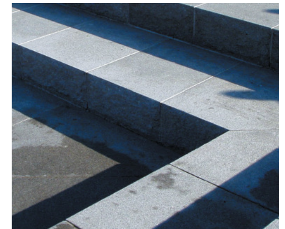
Figure 19.77: Example of paving
