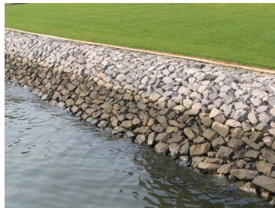
Figure 19.55: Example of 'rip rap' wall
