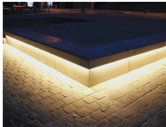
Figure 19.68: Example of landscape lighting
