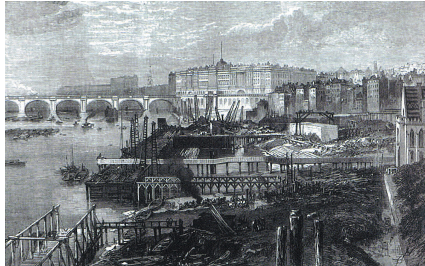
Figure 19.22: Historic drawing of Victoria Embankment under construction © Mary Evans Picture Library
