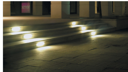
Figure 19.67: Recessed step Luminaires - directed light
