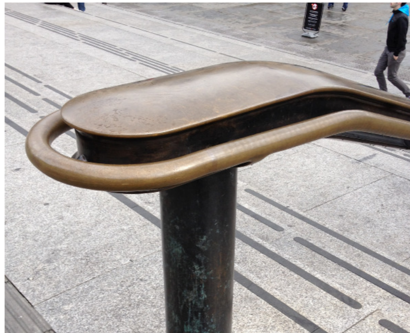
Figure 19.72: Example of brass handrail
