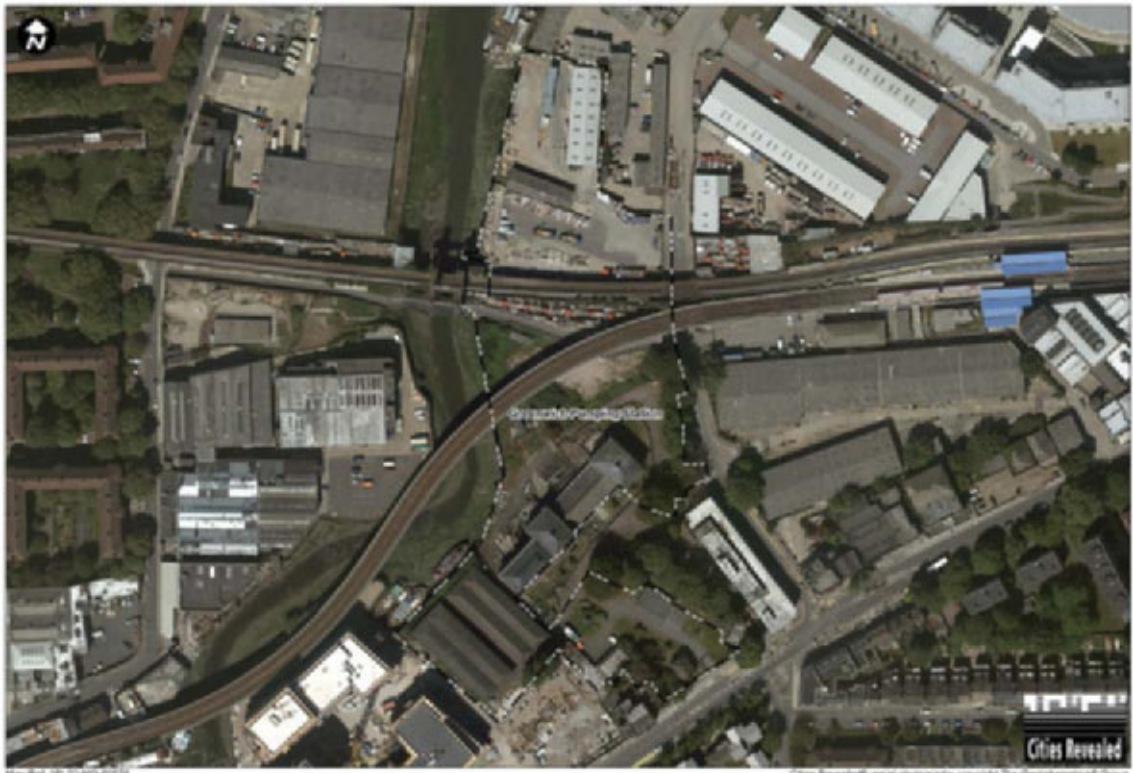
Vol 24 Plate 2.1.1 Greenwich Pumping Station site – aerial photograph
