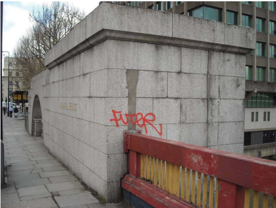
Vol 3 Plate E.56 North-east abutment walls viewed from deck level
