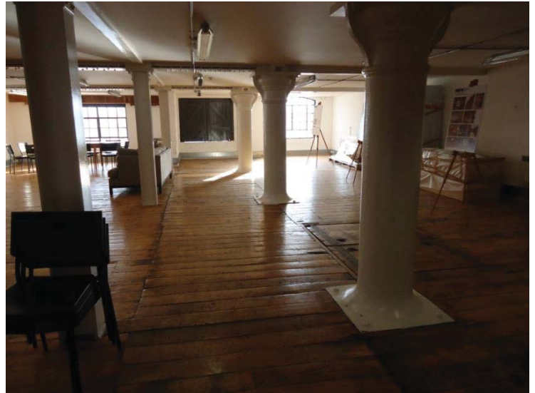
Ground floor columns and timber floor in 'D' Warehouse
