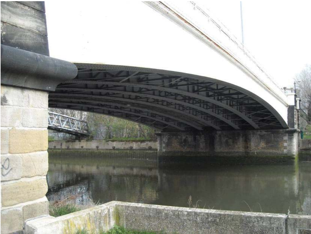
Vol 3 Plate E.131 East span viewed from south
