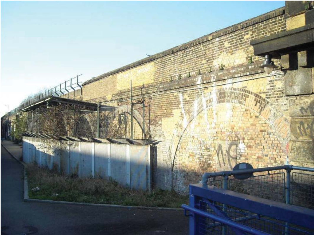
Vol 3 Plate E.120 West viaduct (south side) viewed from footbridge
