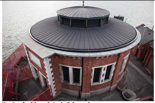
Caption 2 – View of air shaft from above
