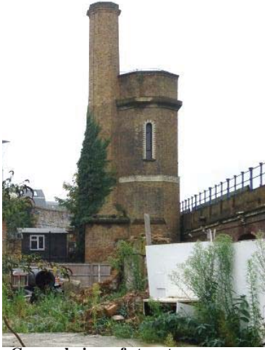
Caption 1 - General view of structure
