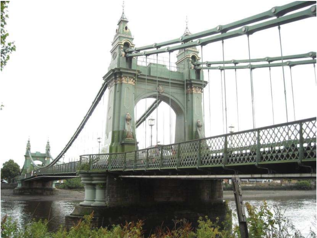
Vol 3 Plate E.2 Hammersmith Bridge viewed from the south-west
