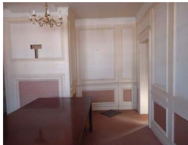
Principal room with panelling and blocked in fireplace
