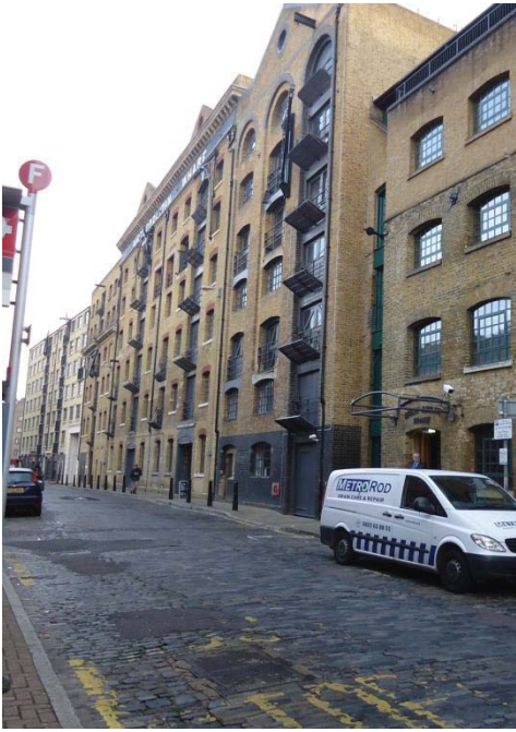
General view of Metropolitan Wharf, with 'A' Warehouse to the far left
