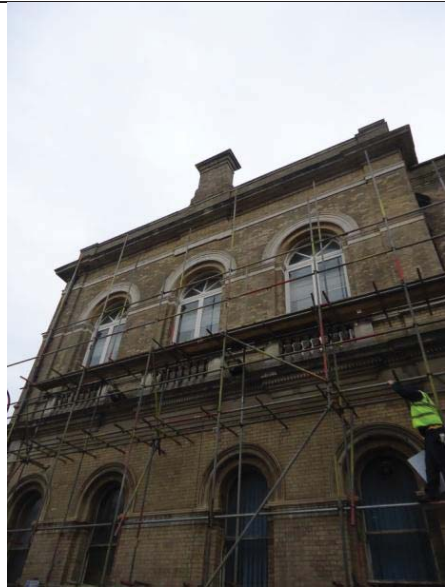
Side (eastern) elevation showing scaffolding
