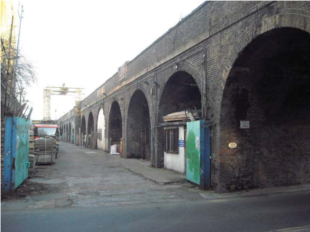
Vol 3 Plate E.121 West viaduct (north side) viewed from Creekside
