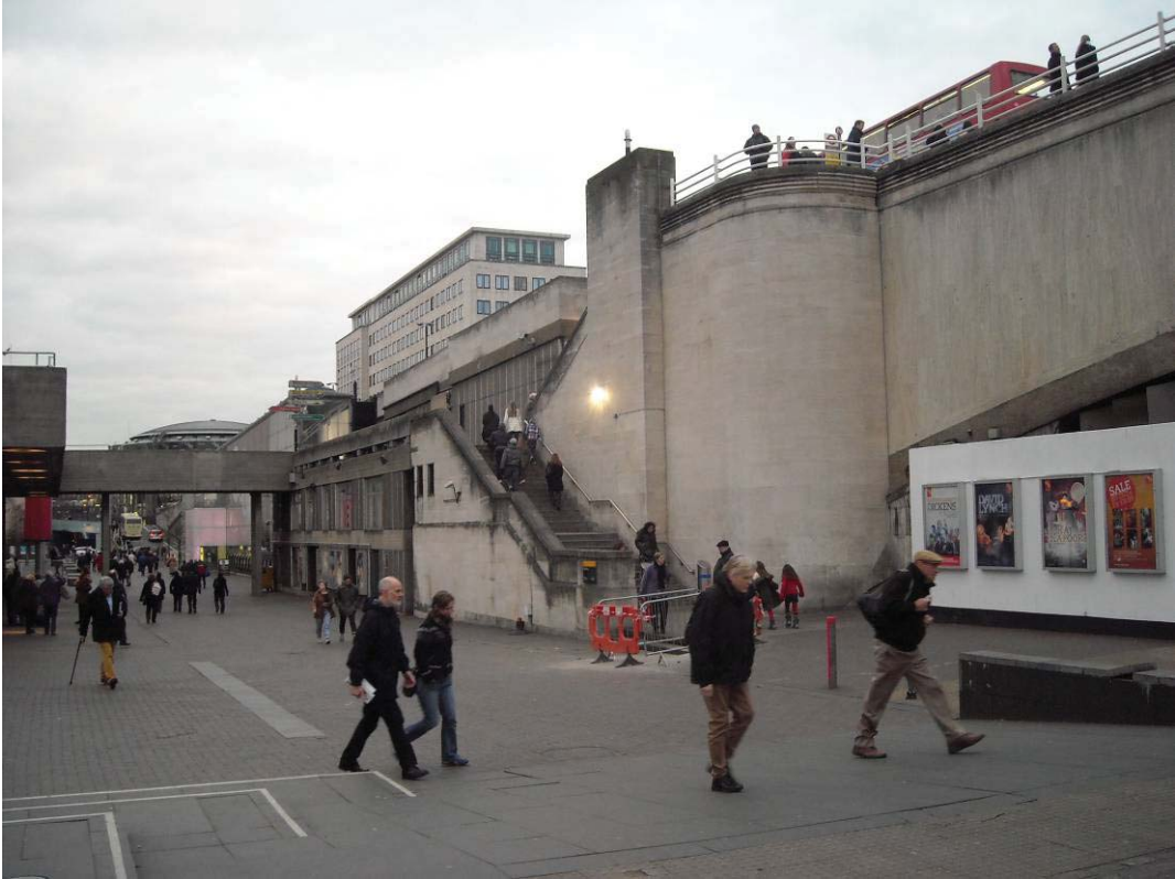
Vol 3 Plate E.73 Waterloo Bridge south shore pier with dog leg staircase
