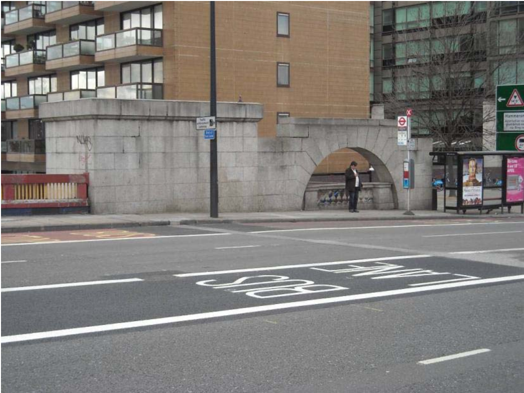
Vol 3 Plate E.55 North-west abutment walls viewed from deck level
