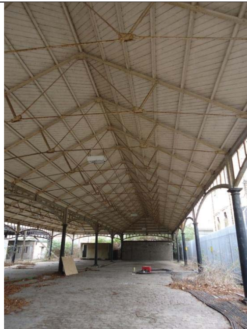
Example of curtilage building on the site, in this case storage sheds with granite sett flooring
