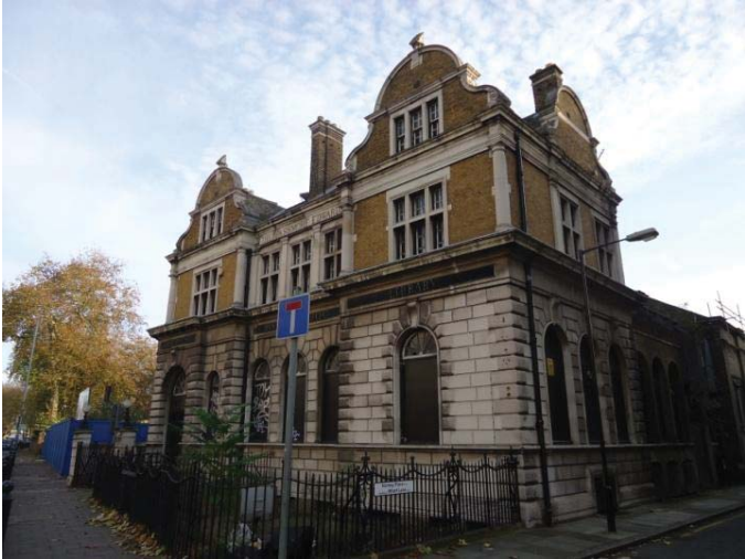
Main (north) elevation
