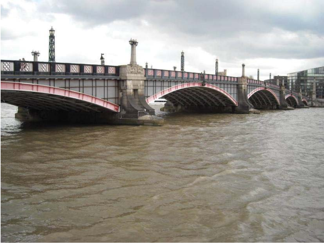
Vol 3 Plate E.62 Lambeth Bridge viewed from the south-west
