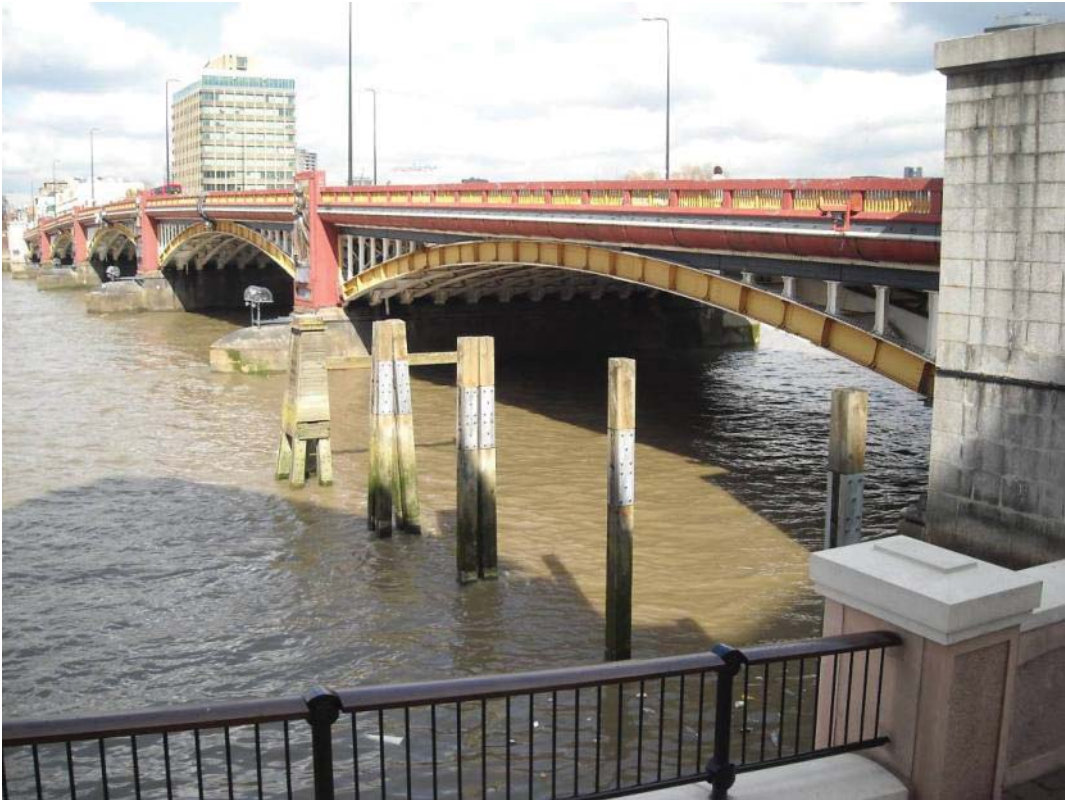
Vol 3 Plate E.47 Bridge viewed from south-west
