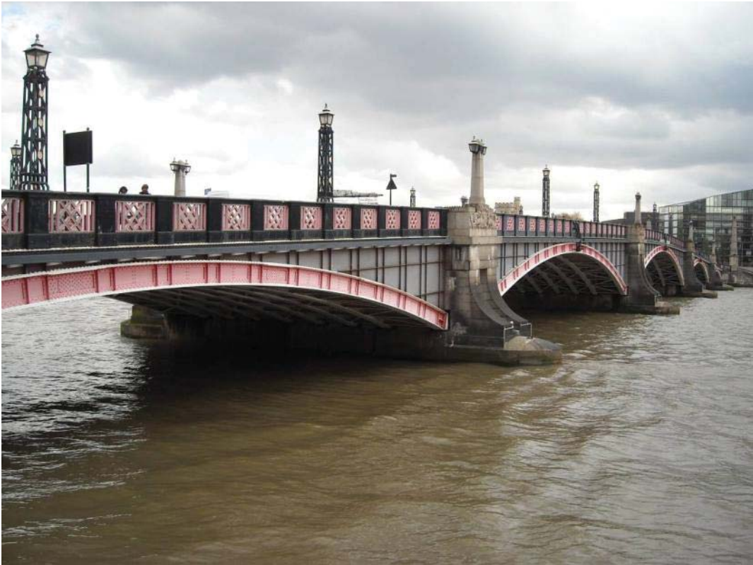
Vol 3 Plate E.63 Lambeth Bridge viewed from the south-west
