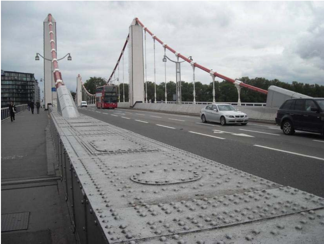
Vol 3 Plate E.34 Chelsea Bridge looking south
