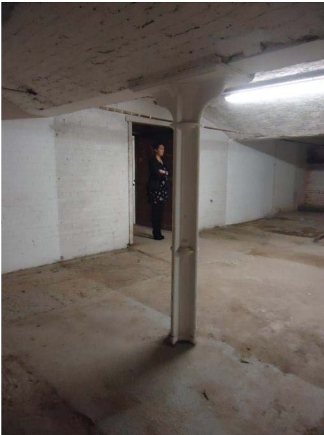
Typical basement view
