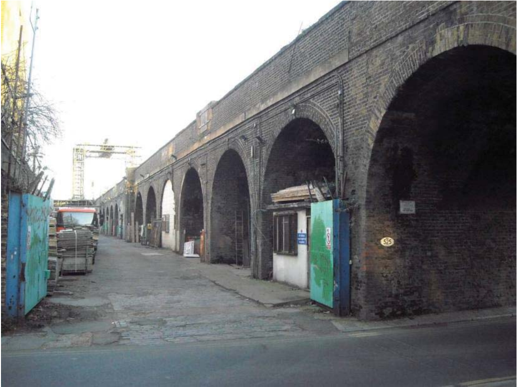
Vol 3 Plate E.107 Railway Bridge over Creekside viewed from north-west
