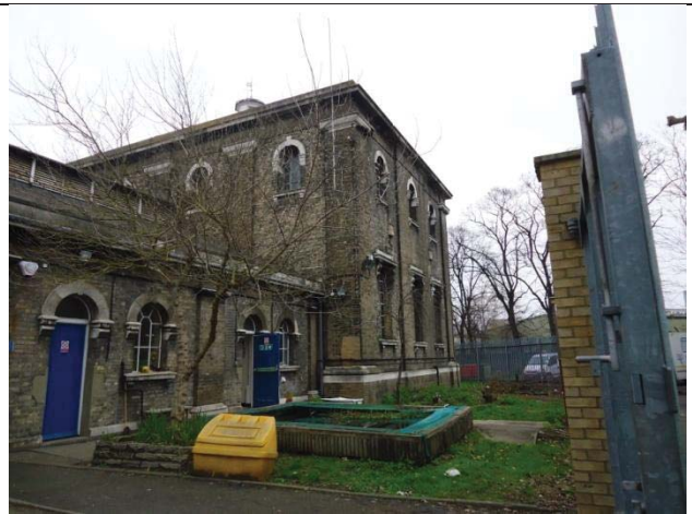
South eastern elevation of the east beam engine house, with linking boiler house to left
