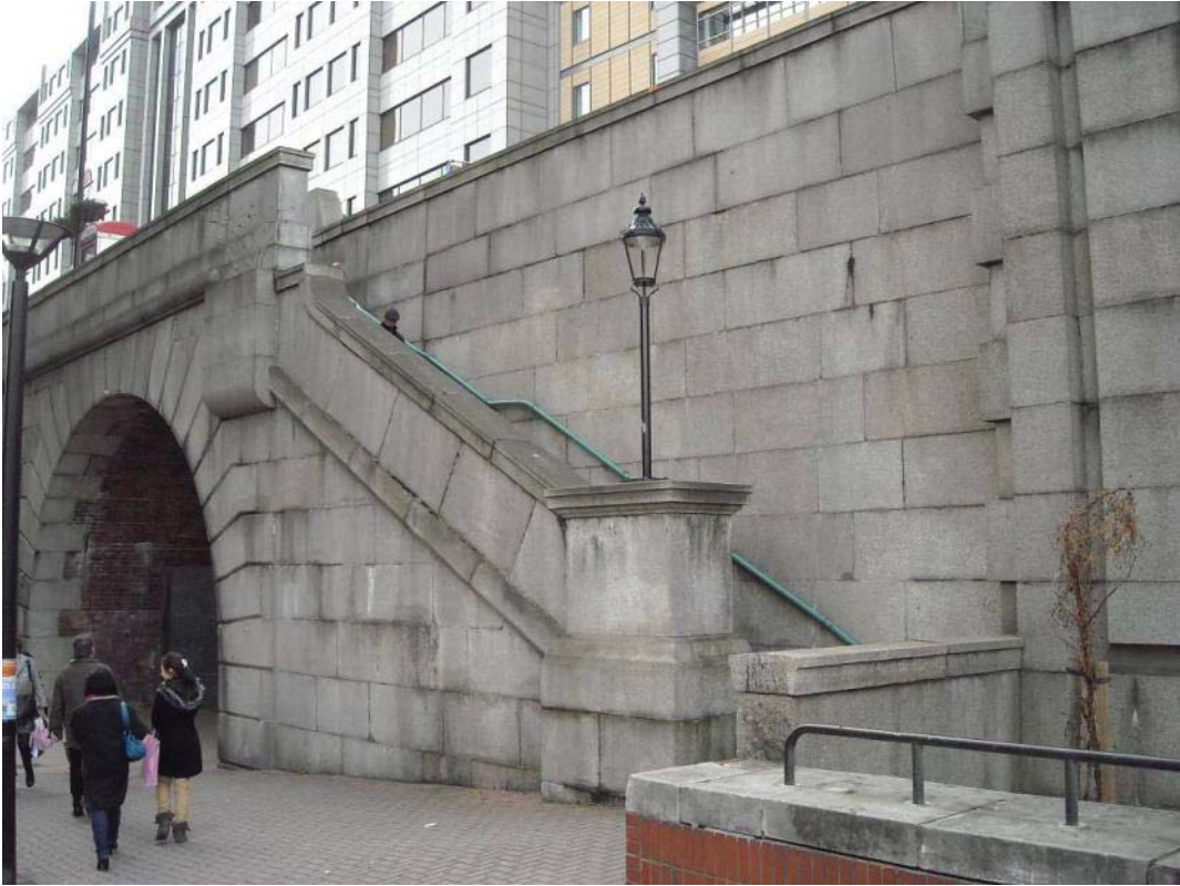
Vol 3 Plate E.87 South abutment vaulted access
