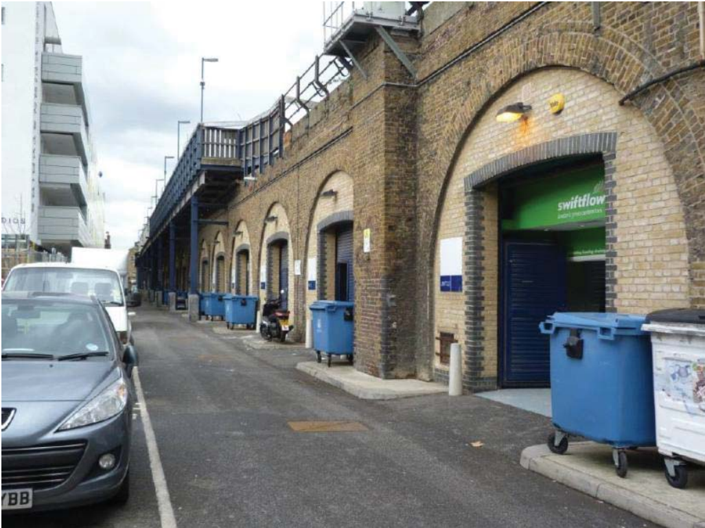
Vol 3 Plate E.101 Mechanics Path Viaduct viewed from south-east
