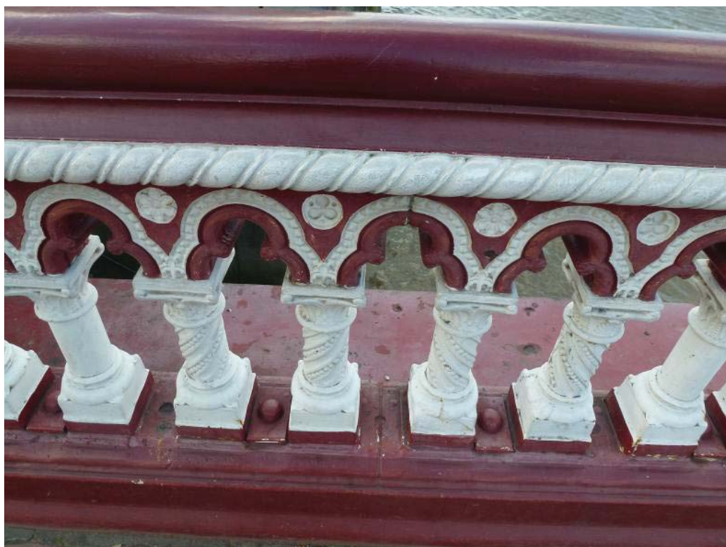
Vol 3 Plate E.79 Detail of the cast iron balustrade
