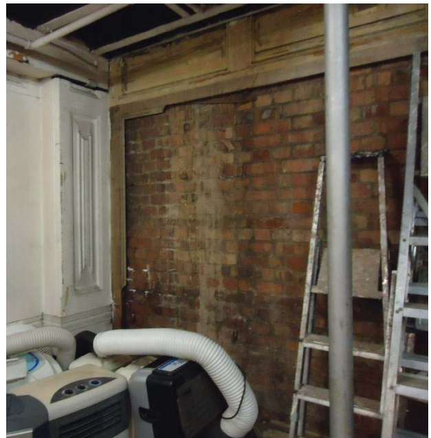
Example of timber panelling with scroll detail in basement
