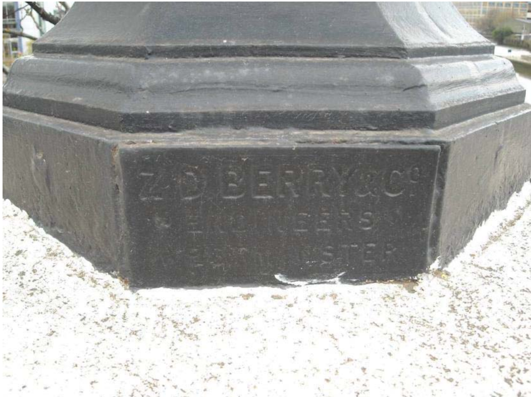
Vol 3 Plate E.136 Detail of gas lamp base displaying manufacturer's name
