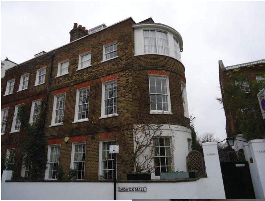
Exterior from river (south)
