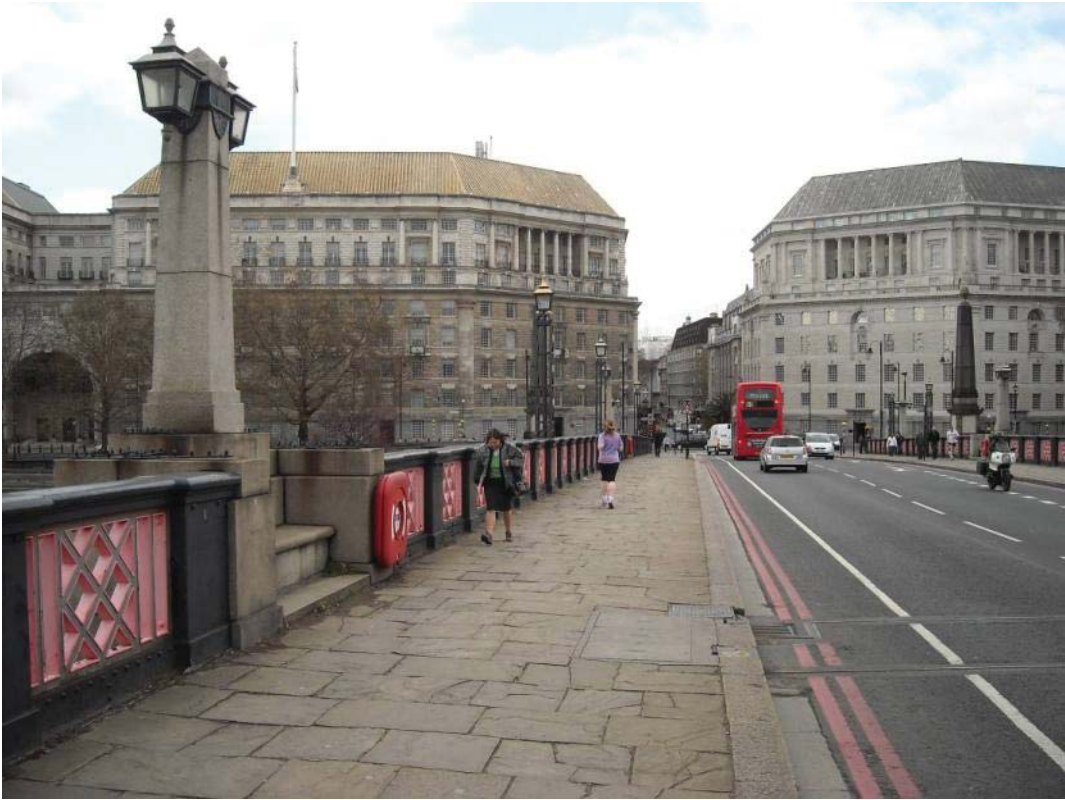
Vol 3 Plate E.64 Looking west at deck level towards Norwest and Thames House
