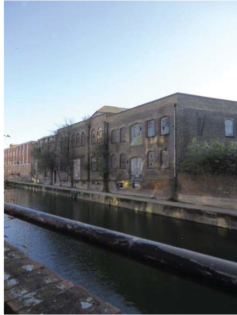
Rear elevation to Limehouse Cut
