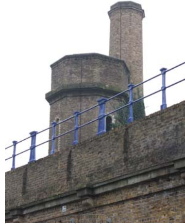
Caption 2 – Upper section of tower and chimney
