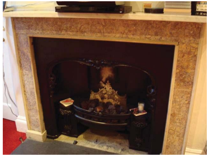
Example of retained fireplace
