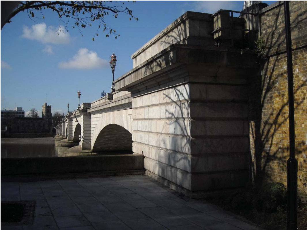
Vol 3 Plate E.9 Putney Bridge viewed from the north-east
