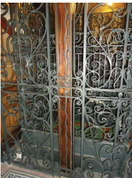
Filigree wrought iron lift casing
