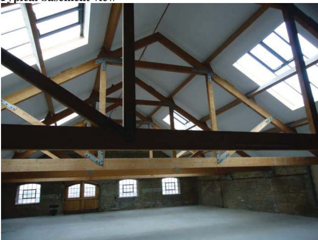
Typical roof truss throughout 'B and C' Warehouses
