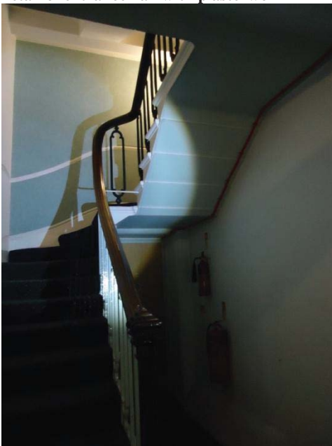
Secondary cantilevered stair
