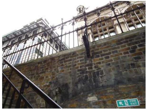
External railings to lightwells
