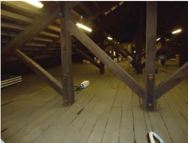
Truss in roof space
