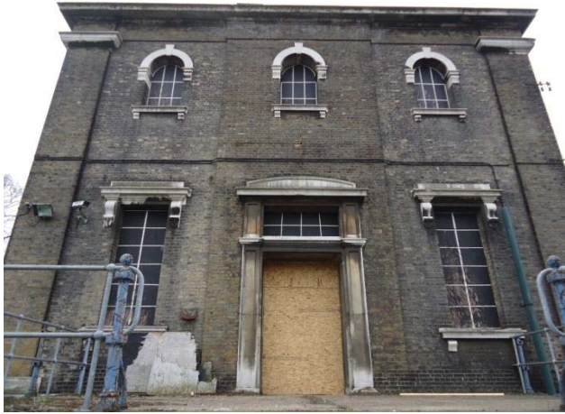
North-eastern elevation of the east beam engine house
