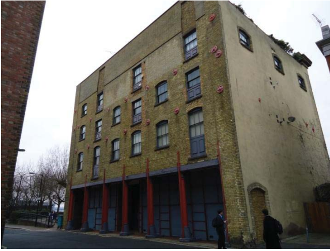
Road (south) elevation and east elevation
