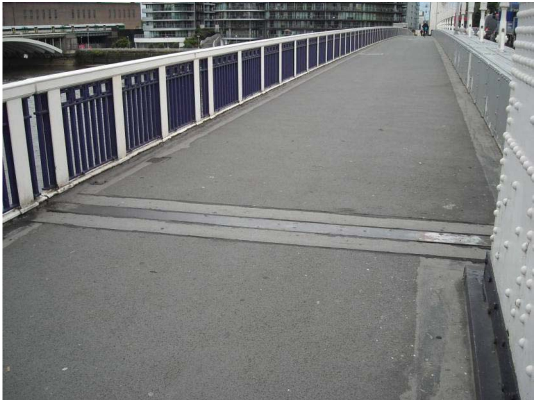
Vol 3 Plate E.35 Chelsea Bridge looking south
