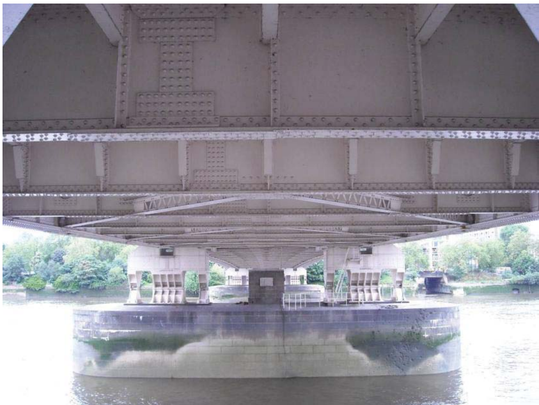
Vol 3 Plate E.36 Underside of bridge deck viewed from south
