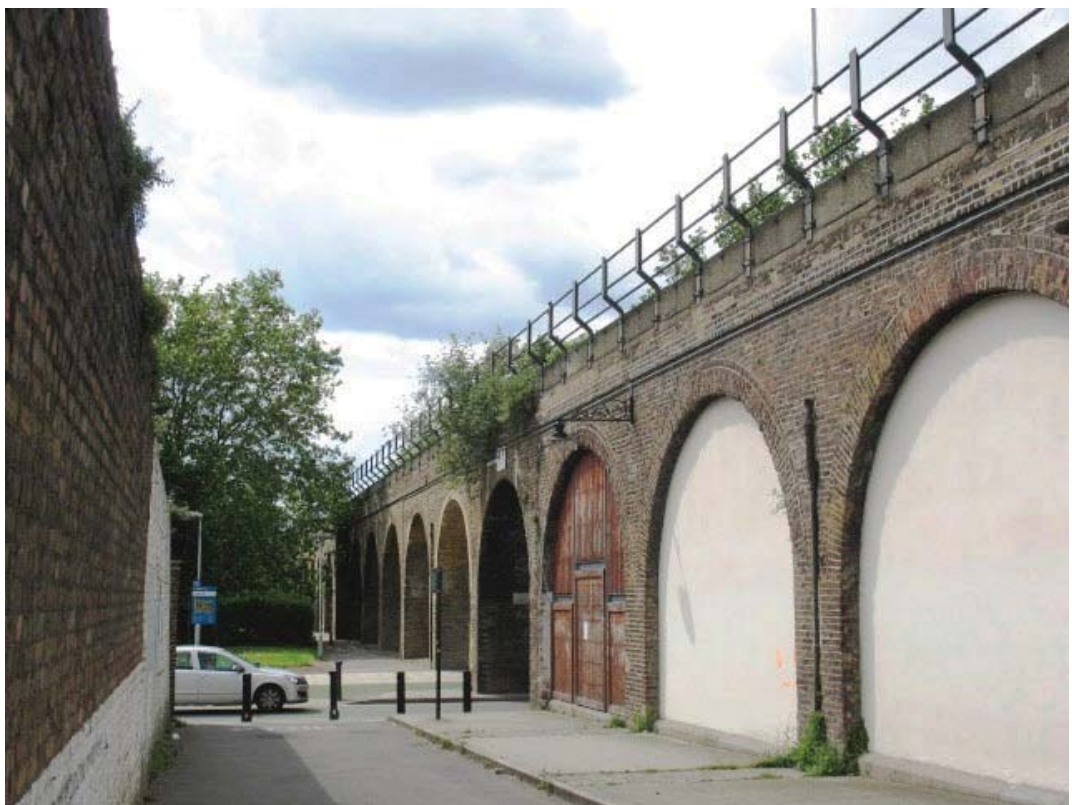
Vol 3 Plate E.111 Sun Wharf Viaduct adjoining Creekside
