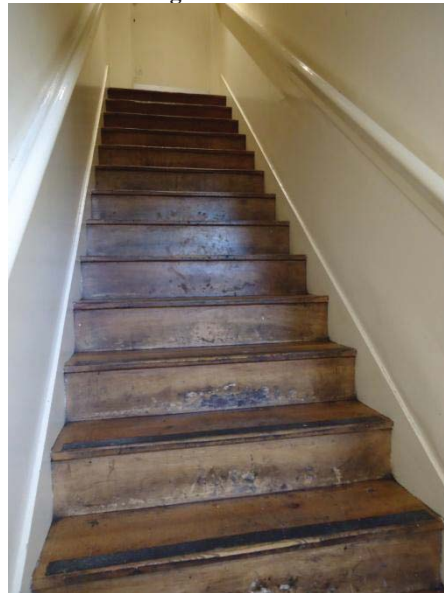
Original timber stair
