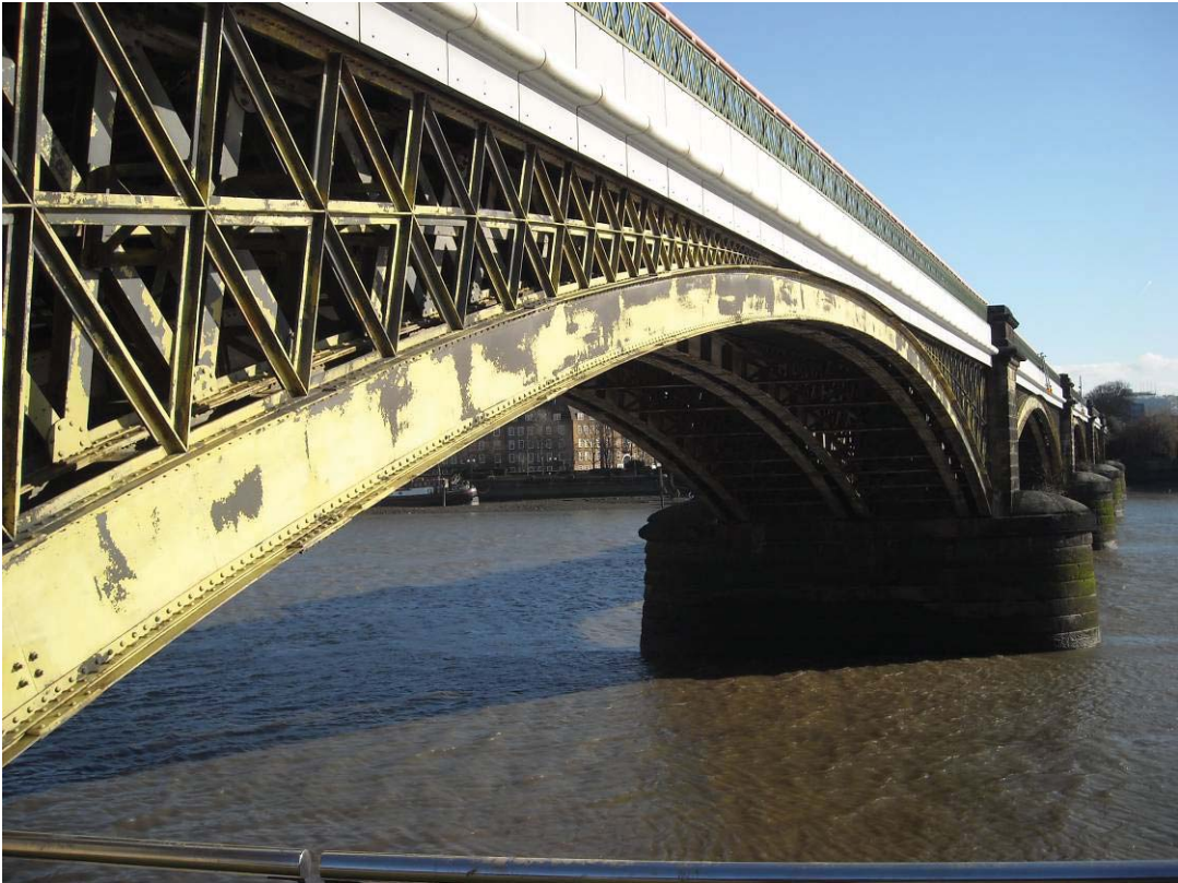
Vol 3 Plate E.41 Bridge viewed from west
