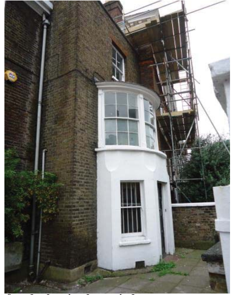
Front façade showing bow window
