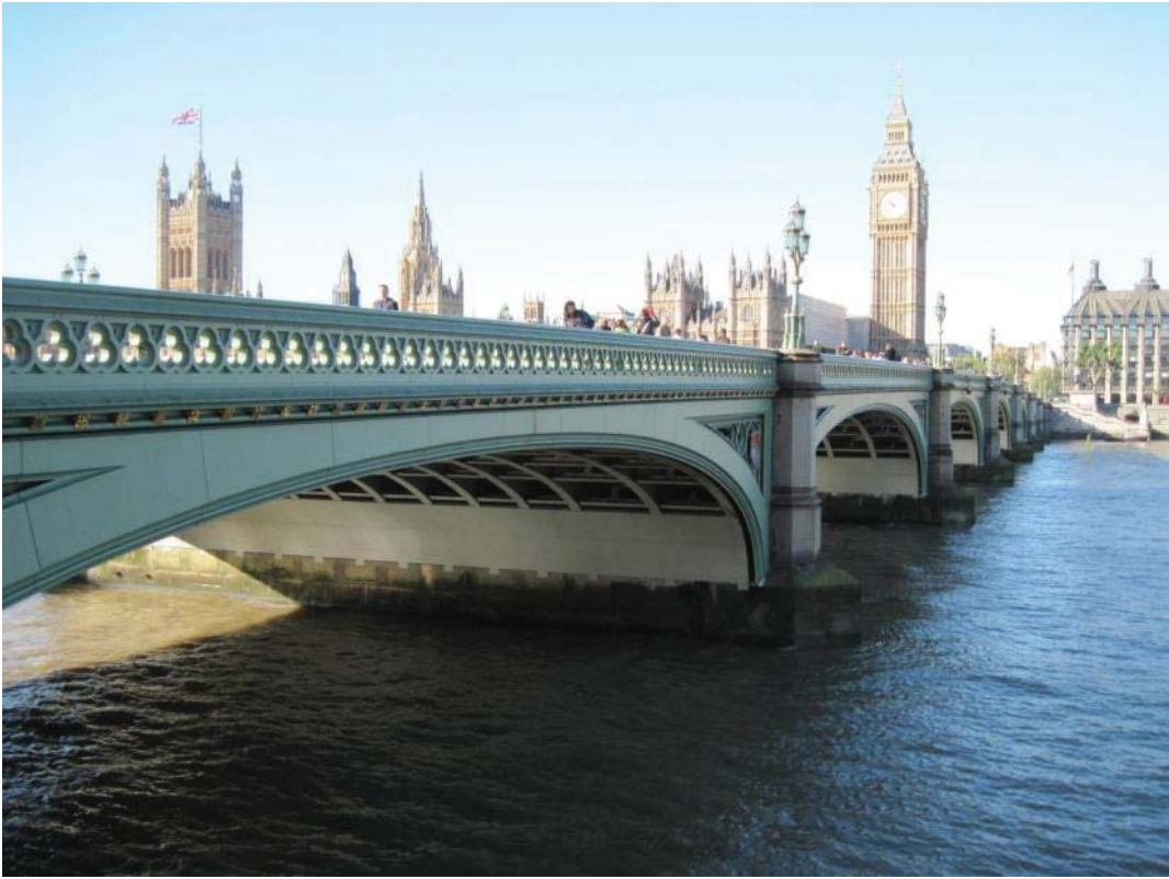
Vol 3 Plate E.69 Bridge viewed from north-east
