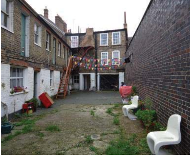
Rear elevation with workers cottages to the left
