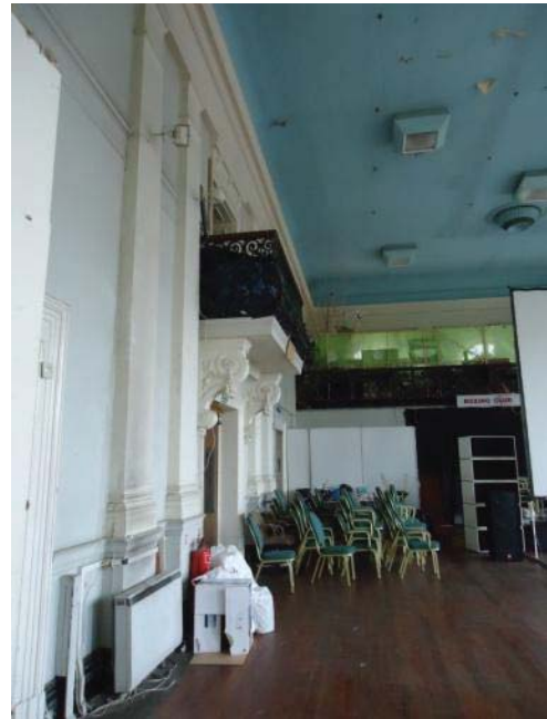
View of the main hall, showing bombe balconette and decorative plasterwork
