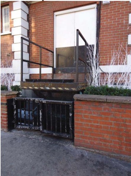
Roadside elevation with lift
