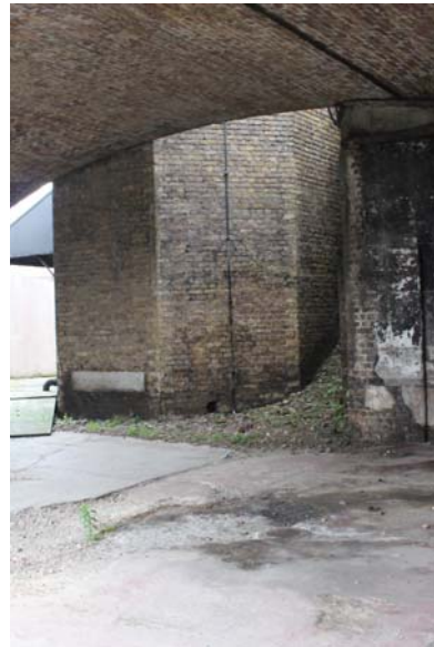
Caption 4 – Base of tower structure
