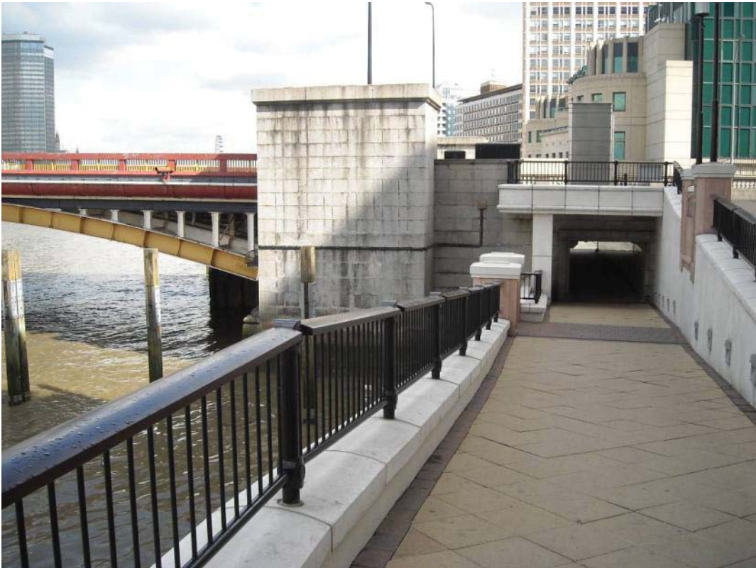
Vol 3 Plate E.48 South abutment and pedestrian underpass viewed from south-west
