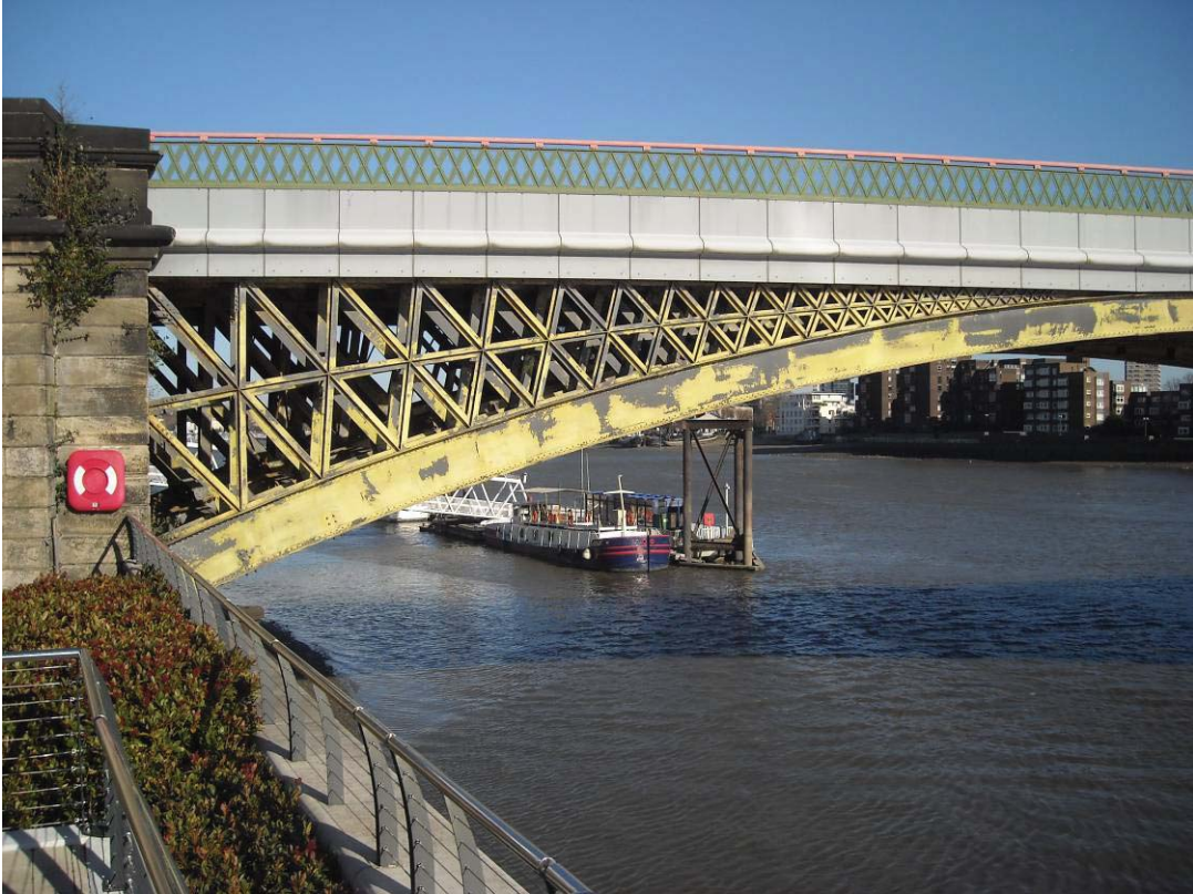
Vol 3 Plate E.44 West abutment viewed from south
