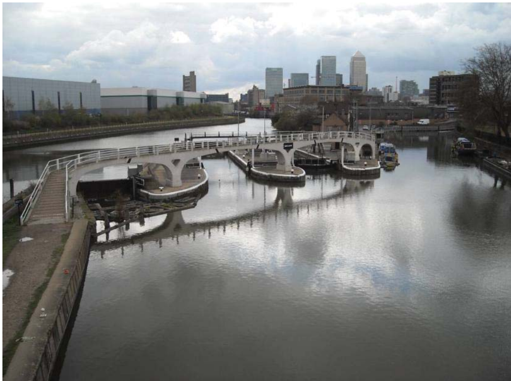
Vol 3 Plate E.137 View of Bow Locks from Twelvvetrees Crescent Bridge
