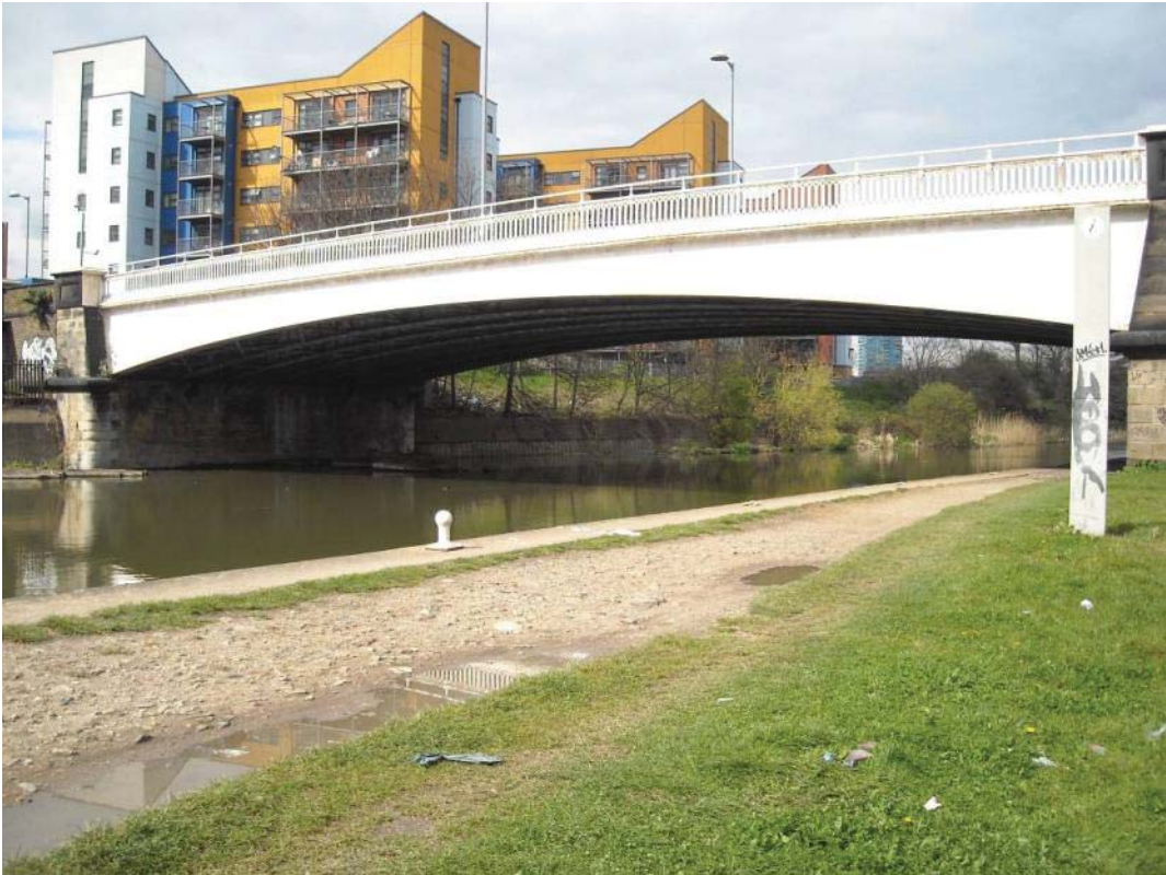
Vol 3 Plate E.130 West span viewed from south
