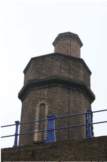
Caption 3 – Upper section of tower and chimney in background
