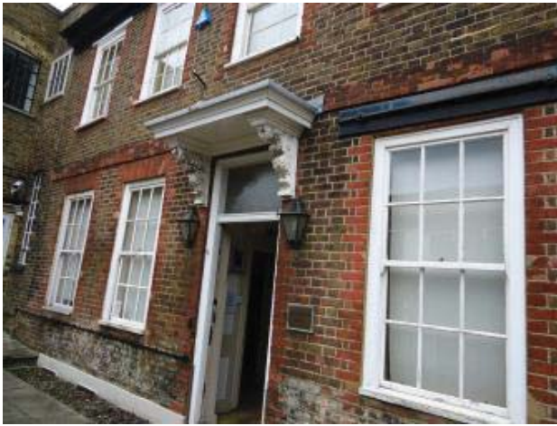
Front (western) façade with timber eaves cornice and hooded doorcase
