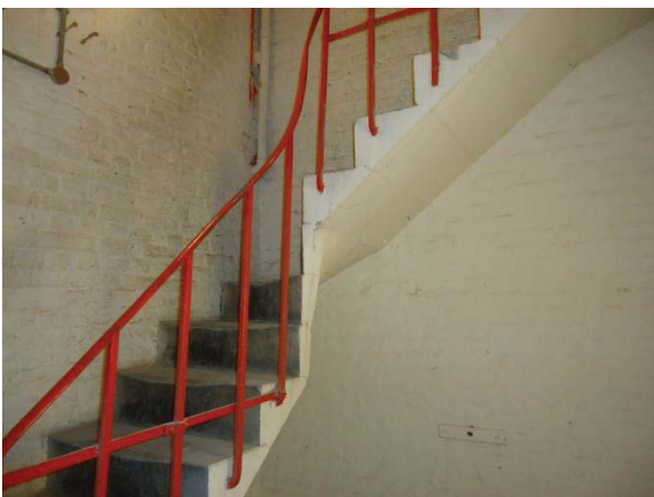
Cantilevered stair between 'A' and 'B' Warehouse
