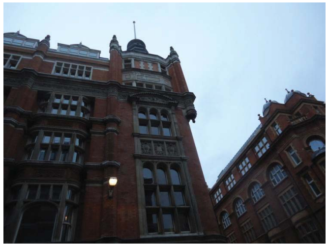
Corner tower from Carmelite Street
