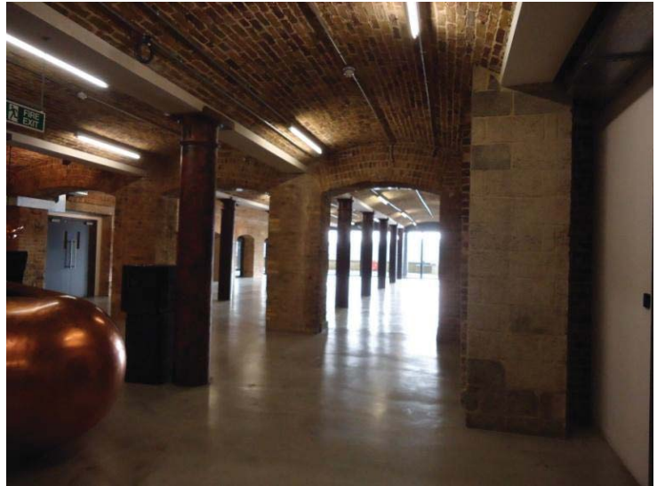
General view of ground floor column layout and structure
