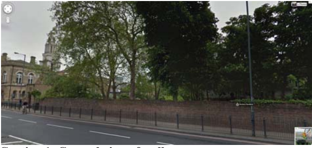
Caption 1: General view of wall
