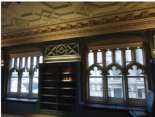
Interior of principal room, showing stone window surrounds and decorative plasterwork
