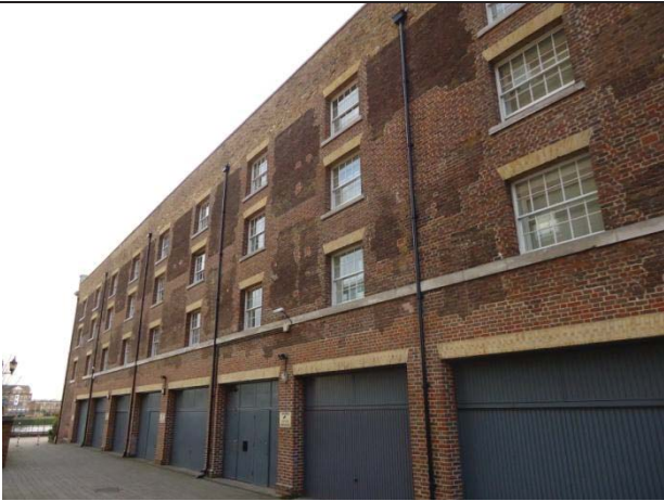
East elevation of eastern building
