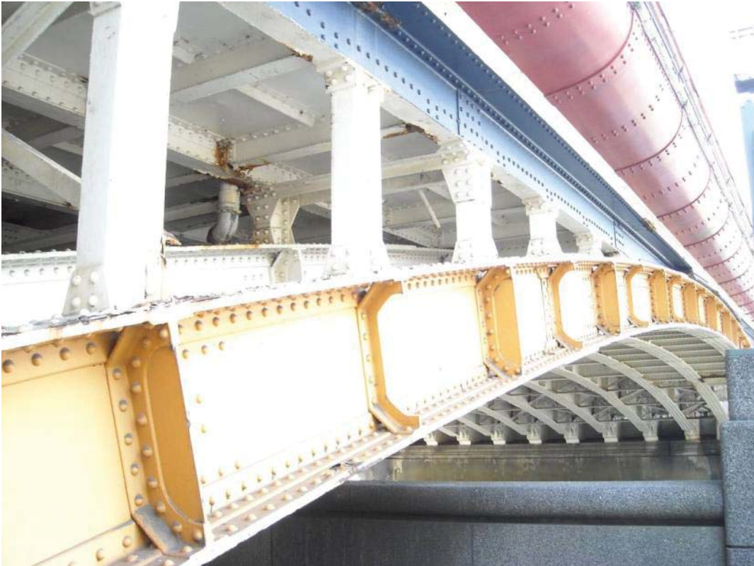
Vol 3 Plate E.51 South most (Lambeth) arch viewed from east
