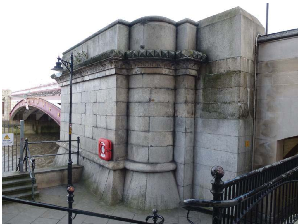
Vol 3 Plate E.80 The southern granite clad abutment
