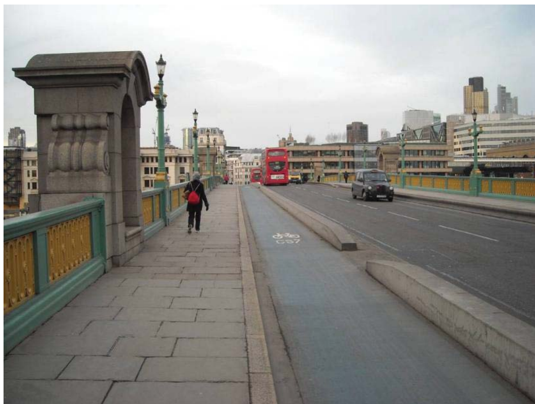
Vol 3 Plate E.88 View looking north along deck
