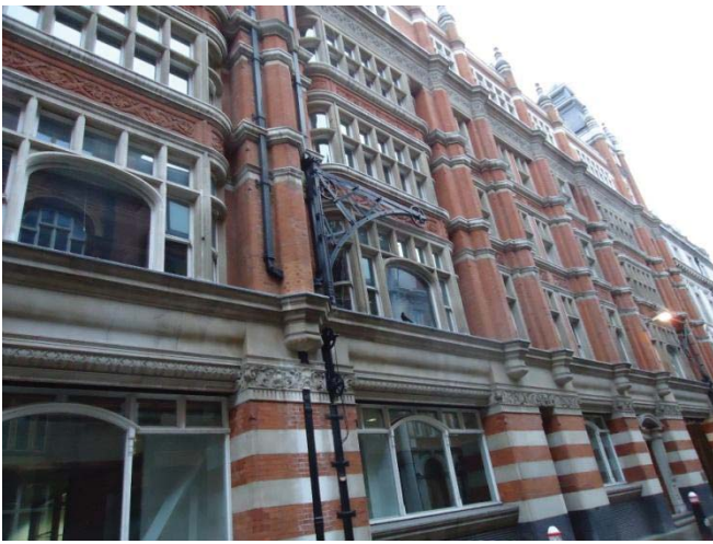
Tallis Street façade
