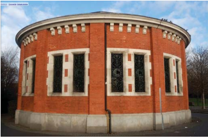
Caption 1 – General view of air shaft
