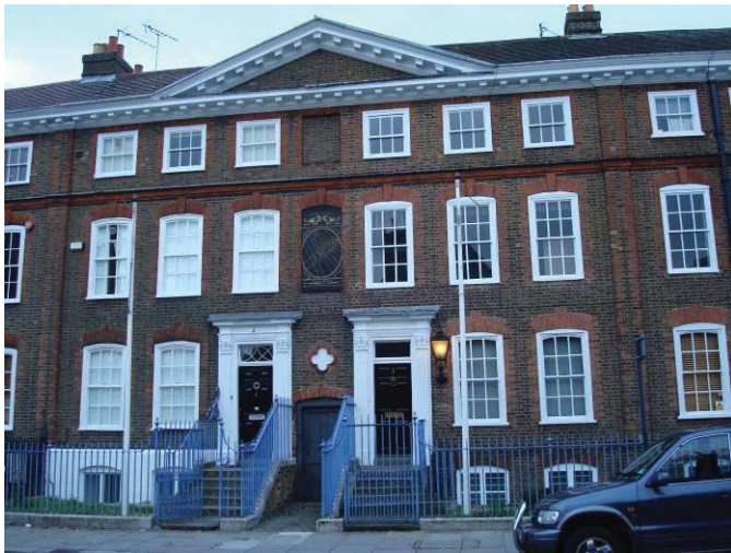
Main façade, from the east
