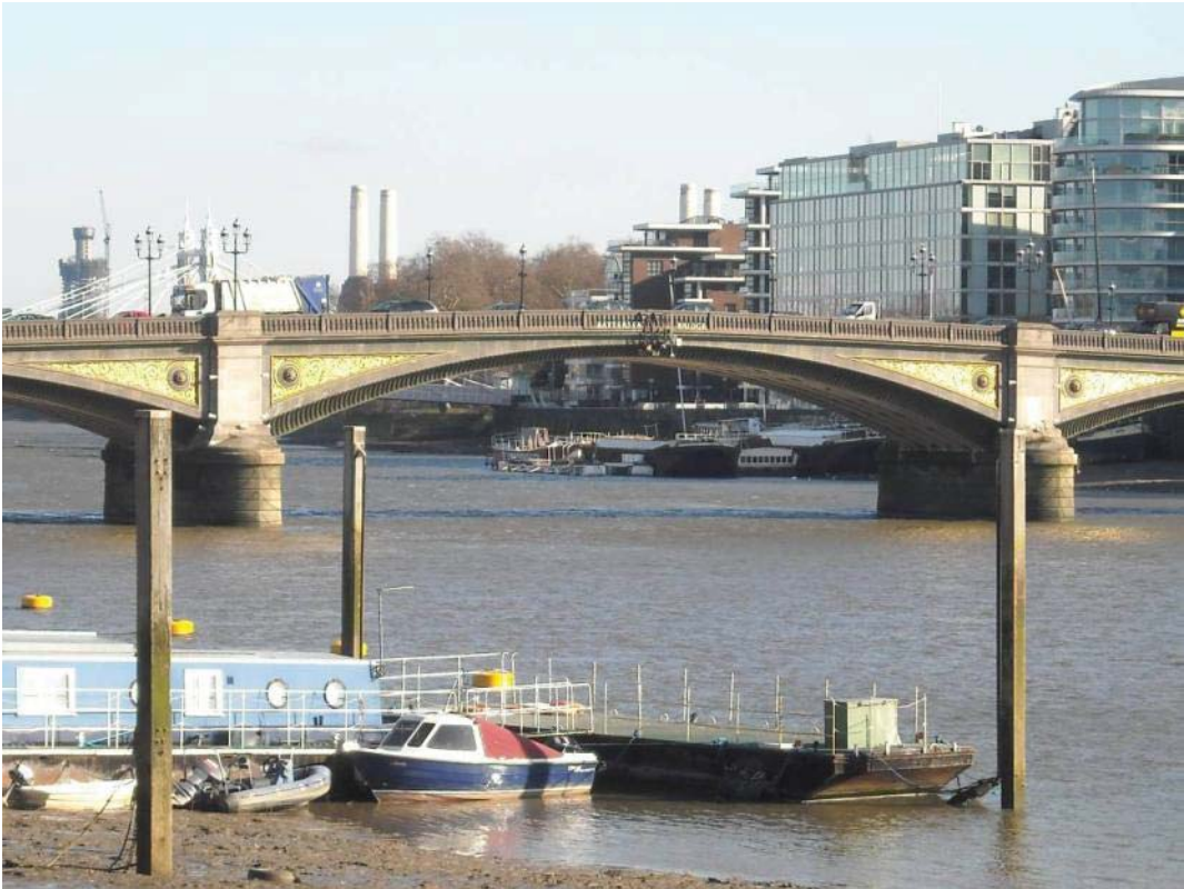
Vol 3 Plate E.18 Bridge viewed from west
