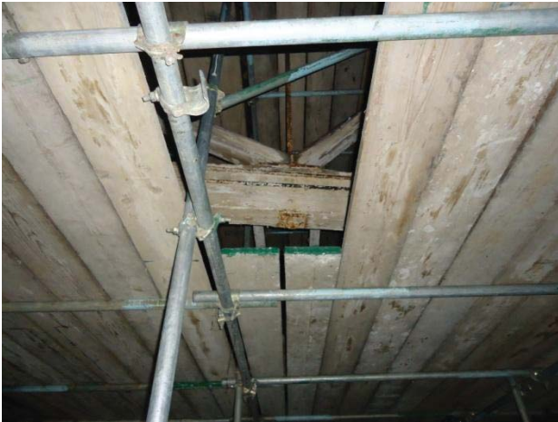
View of queen-rod truss through scaffolding
