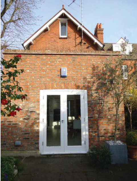
Rear elevation of 60 Bath Road, including recent extension
