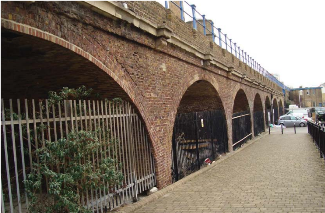
Vol 3 Plate E.126 DLR Viaduct viewed from south-west
