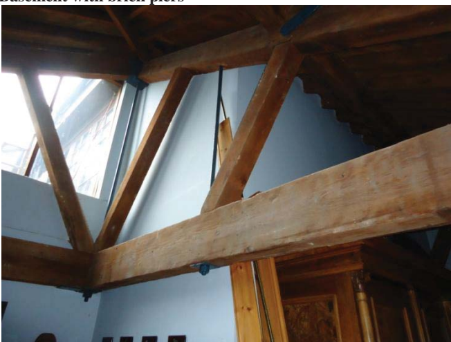
Roof truss visible, top floor
