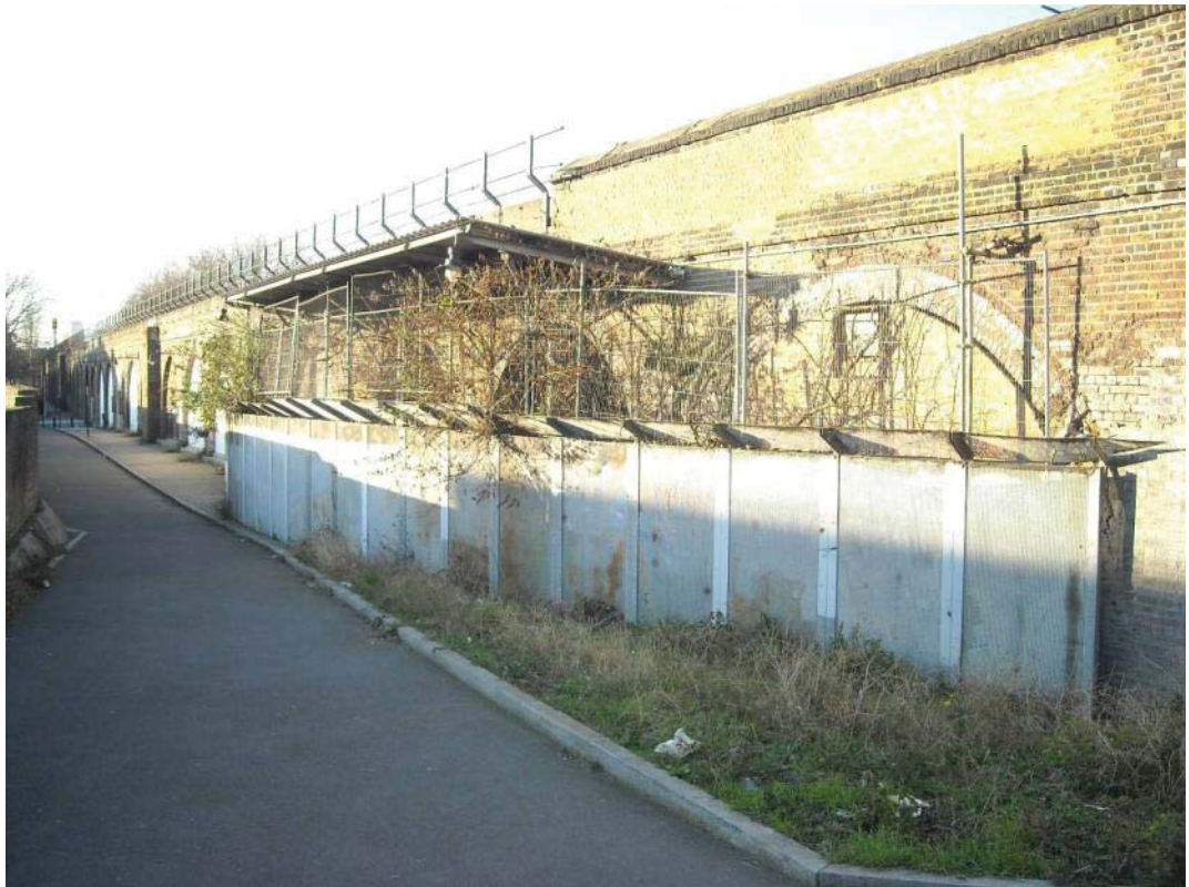
Vol 3 Plate E.110 Sun Wharf Viaduct viewed from south-east
