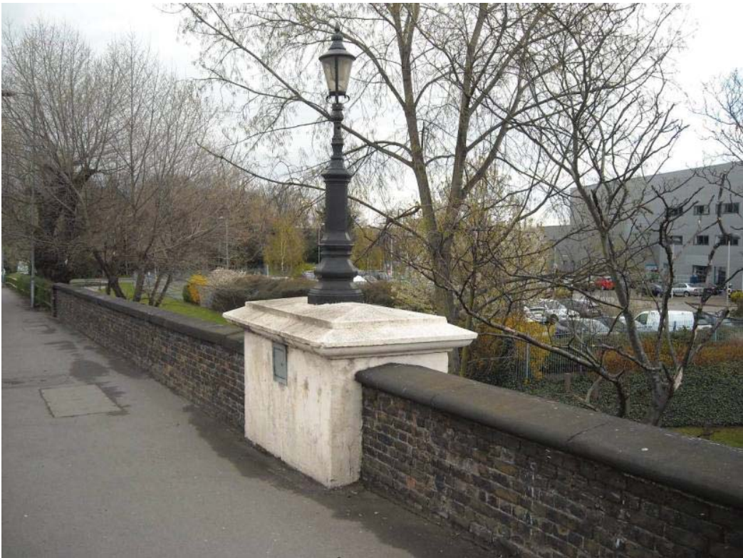
Vol 3 Plate E.135 Historic gas lamp on south-east abutment (one of six)
