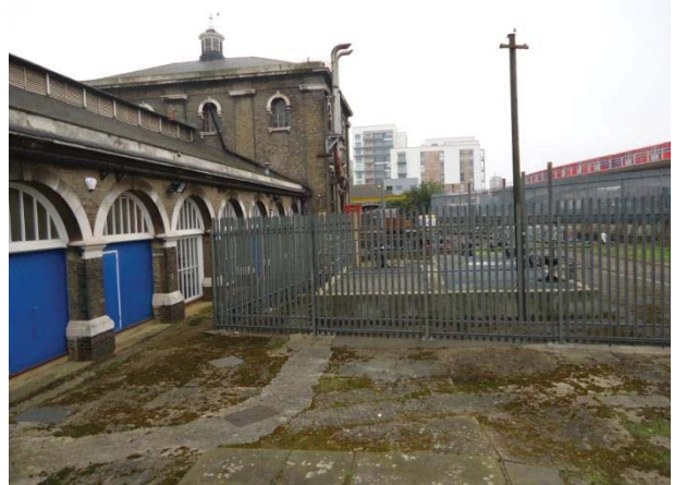
Linking boiler house and west beam engine house beyond
