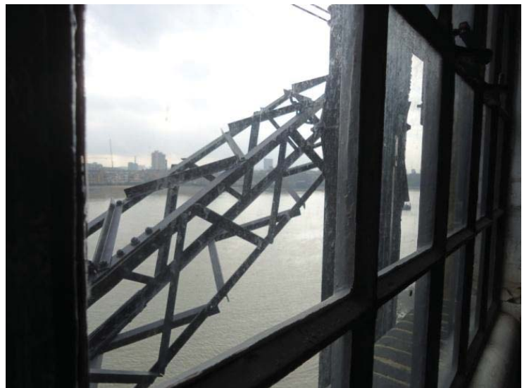
Retained hoist crane to the southern elevation, from inside the building
