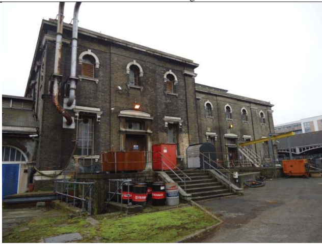
North-western elevation of the west beam engine house
