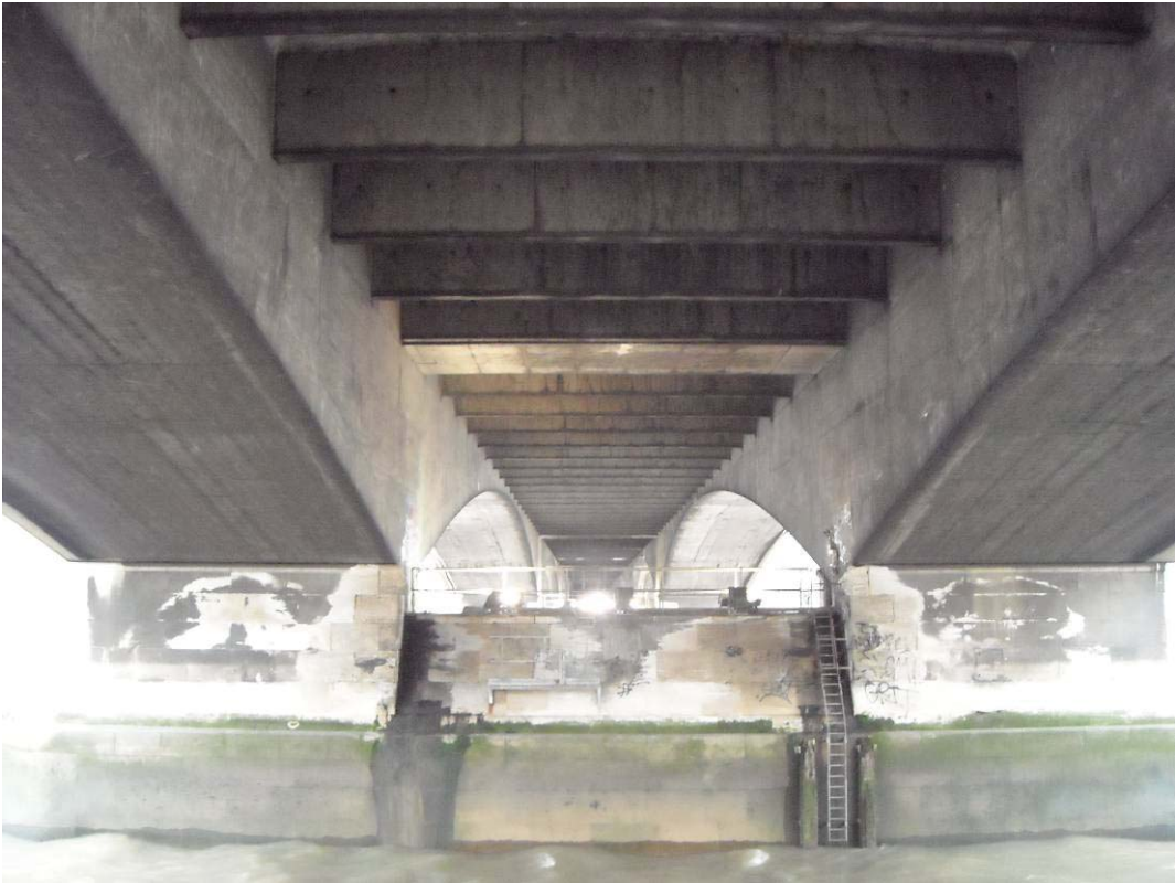
Vol 3 Plate E.76 Underside of bridge viewed from south
