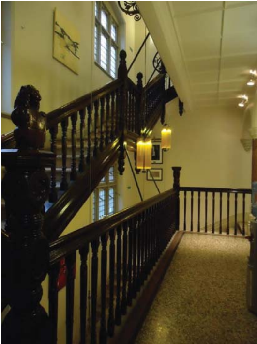
Cantilevered stair showing later supports
