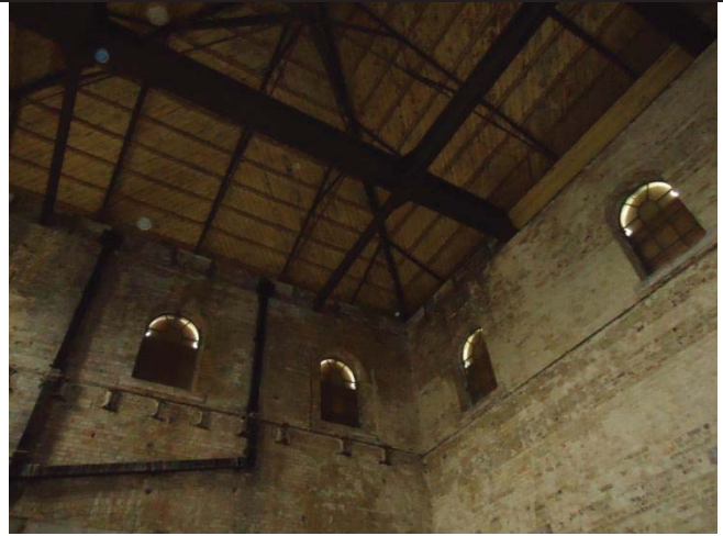
Interior showing roof structure of east beam engine house
