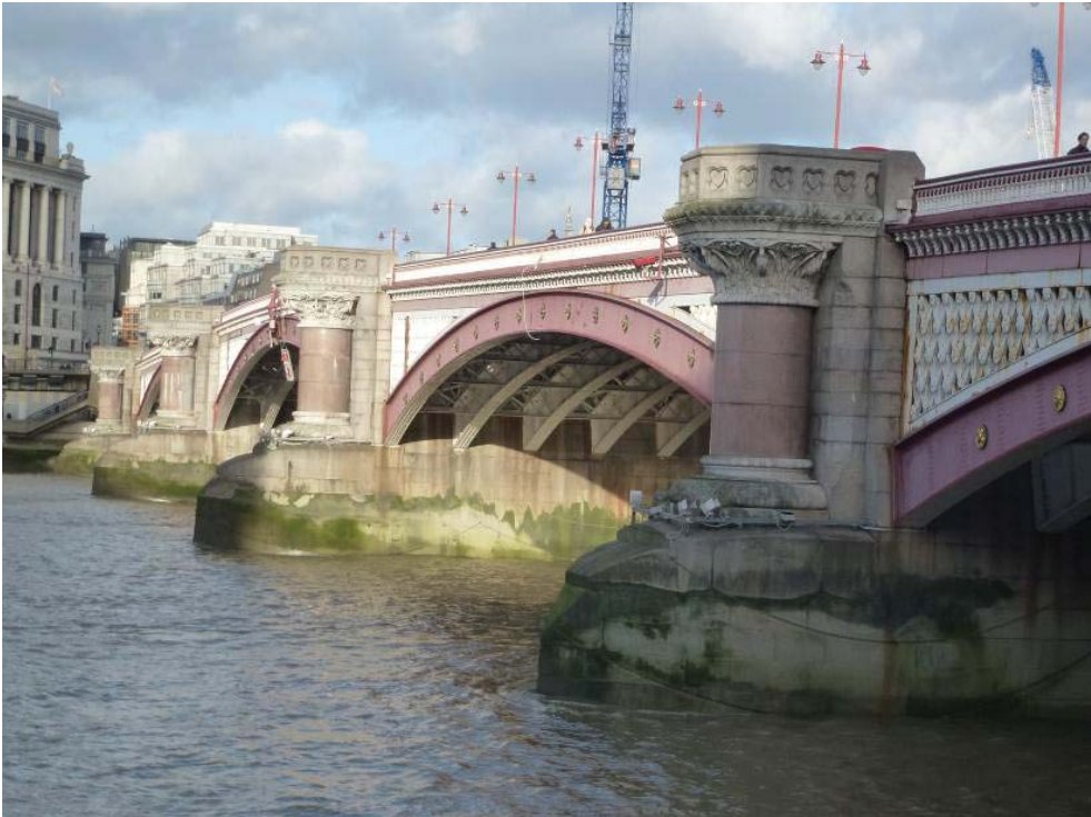
Bridge piers with finely decorated engaged column supporting the seating areas over the pier ends
