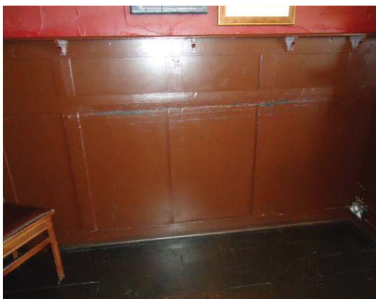
Dado panelling to southern first floor room
