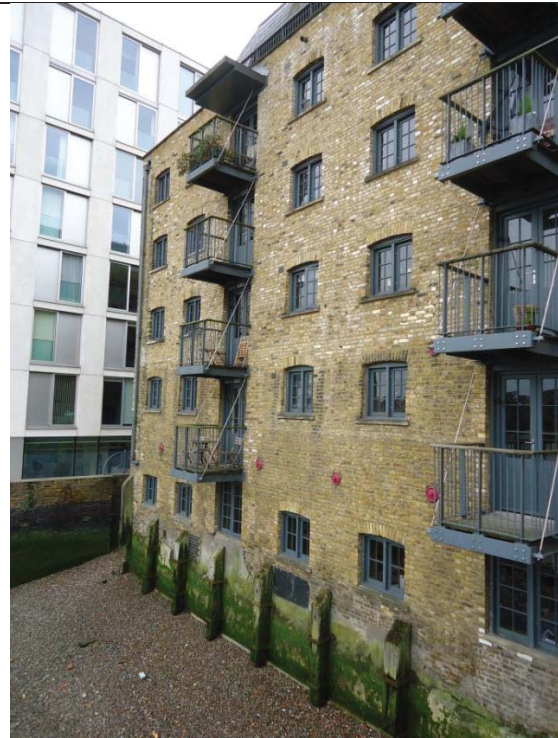
Rear (north) elevation, from the riverside
