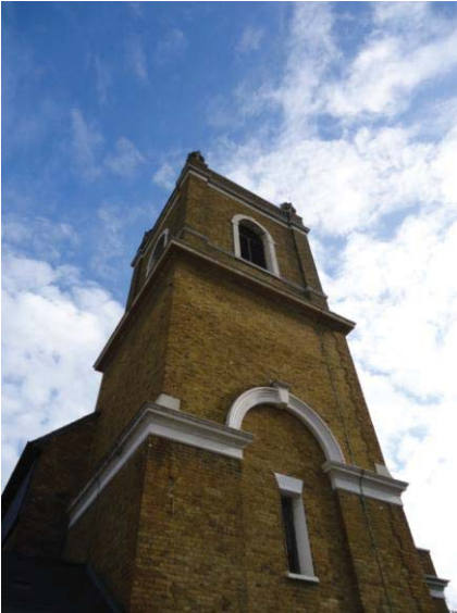
Tower from west
