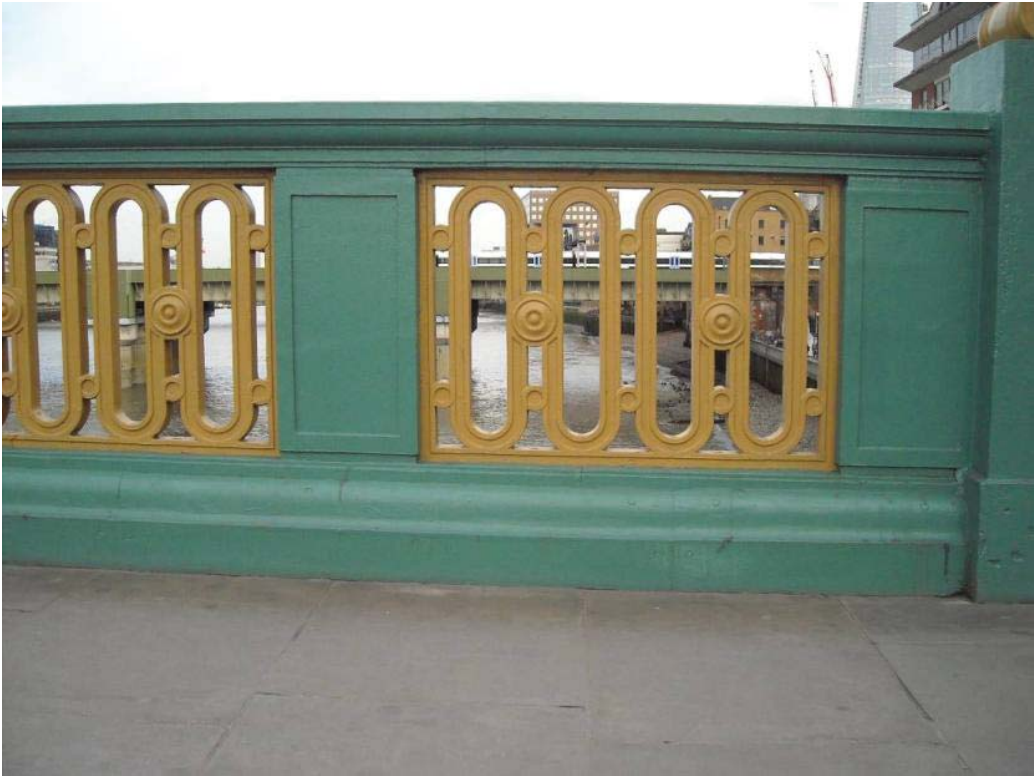
Vol 3 Plate E.90 Detail of cast-iron balustrade
