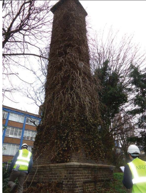
Ivy-covered chimney-vent to the centre of the site
