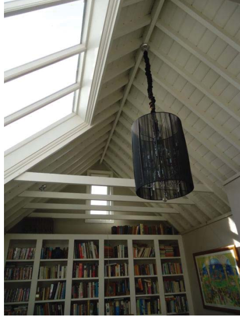
'Studio' room to the first floor, showing modern windows and roof structure
