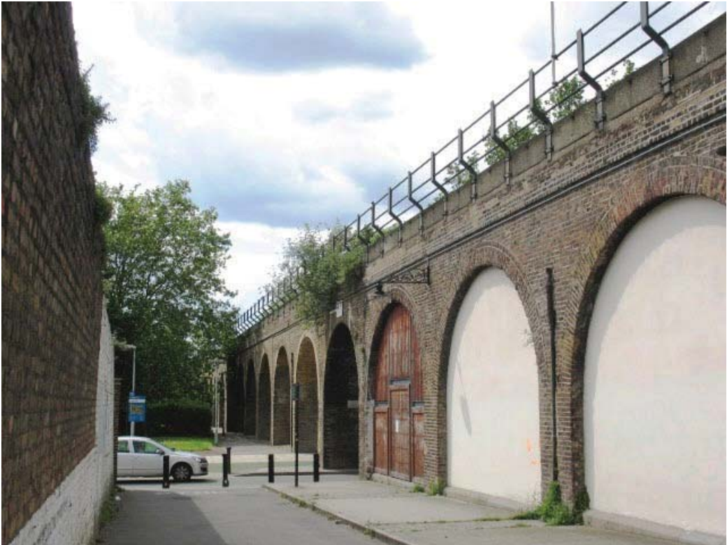
Vol 3 Plate E.108 Railway Bridge over Creekside viewed from south-east
