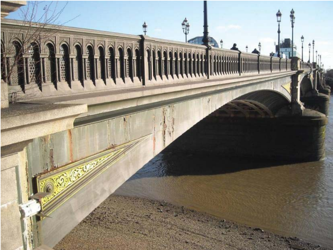
Vol 3 Plate E.20 Bridge viewed from north-west
