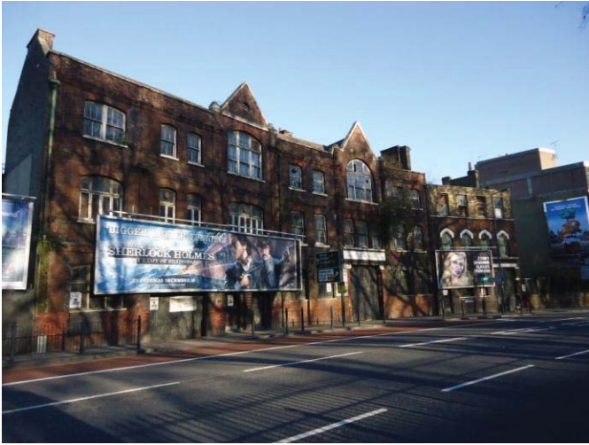
Southern elevation to Commercial Road
