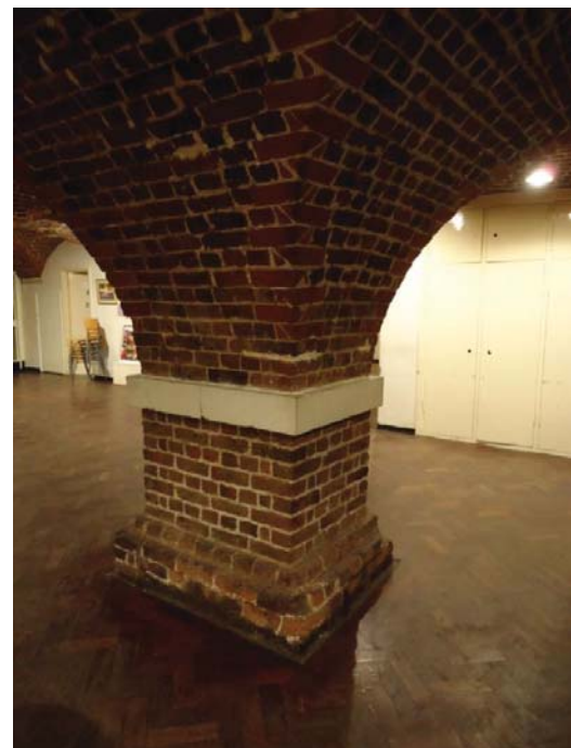
Example of vaulting in the crypt
