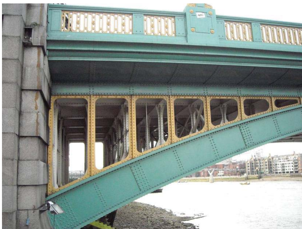
Vol 3 Plate E.89 South abutment viewed from east
