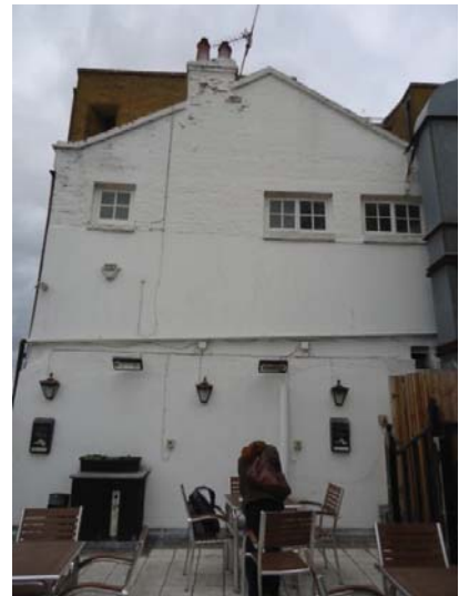
Eastern elevation above ground floor
