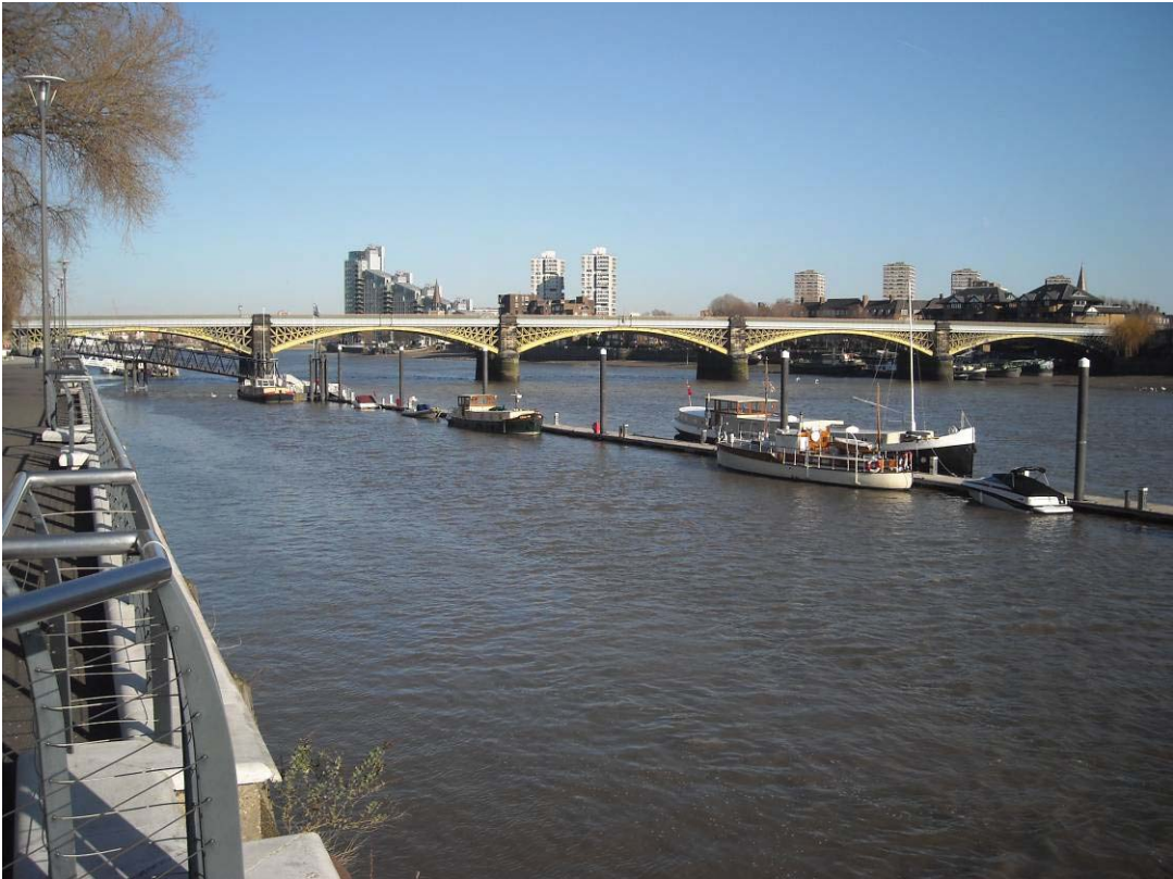
Vol 3 Plate E.40 Bridge viewed from south (upstream)
