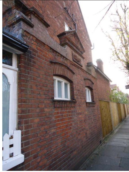
Single storey abutment to 60 Bath Road, with decorative brick
