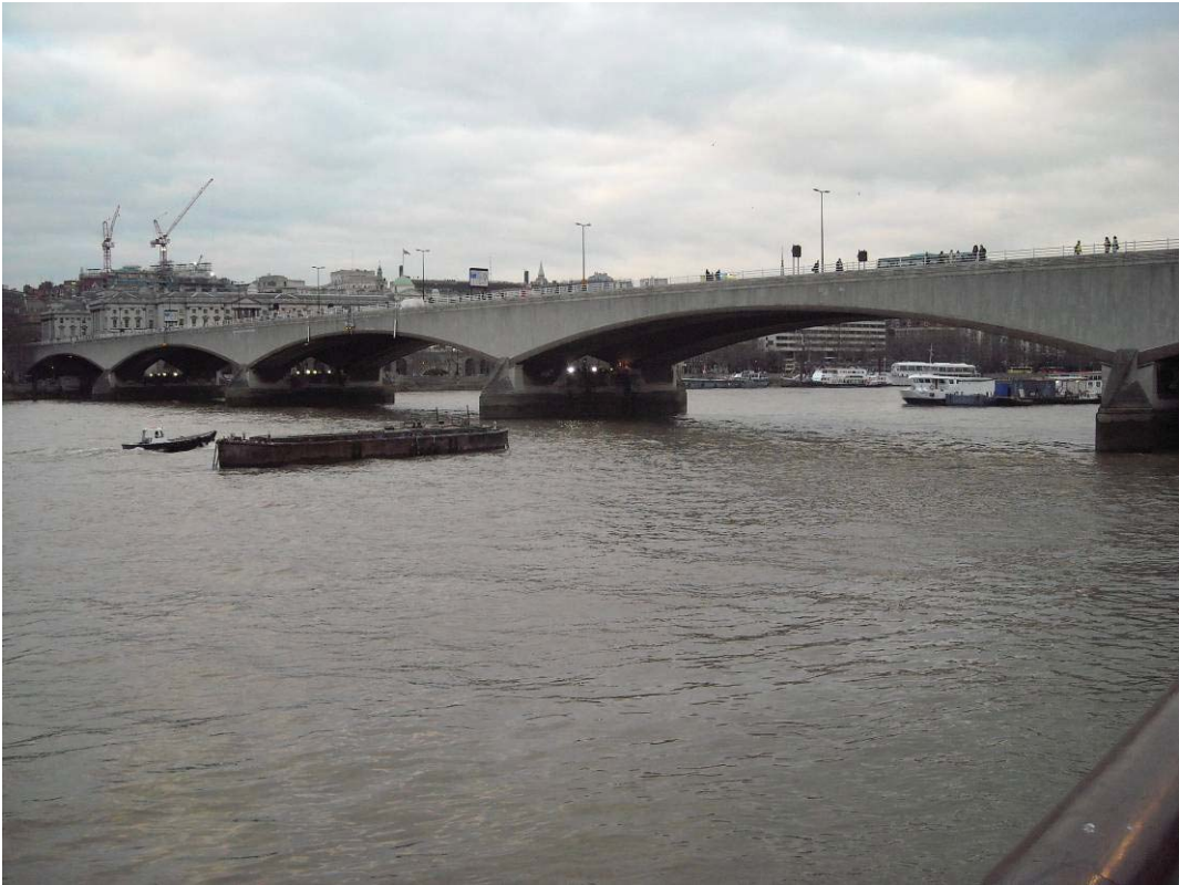
Vol 3 Plate E.74 Waterloo Bridge viewed from south-west
