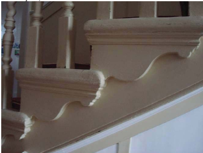
Detail of timber stair with turned balusters
