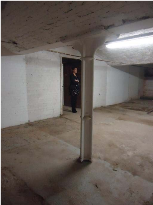
Typical basement view
