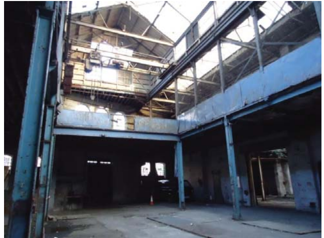
General view of industrial interior
