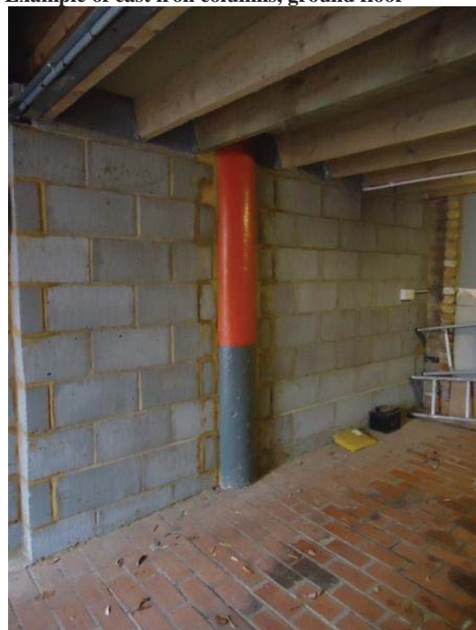
Cast iron column embedded in modern wall, ground floor storage area
