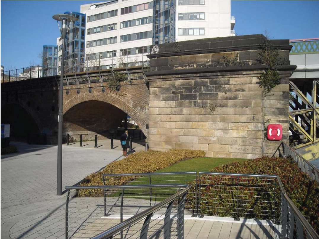
Vol 3 Plate E.45 West abutment with flanking viaduct viewed from south
