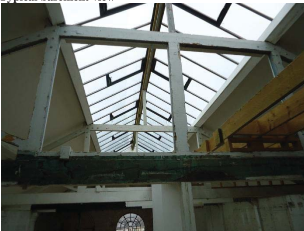
Truss and rooflight in 'D' Warehouse
