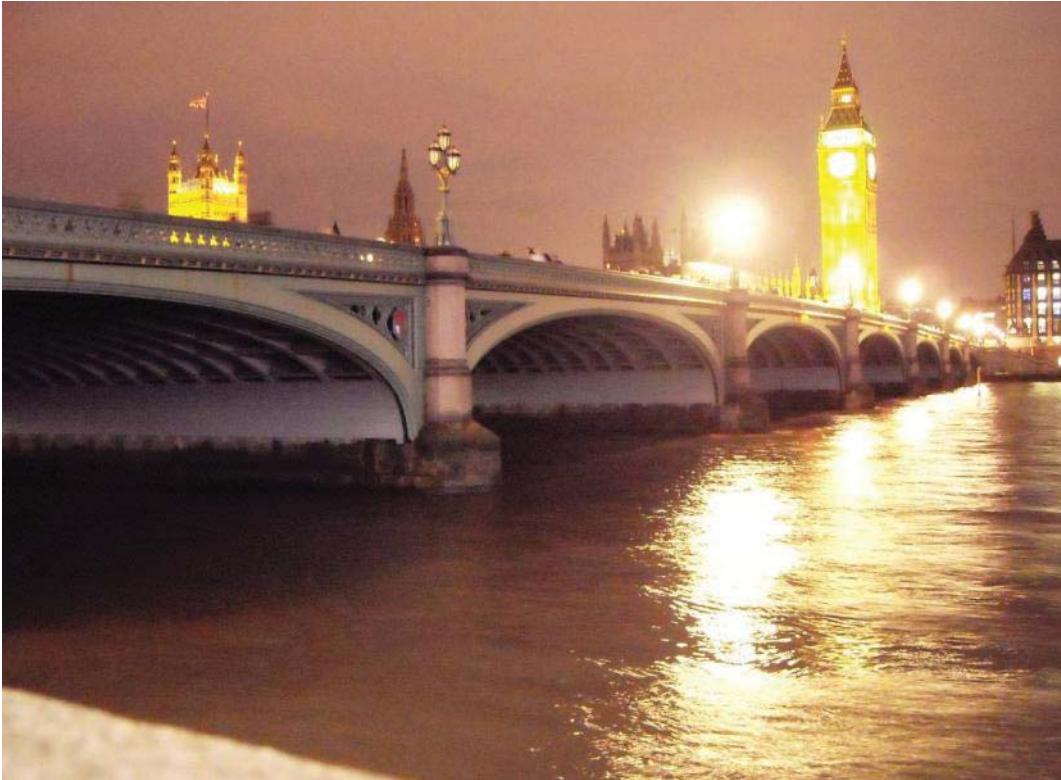
Vol 3 Plate E.71 Bridge viewed from north-east
