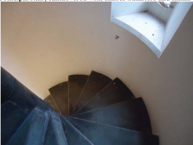
Stone stair within corner tower
