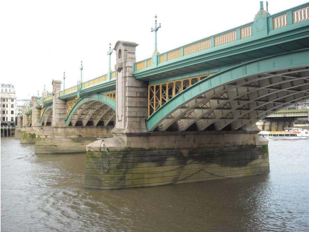
Vol 3 Plate E.86 Bridge viewed from south-west
