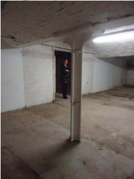
Typical basement view
