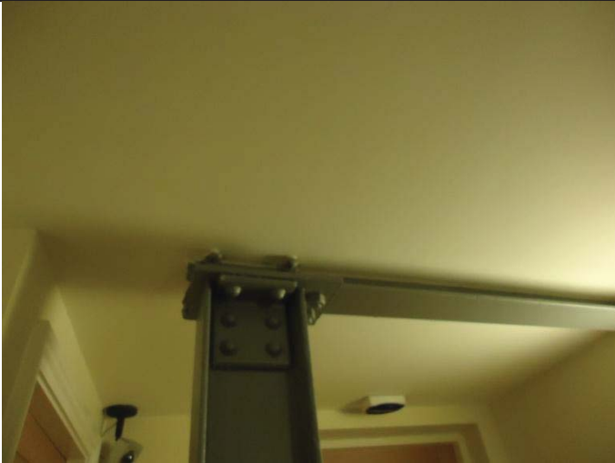
Modern finishes within the public areas
