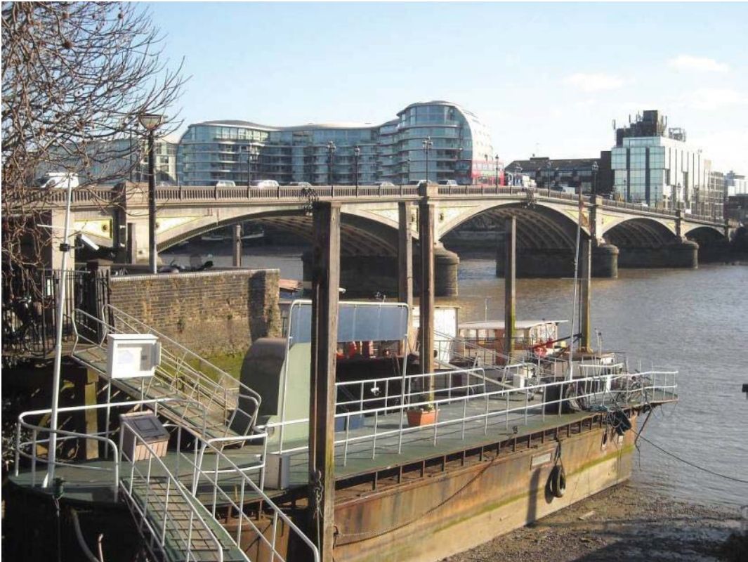
Vol 3 Plate E.19 Bridge viewed from north-west
