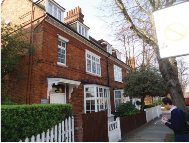
Main (northern) elevation of 62 Bath Road, with 60 to the right
