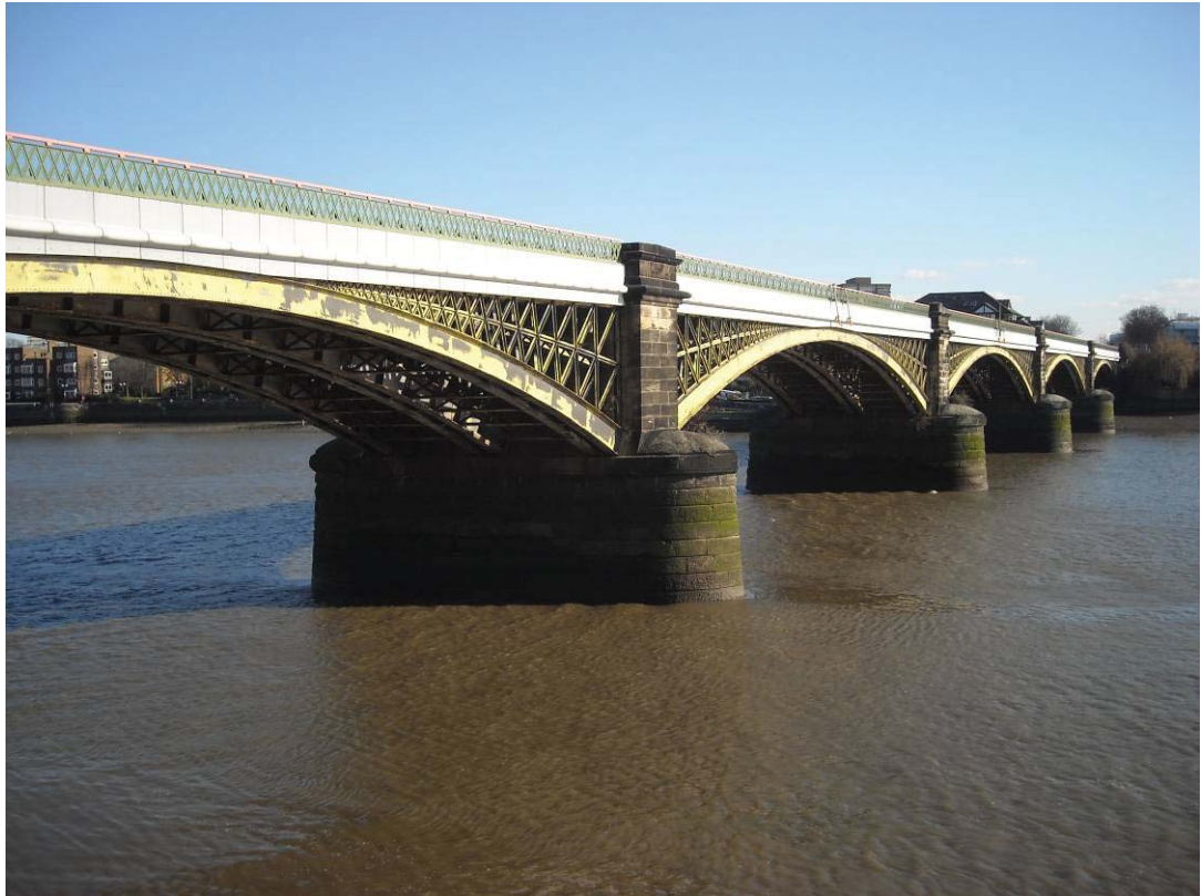
Vol 3 Plate E.42 Bridge viewed from west
