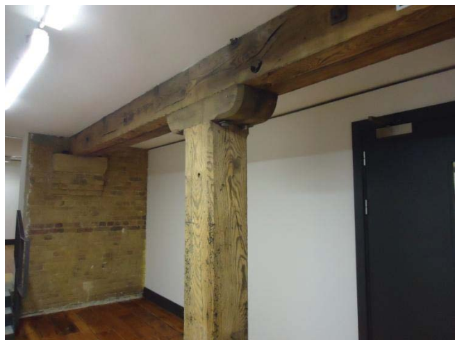
Timber column and beam structure in 'A' Warehouse
