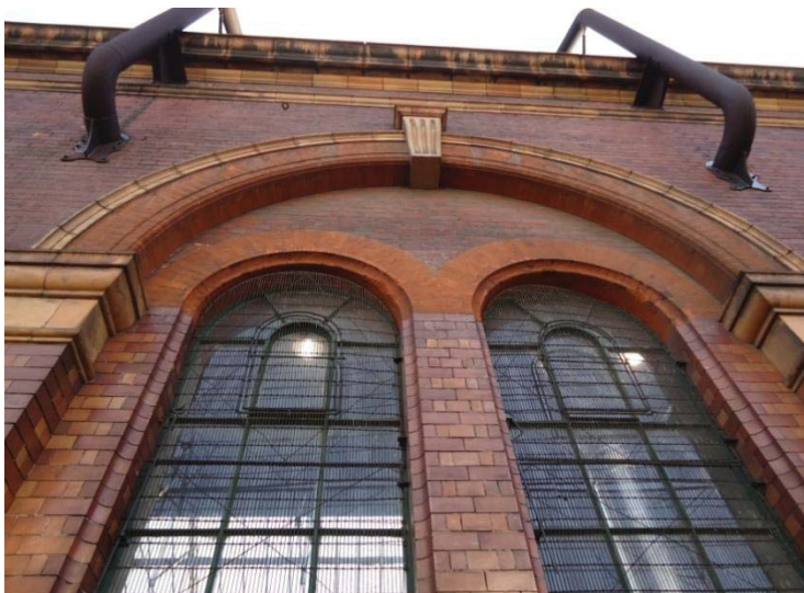
Paired window with terracotta dressings
