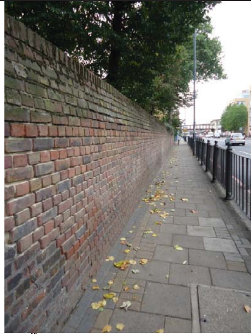
Caption 2: 19 th century section of wall (western end)
