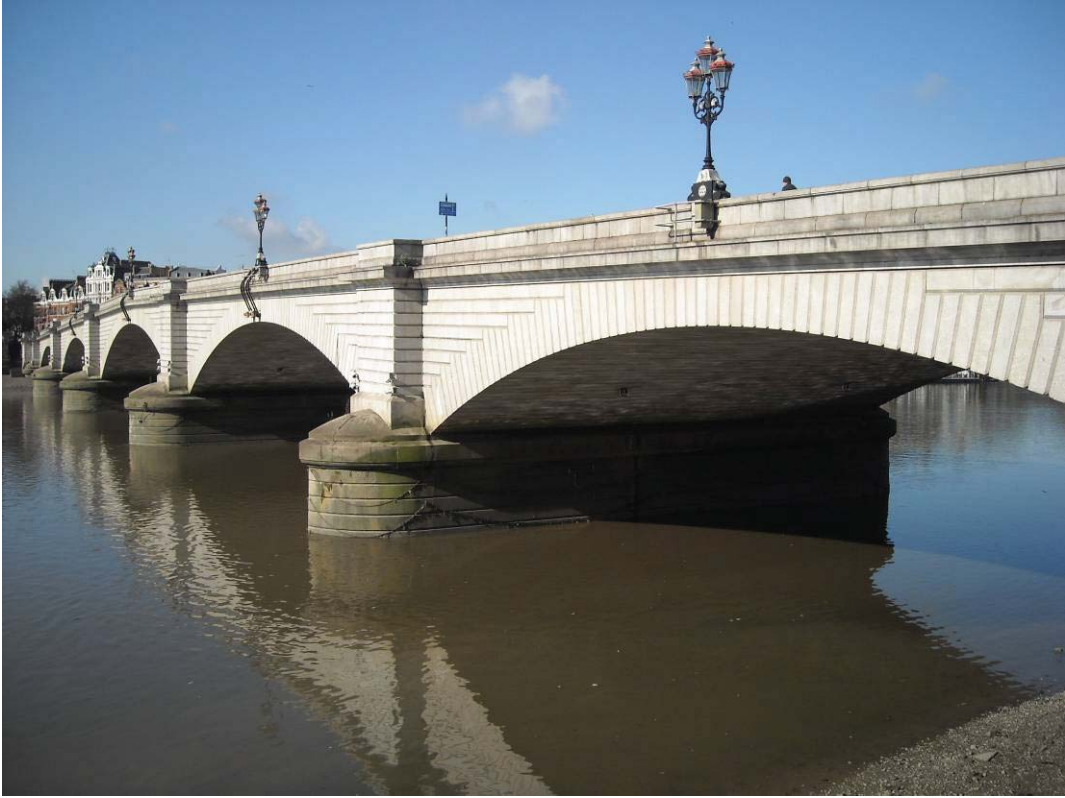
Vol 3 Plate E.8 Putney Bridge viewed from the north-east
