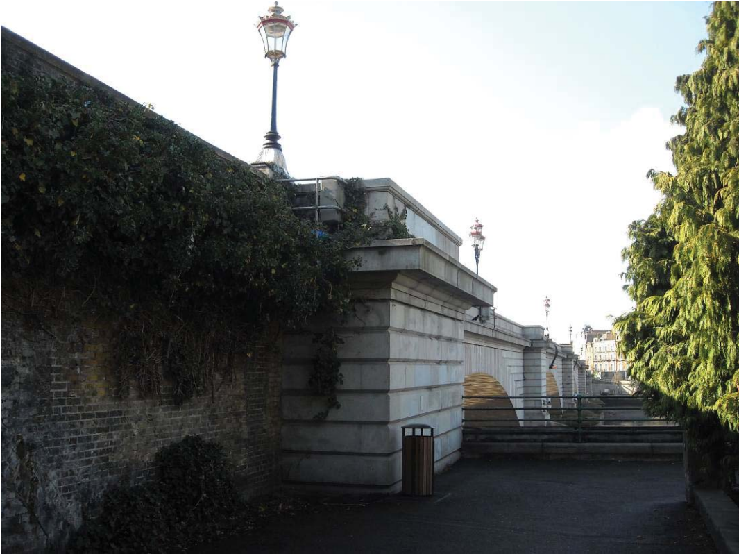
Vol 3 Plate E.11 Putney Bridge viewed from north-west
