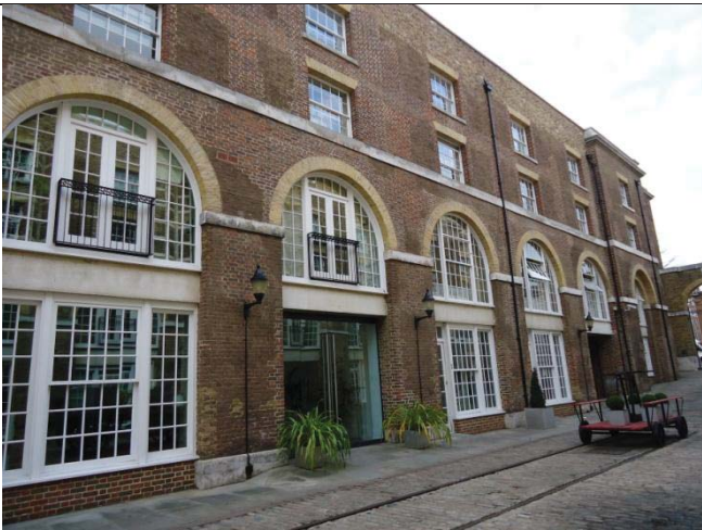
Courtyard elevation of western building, also showing remaining tracks and rails
