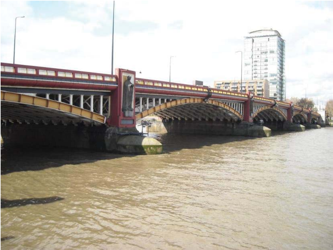
Vol 3 Plate E.53 Bridge viewed from south-west
