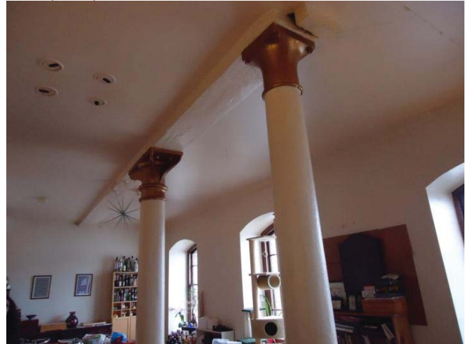
Example of cast iron columns, ground floor
