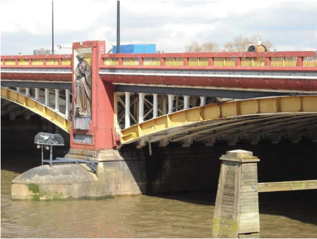
Vol 3 Plate E.49 Detail of bridge viewed from south-west
