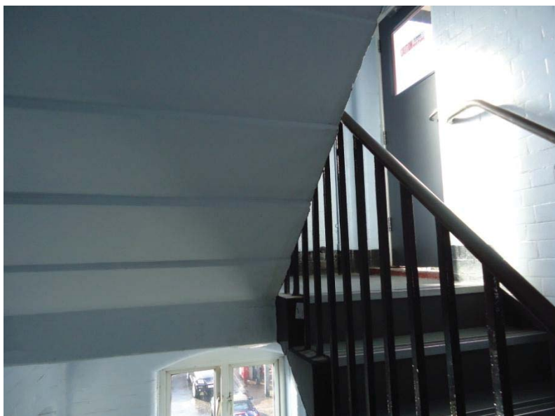
Cantilevered stair
