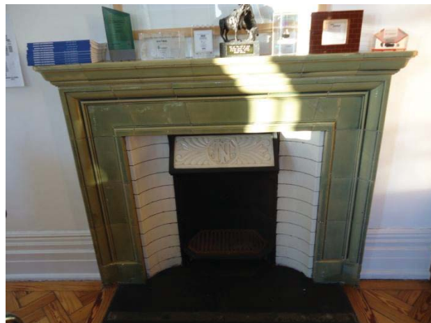
Example of a 'TN' lettered tiled fireplace, found in many of the non-principal rooms to all floors
