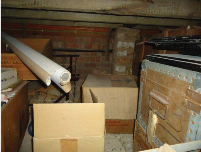
Basement with brick piers
