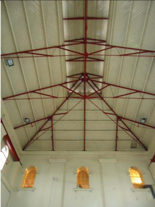
Interior of western section of the west beam engine house
