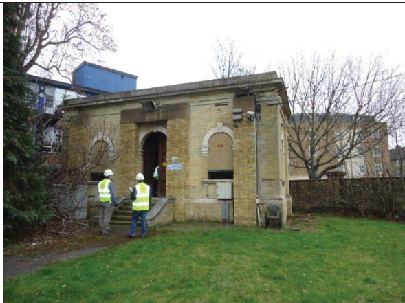
Example of curtilage building on the site, in this case the head stock house
