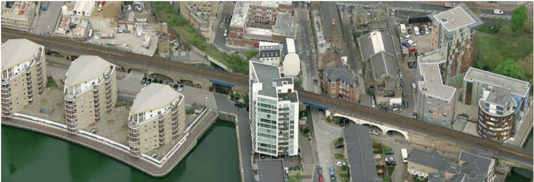
Vol 3 Plate E.125 Aerial view of DLR Viaduct at Island Row viewed from the south
