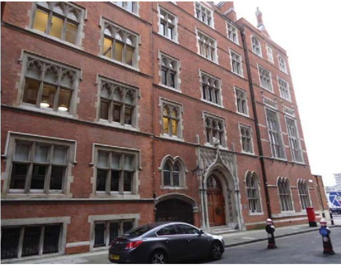
Façade to Carmelite Street
