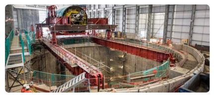
Two tunnel boring machines (TBMs) have been lowered 60m down the shaft at Kirtling Street – the most important construction milestone on the project to date.
