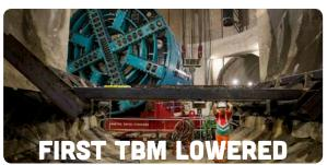
Two giant tunnel boring machines (TBMs) have been lowered 60m down the shaft at Kirtling Street in Battersea. The twin machines, Millicent and Ursula, will be used to dig the central section of the Thames Tideway Tunnel. Site Manager Paul Hallows said: "This is a massive milestone for us."
