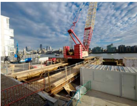
CHAMBERS WHARF, SOUTHWARK
