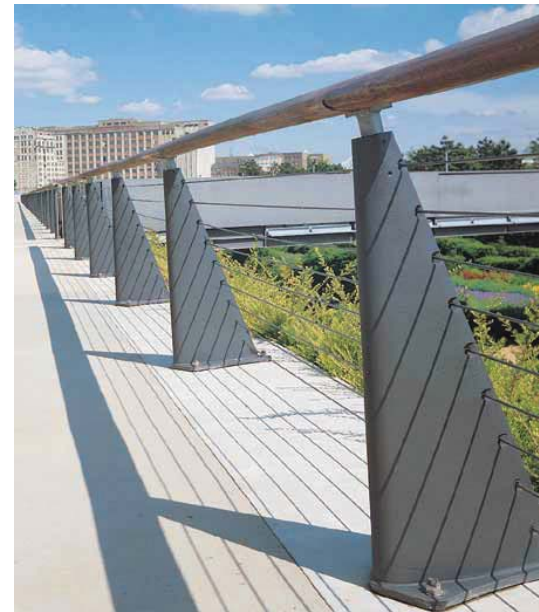
Figure 12.45: Example of handrail
