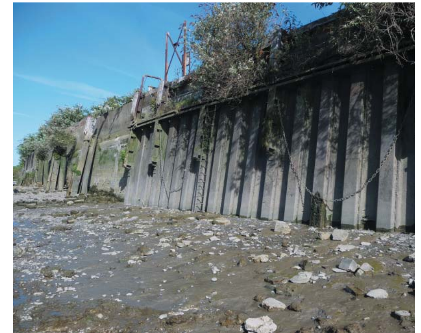
Figure 12.42: Riverwall at existing Carnwath site
