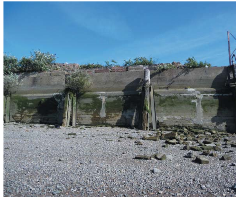
Figure 12.41: River wall at existing Carnwath site
