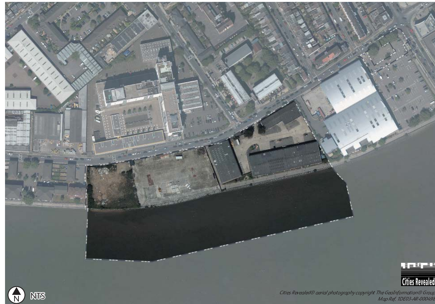
Figure 12.1: Aerial photograph of the existing Carnwath Road Riverside with LLAU indicated
