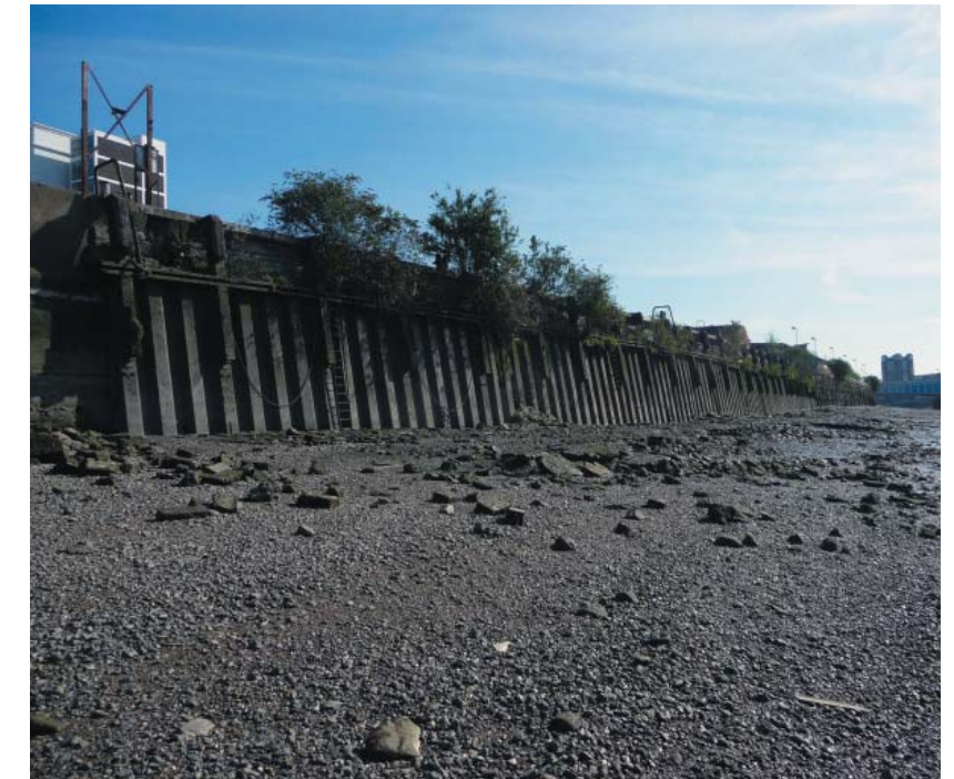
Figure 12.40: River wall at existing Carnwath site
