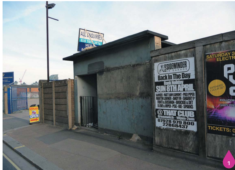
Figure 12.3: Substation on Hurlingham Wharf
