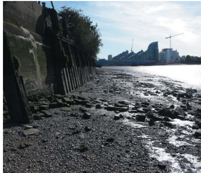
Figure 12.39: River wall at existing Carnwath site
