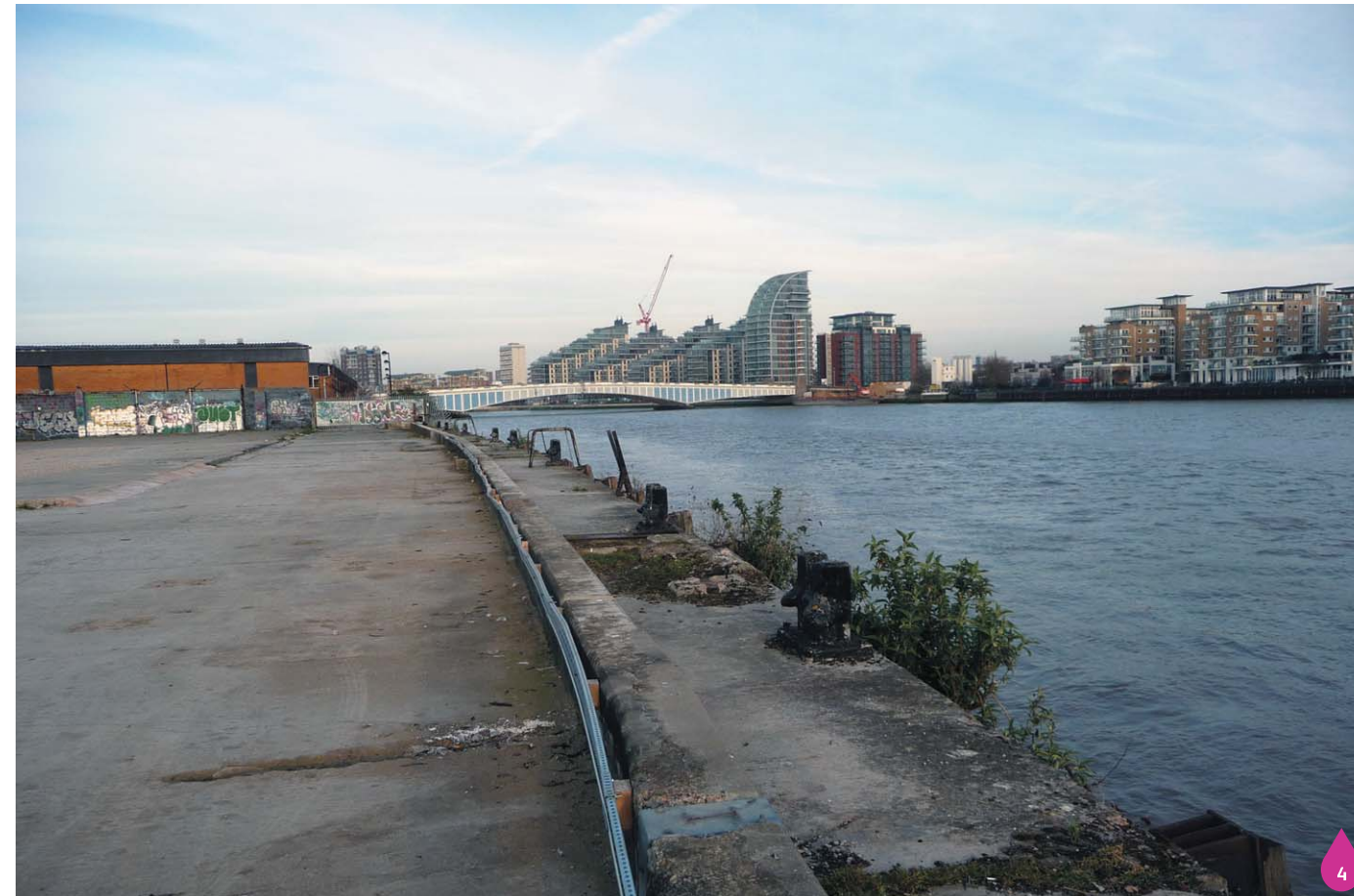
Figure 12.6: River wall at Hurlingham Wharf
