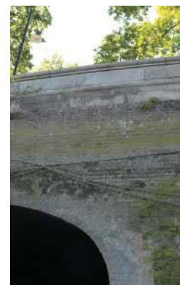
Figure 15.43: River wall showing Parish Boundary marker
