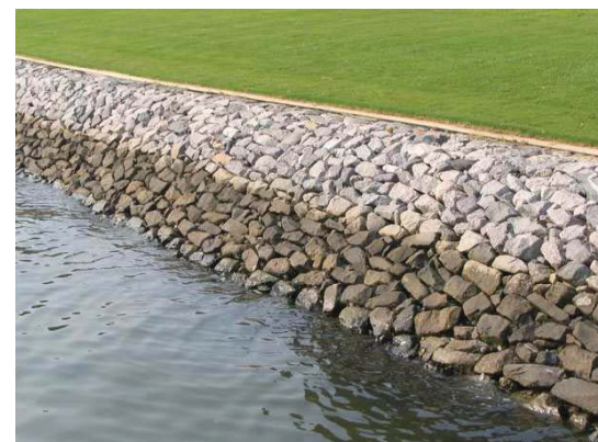
Figure 15.41: Example of 'rip rap scour protection'
