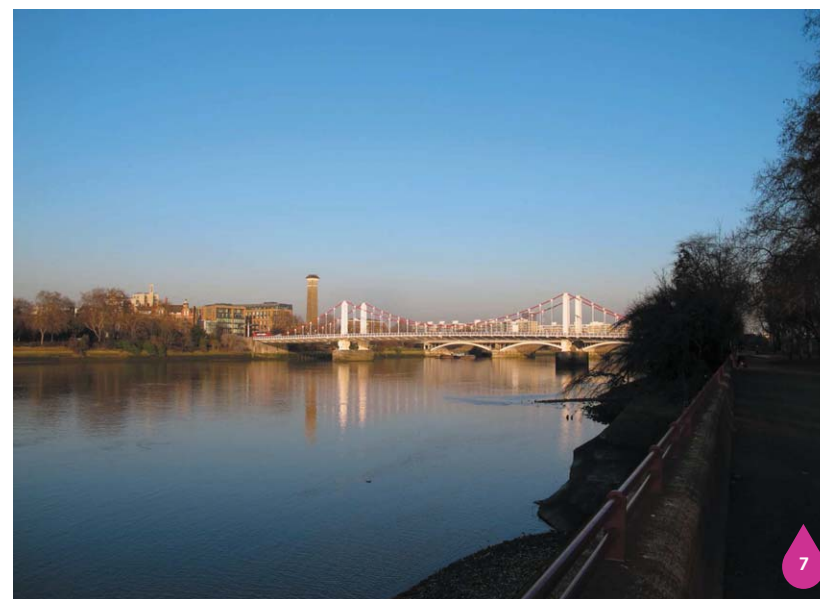
Figure 15.10: Chelsea Bridge from Battersea Park
