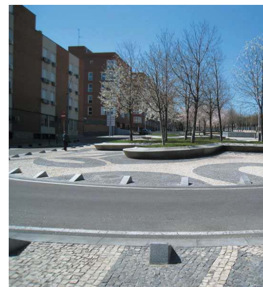
Figure 15.60: Paving and tarmac
