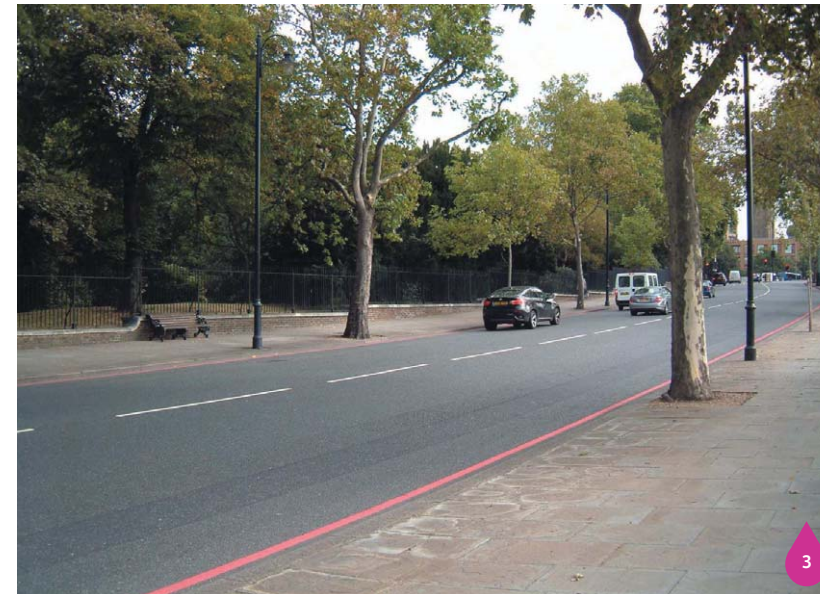
Figure 15.5: Chelsea Embankment looking east towards Chelsea Bridge Road
