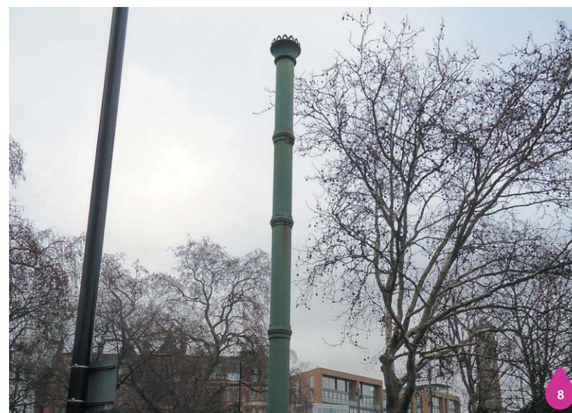
Figure 15.11: Listed sewer vent at Chelsea Embankment
