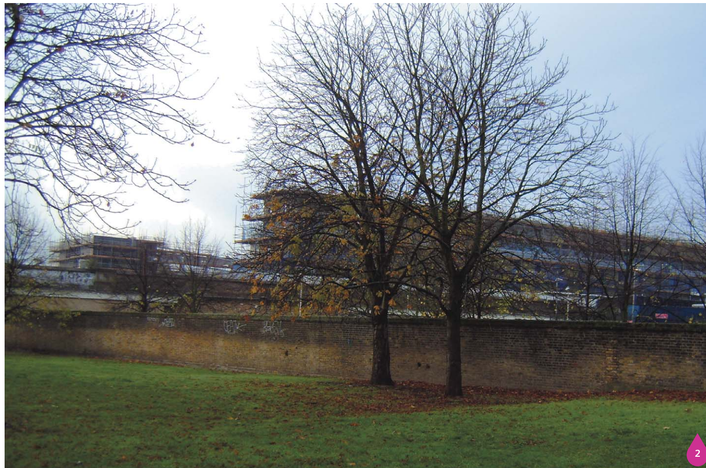
Figure 25.4: View showing existing wall
