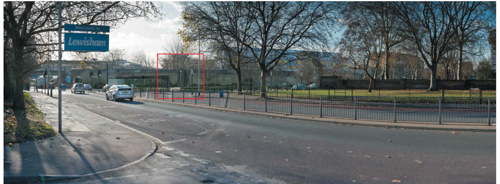
Figure 25.39: View of ventilation columns
