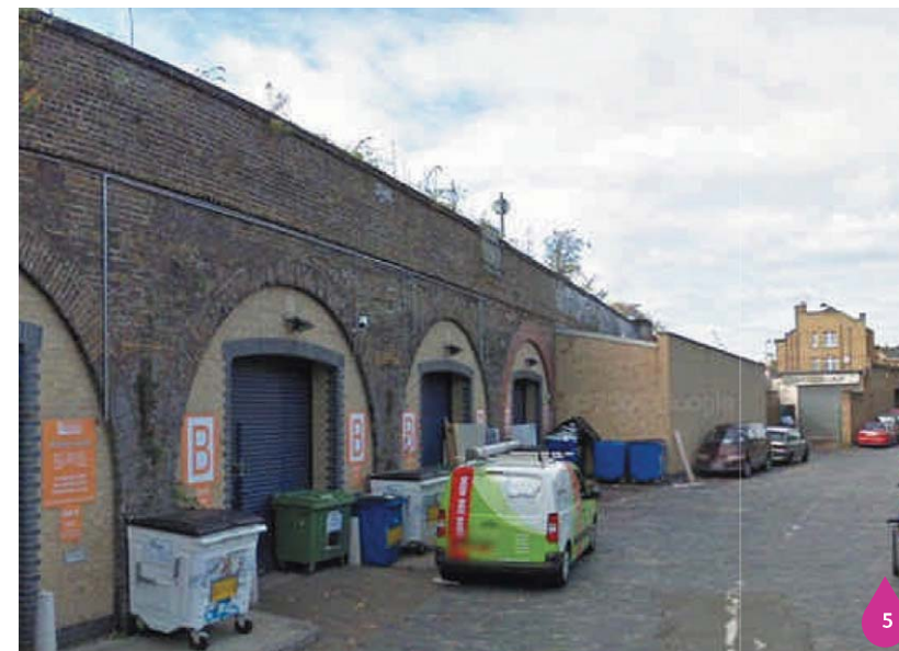
Figure 25.7: View of industrial units in viaduct
