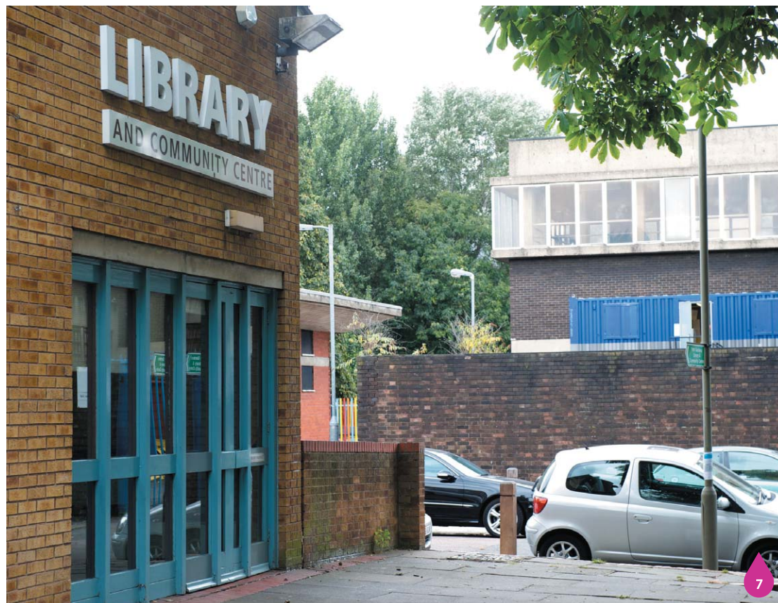
Figure 13.9: Falconbrook Pumping Station and library entrance
