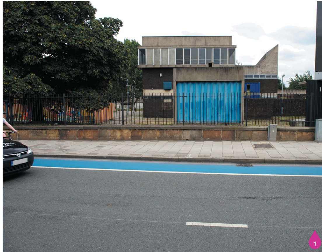
Figure 13.3: Falconbrook Pumping Station from York Way
