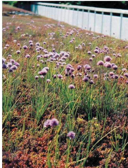
Figure 13.26: Example of planted brown roof
