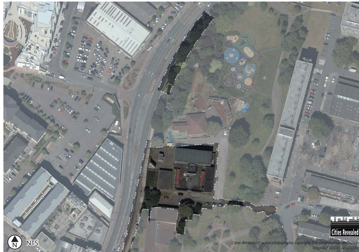
Figure 13.1: Aerial photograph of the existing Falconbrook Pumping Station site with LLAU indicated
