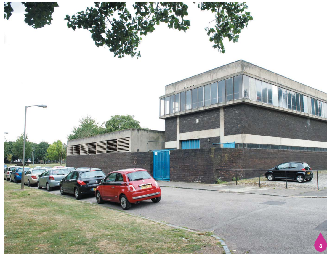
Figure 13.11: Falconbrook Pumping station from York Gardens
