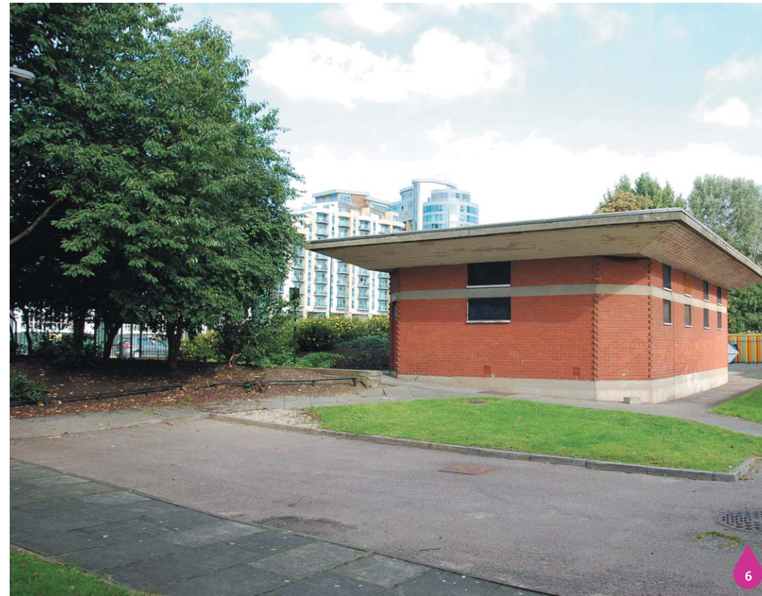
Figure 13.10: Disused toilet block
