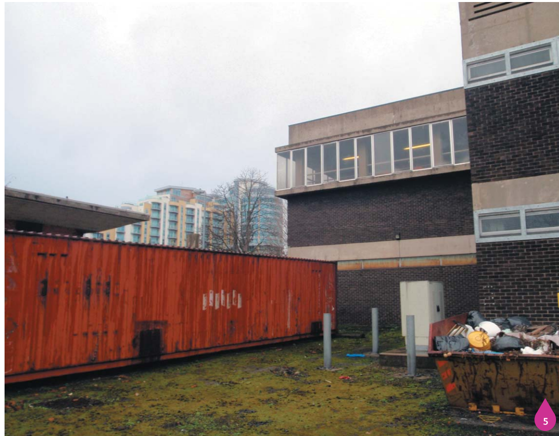
Figure 13.8: Falconbrook Pumping Station from within the compound
