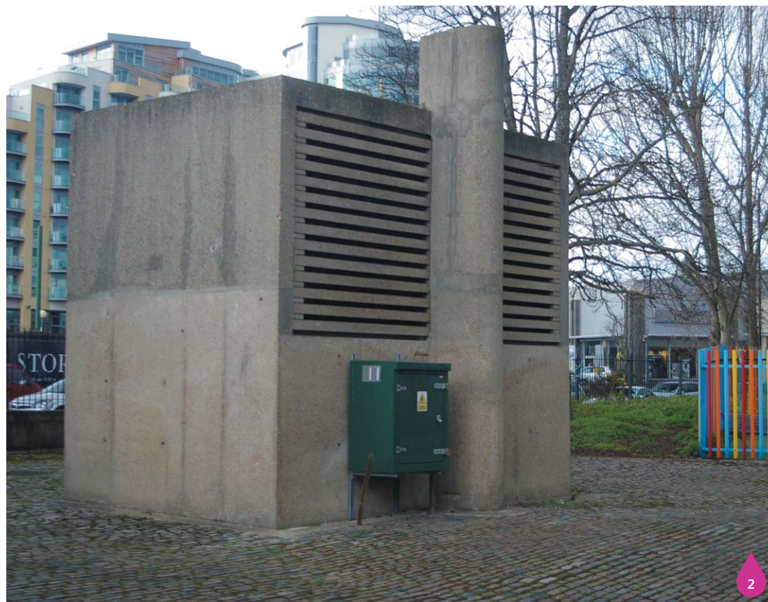
Figure 13.4: Existing concrete ventilation building and cobbled paving
