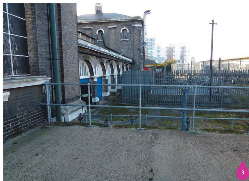
Figure 26.5: East Beam Engine House
