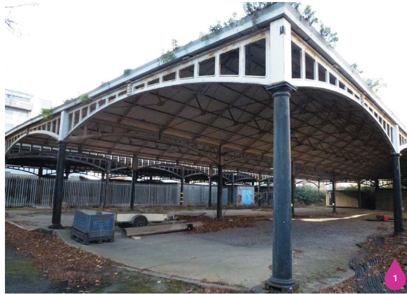
Figure 26.3: Existing coal shed
