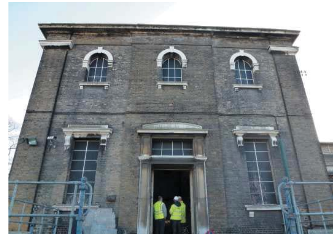
Figure 26.23: Investigation into the use of the East Beam Engine House
