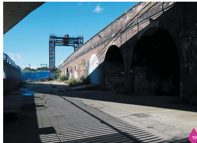
Figure 26.14: View along Listed Viaduct
