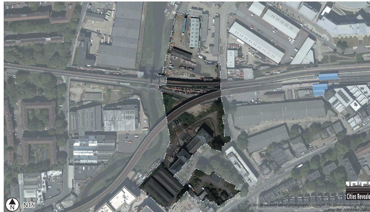
Figure 26.1: Aerial photograph of the existing Greenwich Pumping Station site with LLAU indicated
