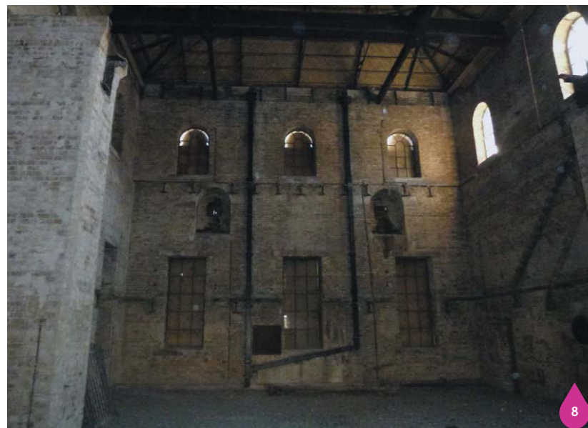
Figure 26.11: Interior of East Beam Engine House
