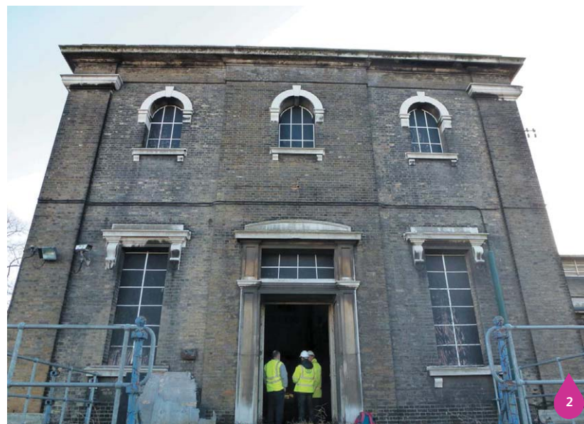
Figure 26.4: East Beam Engine House
