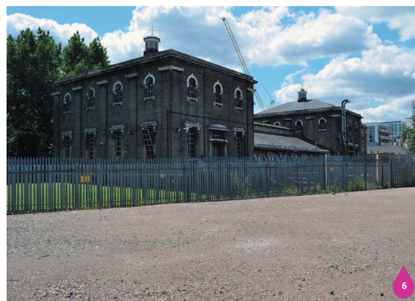
Figure 26.8: East Beam Engine House
