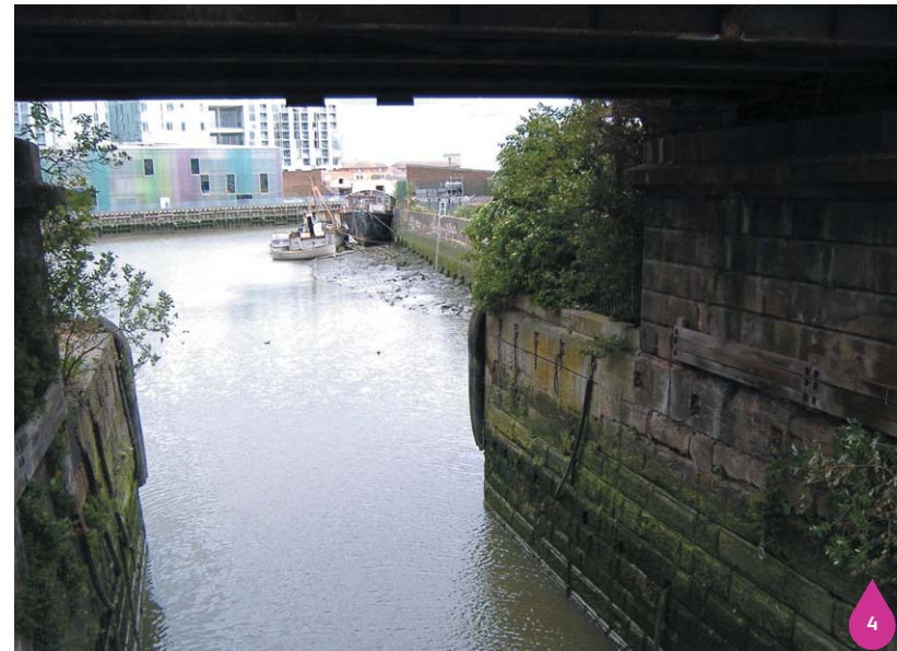
Figure 26.6: View from under bridge on Deptford Creek toward Laban Centre
