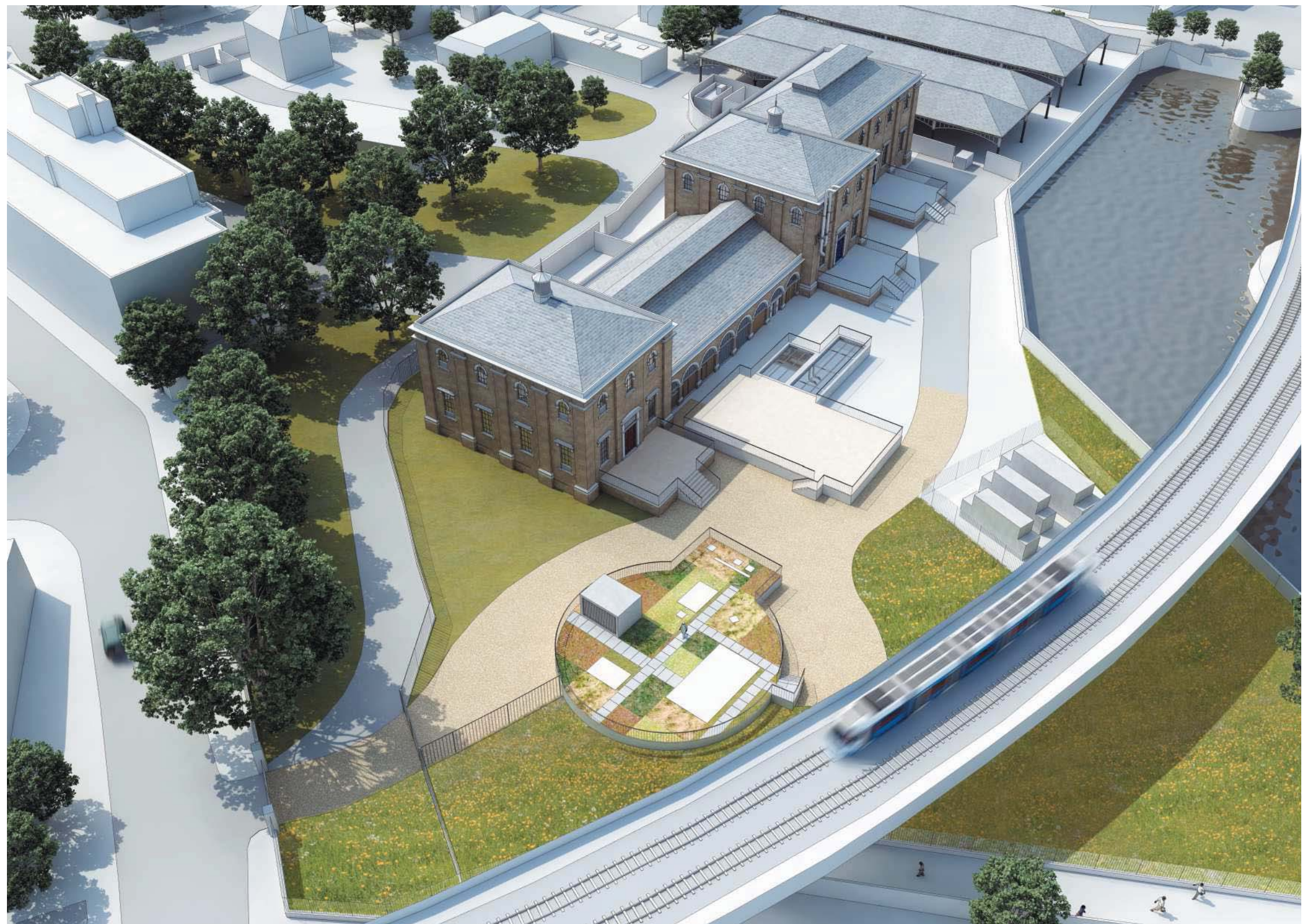
Figure 26.29: Works within the compound
