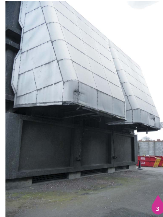
Figure 7.5: Screen house building within compound
