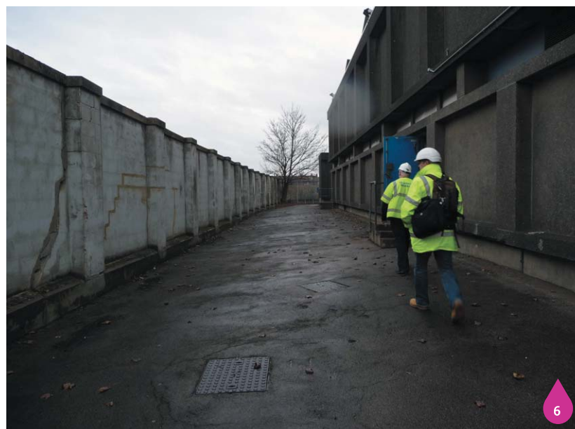
Figure 7.8: Along southern boundary within compound
