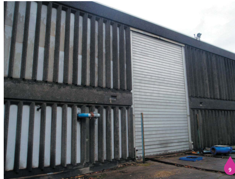
Figure 7.12: Access doors in the western elevation of pumping station
