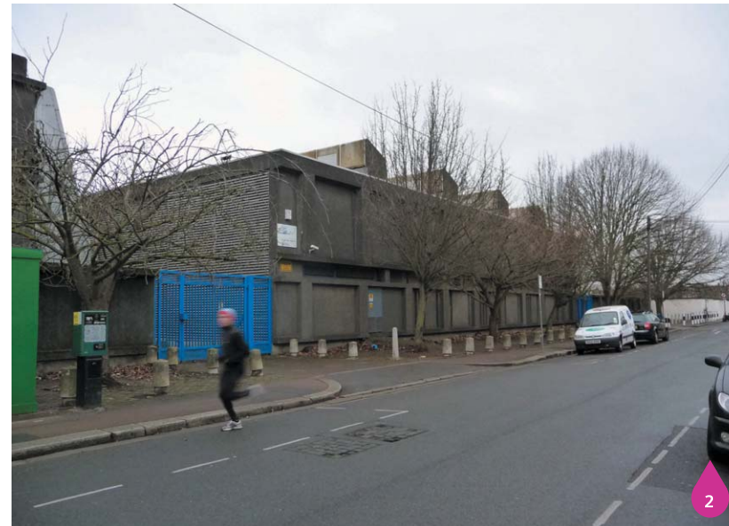
Figure 7.4: Pumping station on Chancellor's Road
