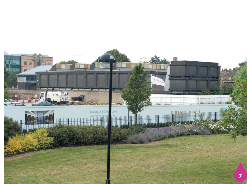
Figure 7.9: Fulham reach development site with pumping station behind
