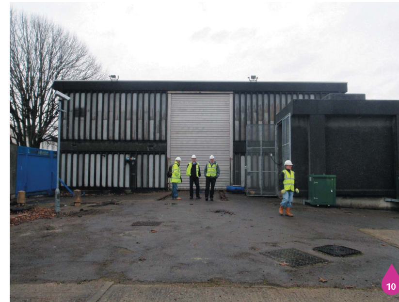
Figure 7.13: West elevation of pumping station and Venturi building
