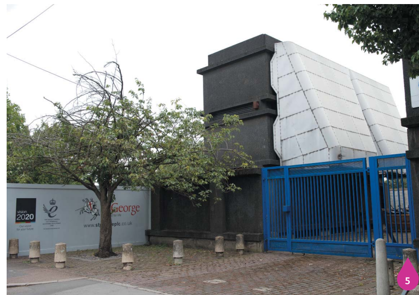
Figure 7.7: Screen house building outside compound
