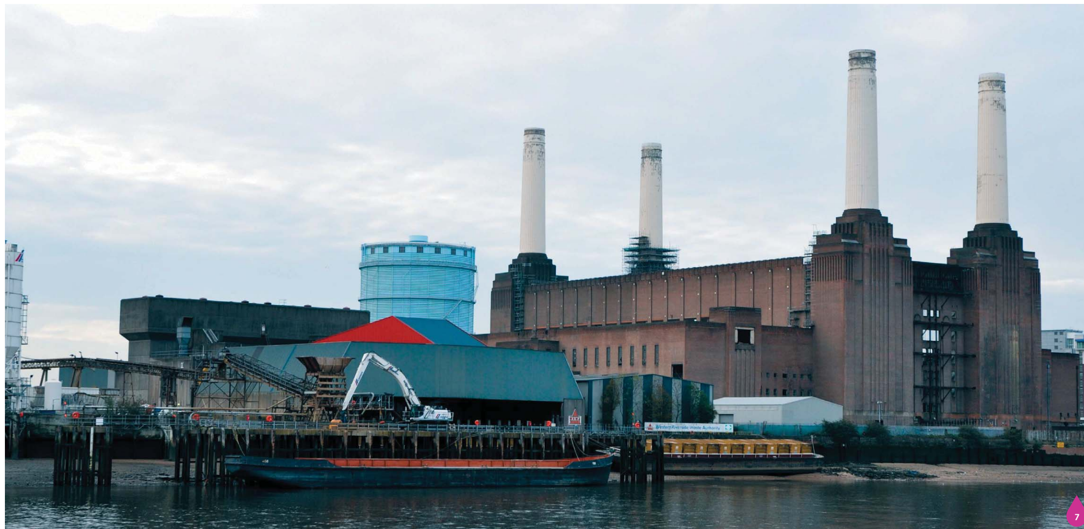
Figure 16.12: Existing site and Battersea Power Station from the River Thames
