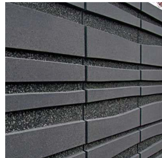
Figure 16.36: Example of high quality patterned concrete
