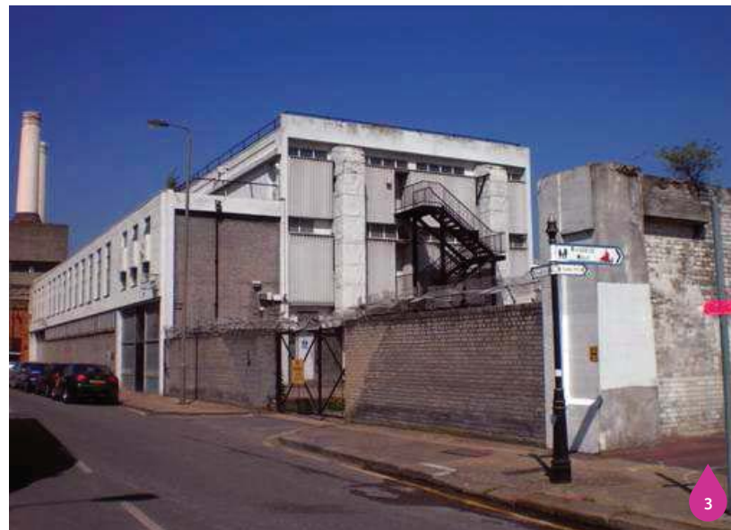
Figure 16.5: Existing warehouse on site
