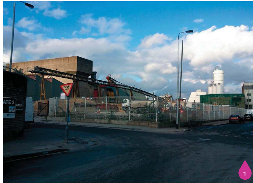
Figure 16.3: Existing site and access to concrete Batching works
