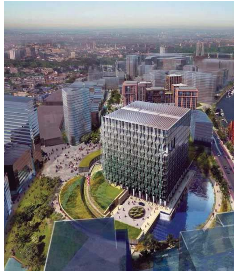
Figure 16.17: Visualisation of approved US Embassy and Embassy Gardens developments and wider Nine Elms developments by others (from east) © US Embassy
