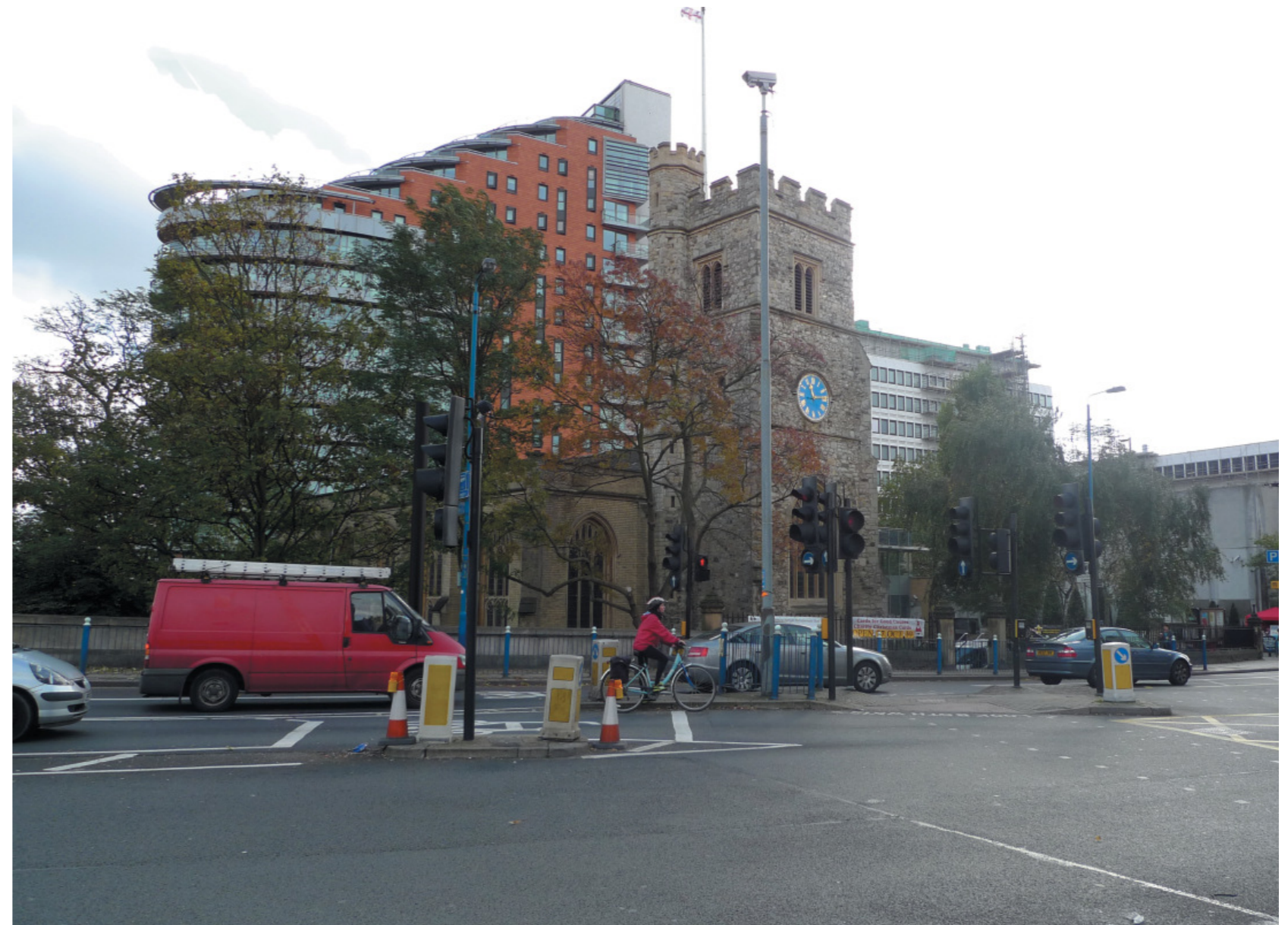
Figure 9.32: Proposed view of ventilation column in front of Grade II* listed St Mary's church
