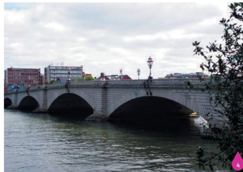
Figure 9.6: Putney Bridge from Lower Richmond Road looking east
