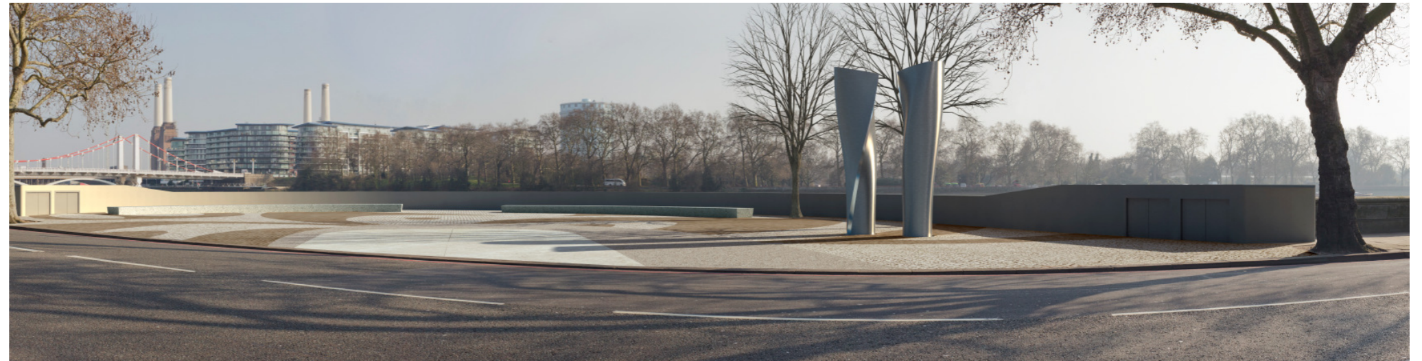
Figure 5.38: Type B ventilation columns at Chelsea Embankment Foreshore
