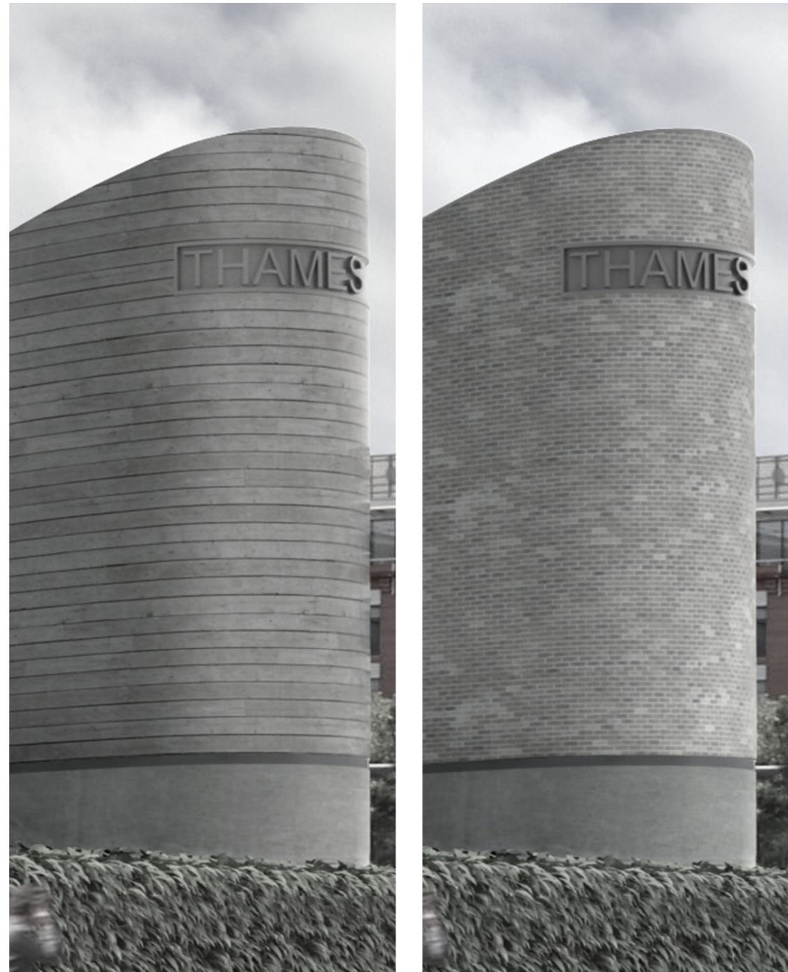
Figure 5.20: Design development images for a phase one consultation combined kiosk and ventilation structure
