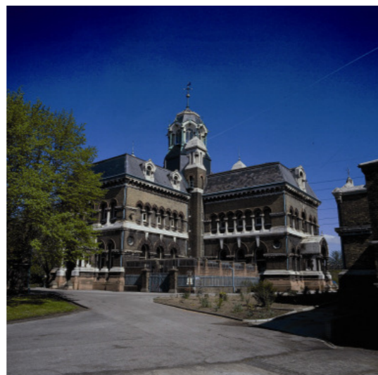
Figure 5.34: Photograph of the Historic Abbey Mills Pumping Station A
