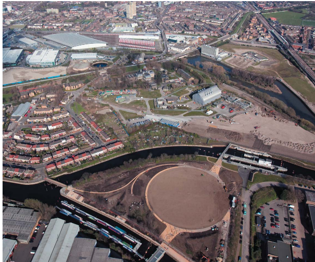
Figure 27.3: Existing aerial view of Abbey Mills Pumping Station site and surroundings
