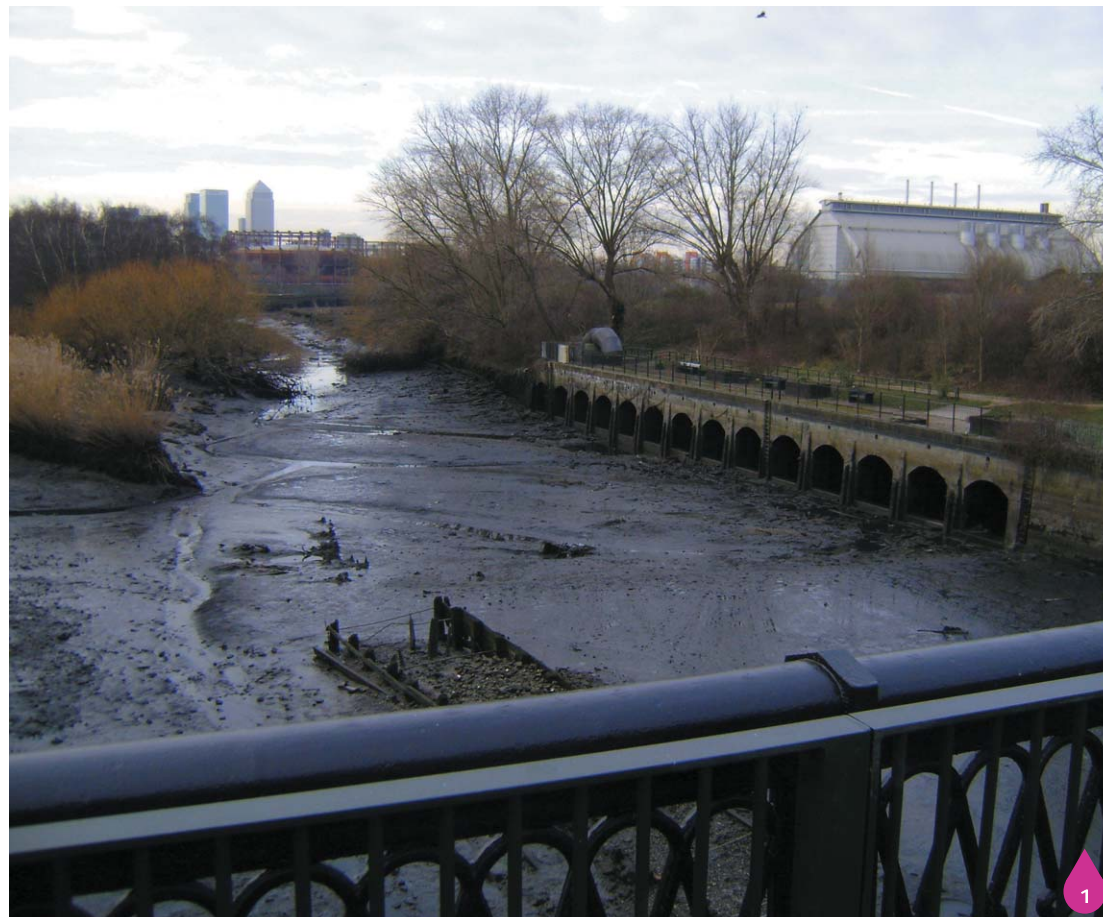
Figure 27.4: View of the Abbey Mills Pumping Station site F and Abbey Creek from the Greenway
