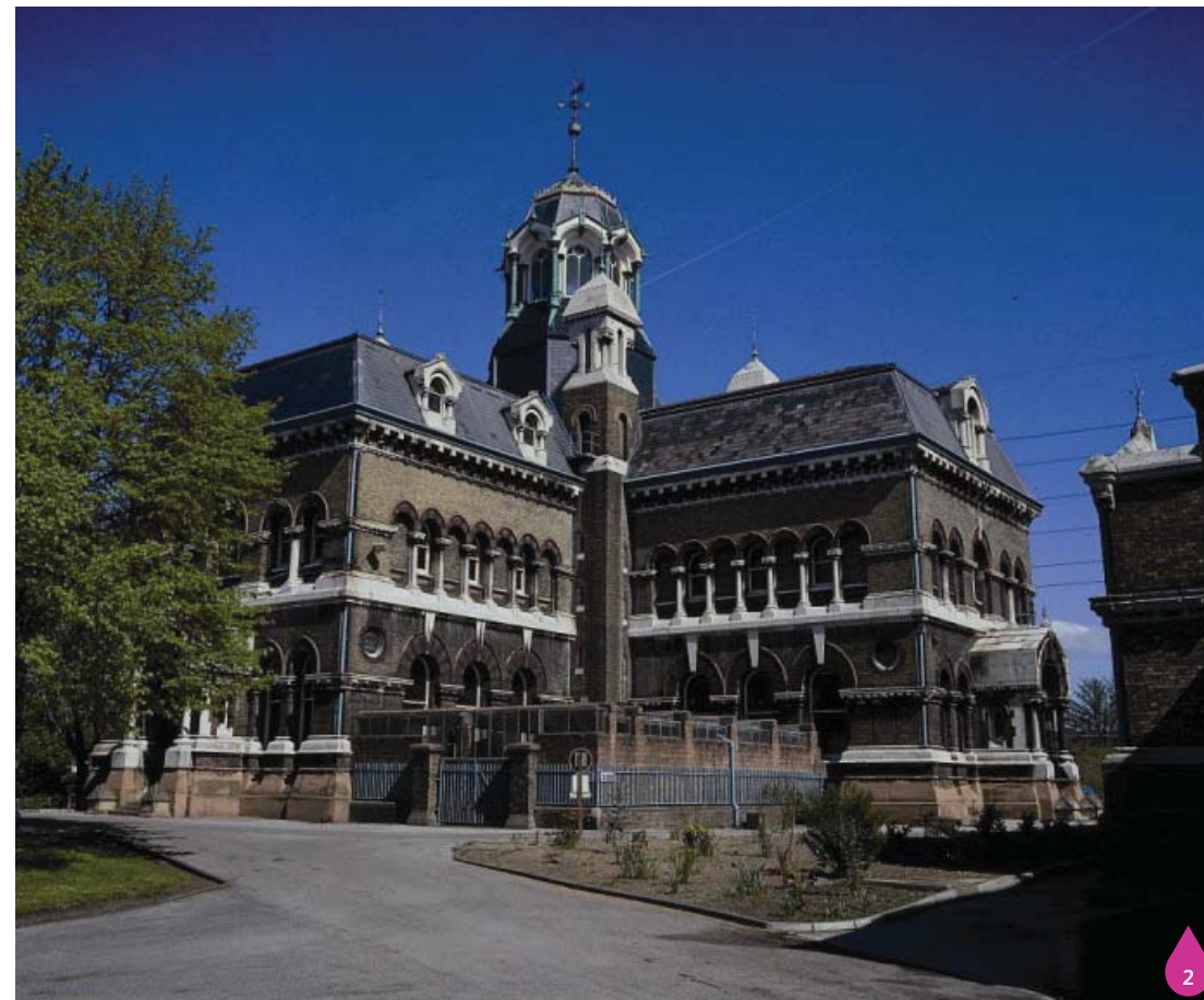
Figure 27.6: View of the Abbey Mills Pumping station A
