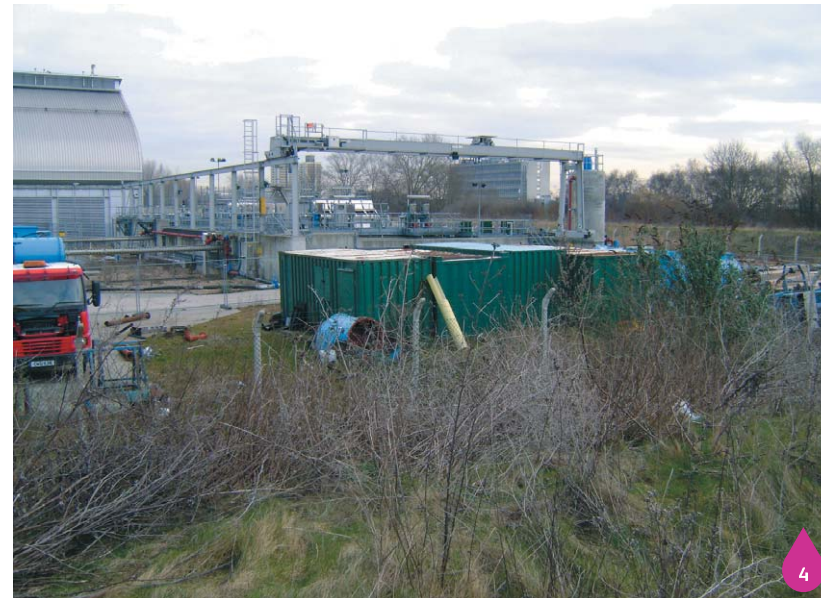
Figure 27.10: View within Abbey Mills Pumping Station site
