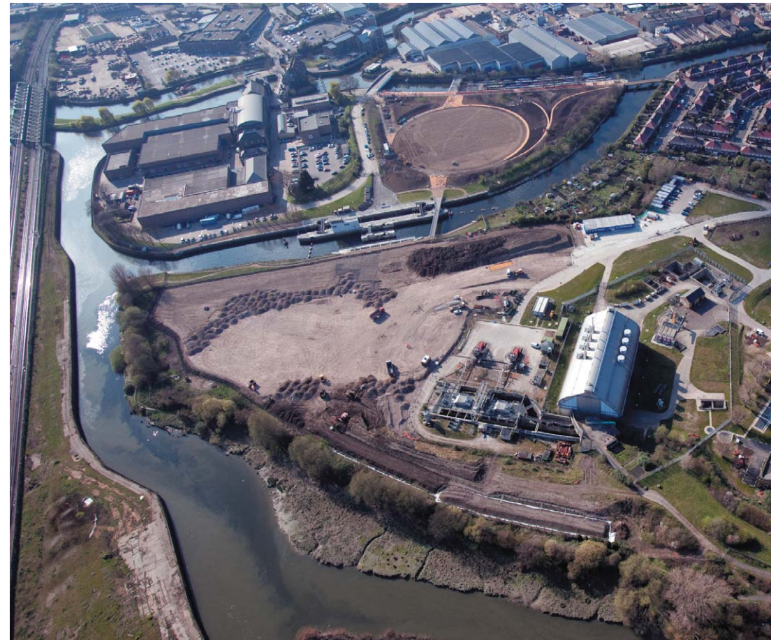
Figure 27.5: Existing aerial view of Abbey Mills Pumping Station site and surroundings
