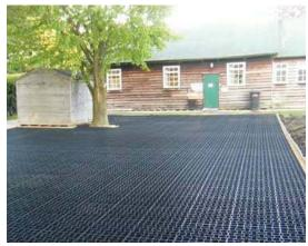
Figure 8.43: Access road ground reinforcement
