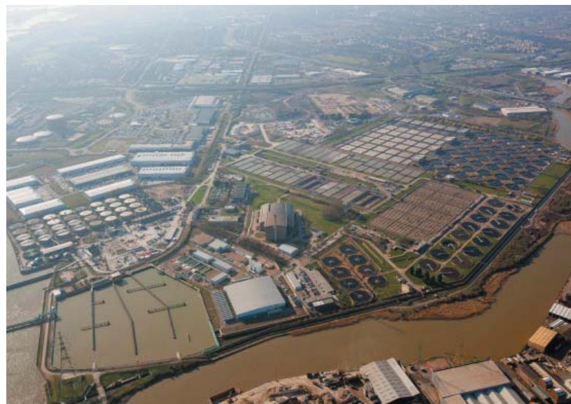
Figure 28.5: Aerial view of proposed site from South East
