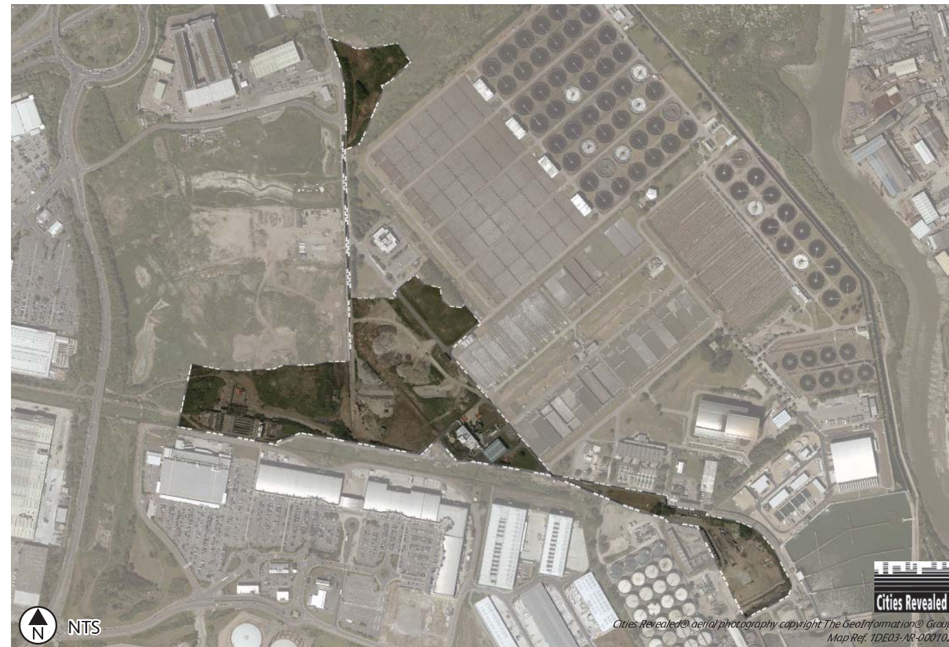
Figure 28.1: Aerial photograph of the existing Beckton Sewage Treatment Plant site with LLAU indicated
