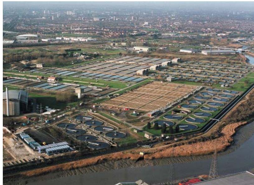
Figure 28.3: Aerial view of proposed site from East
