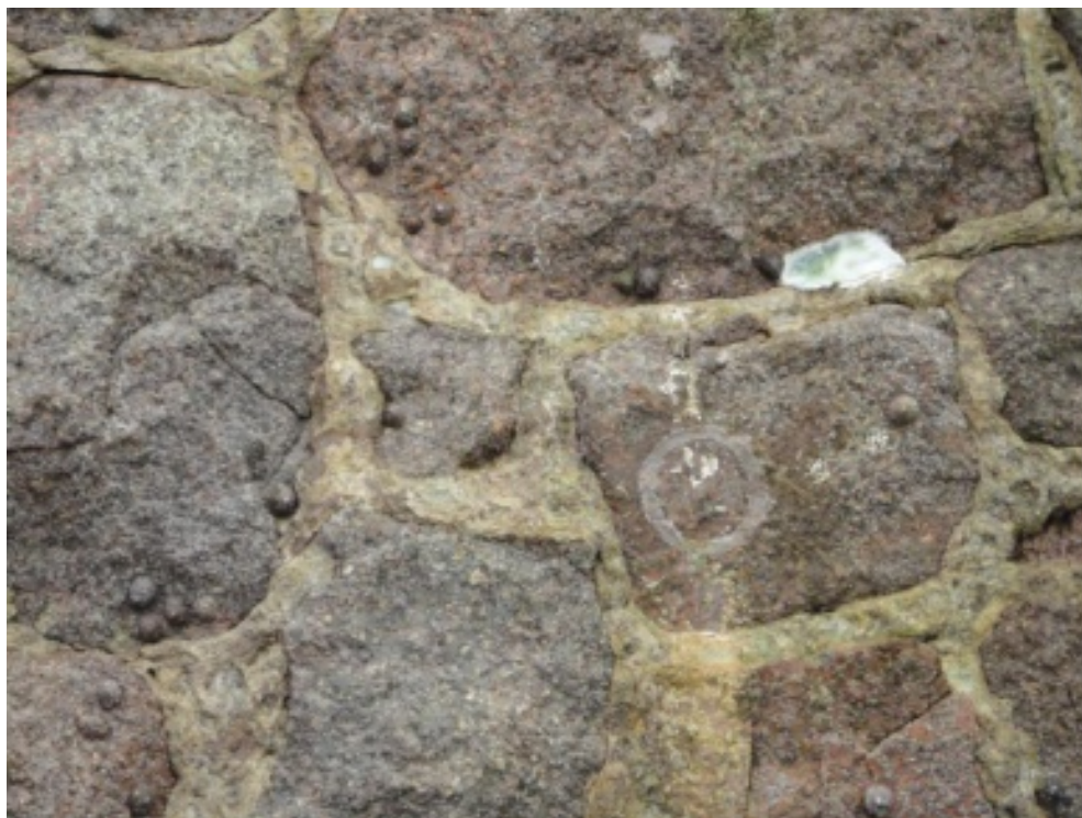
Figure 2.1: Example of stone plug - St. Aubin’s Harbour
