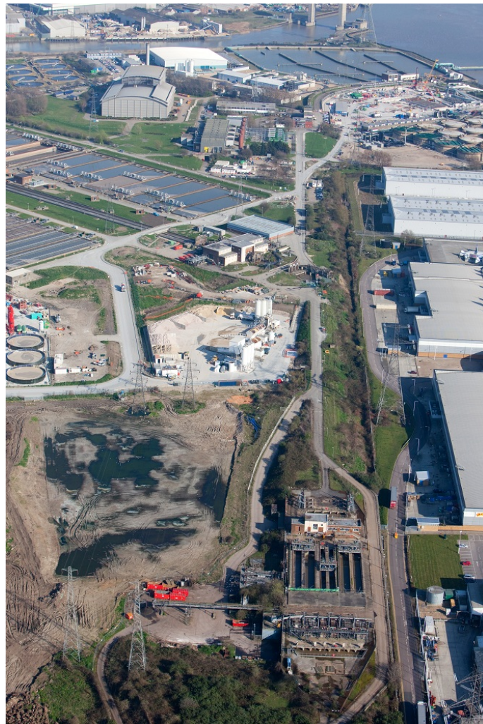
Figure Y.1 Aerial photograph of Beckton Sewage Treatment Works
