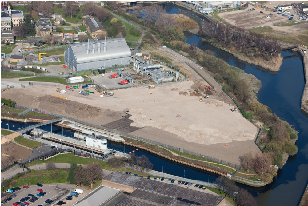
Figure X.1 Aerial photograph of Abbey Mills Pumping Station
