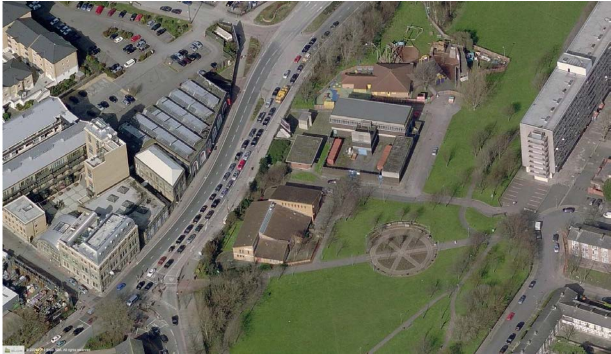
Figure H.1 Aerial photograph of Falconbrook Pumping Station
