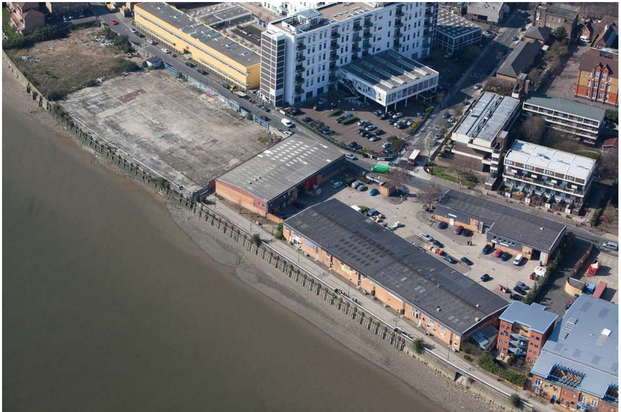
Figure G.1 Aerial photograph of Carnwath Road Riverside
