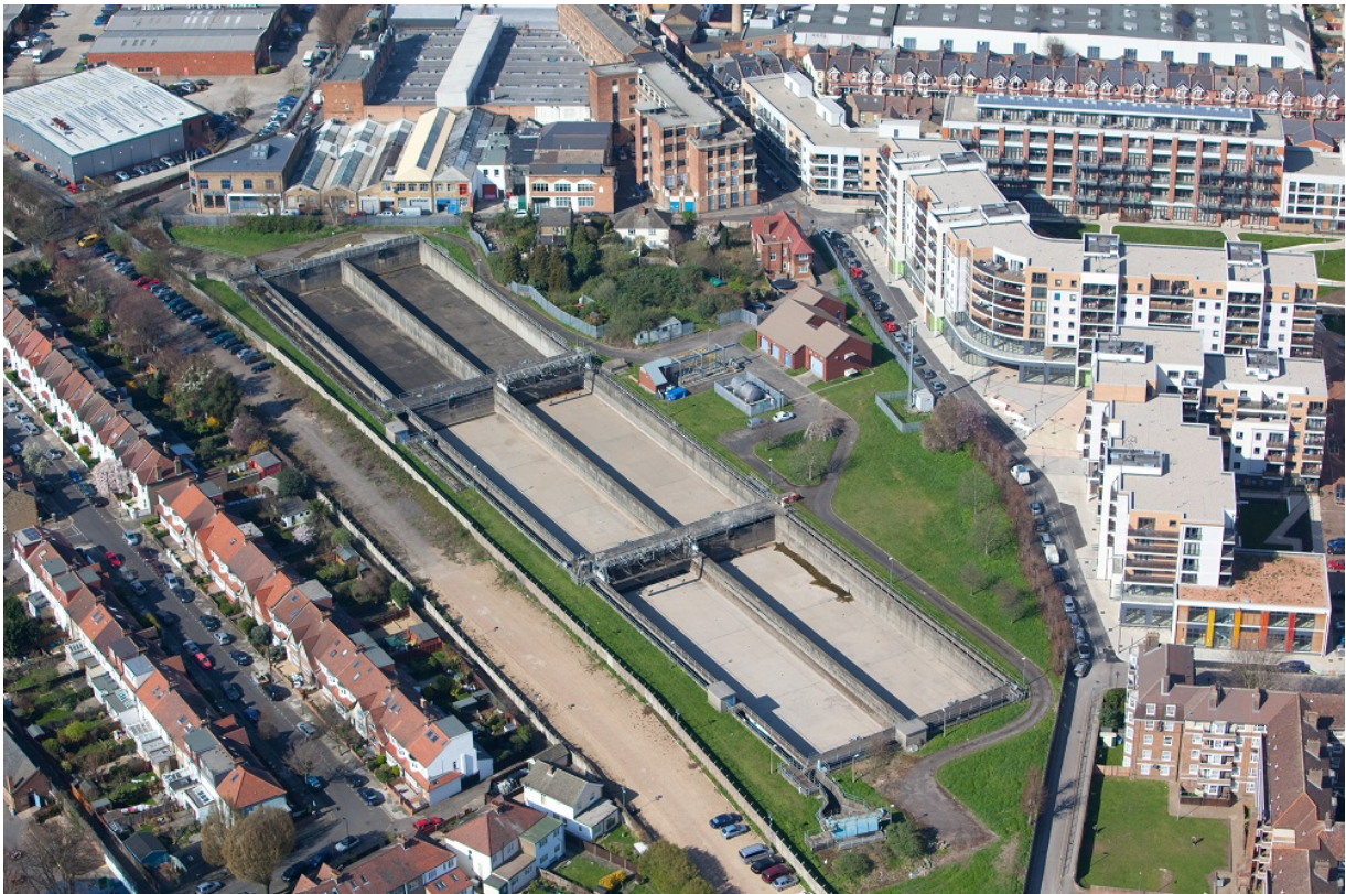
Figure A.1 Aerial photograph of Acton Storm Tanks
