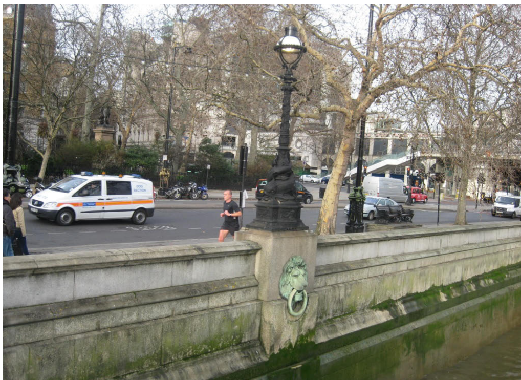
Figure H.1 View from the Tattershall Castle towards the river wall
