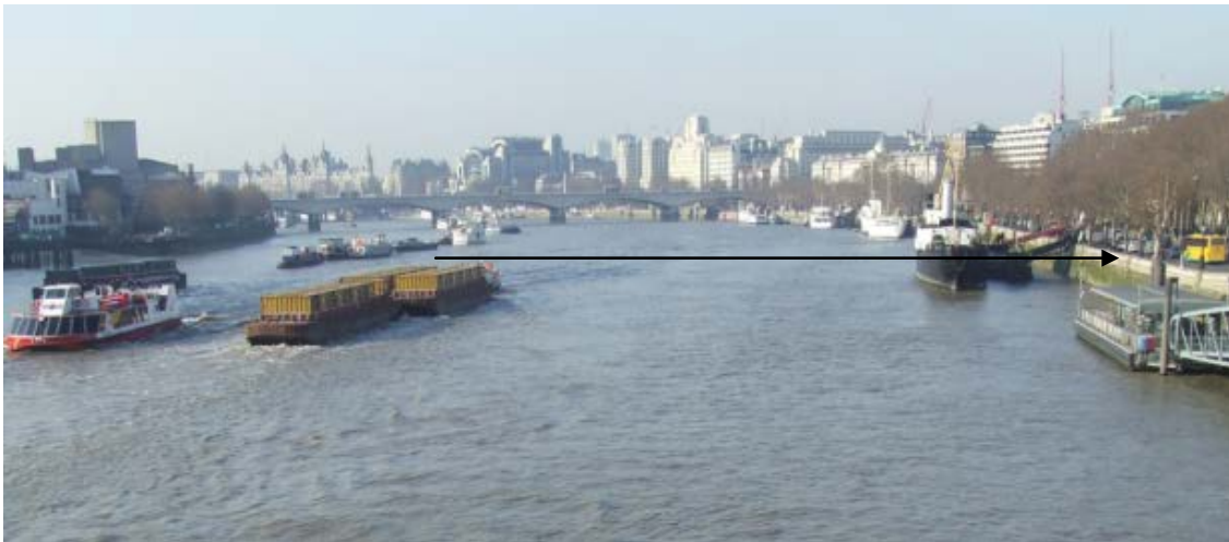
Figure 6.4 Barges through arch No3
