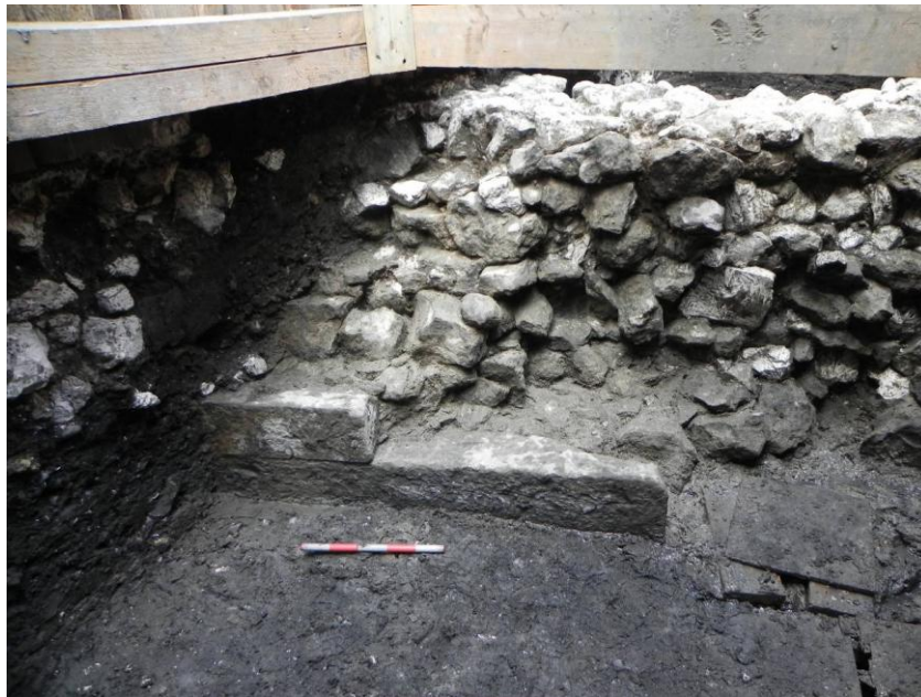
Plate B.1 A medieval revetment at Three Quays House (City of London). Similar waterfront structures could be preserved on the landwards side of the river wall
