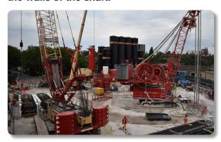
A giant machine called a 'hydrofraise' (pictured) was used to excavate the ground and create each of the 26 shaft wall panels to a depth of more than 60 metres.
