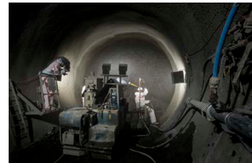
Hammersmith Pumping Station
