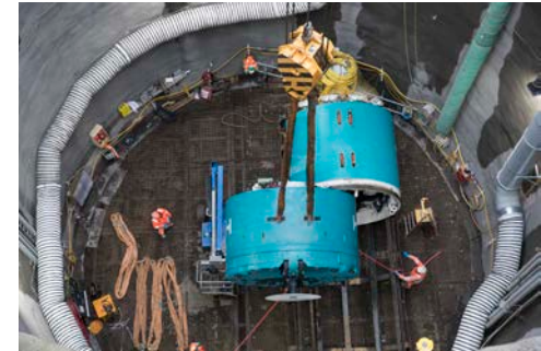
TBM Charlotte lowering at Dormay Street
