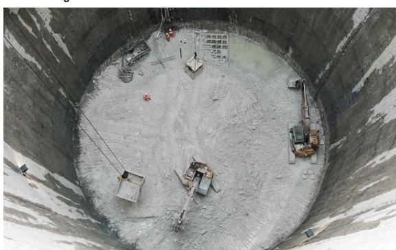
Figure 27.7 Overhead view of construction of shaft for Lee Tunnel
