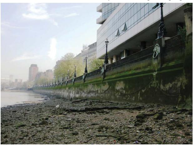
Figure 18.10 Extended section of river wall to the north east of the site, decorated with lion head sculptures containing mooring rings
