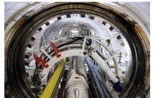
Carnwath Road Riverside
