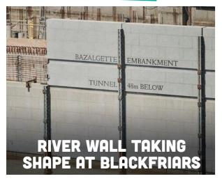
The new permanent river wall at Tideway's site at Blackfriars is beginning to take shape, with the engraved granite facade now visible from the bridge. The new land created in this area is to be named 'Bazalgette Embankment' after the Victorian engineer who designed London's existing sewer network.
