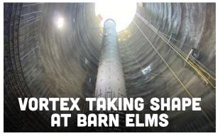
This summer, a giant vortex system was installed into a 34m-deep shaft at Tideway's Barn Elms site, where the team is working to intercept the 'west Putney storm relief' sewer overflow point.
