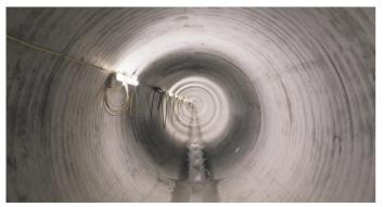
The 1.1km tunnel – known as the Frogmore Connection Tunnel – was excavated in two separate drives between 2019 and 2020, by a three-metrewide tunnel boring machine (TBM) called Charlotte.
