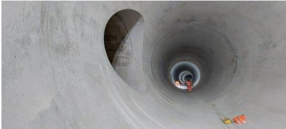
Main Tunnel A secondary lining at Hammersmith junction
