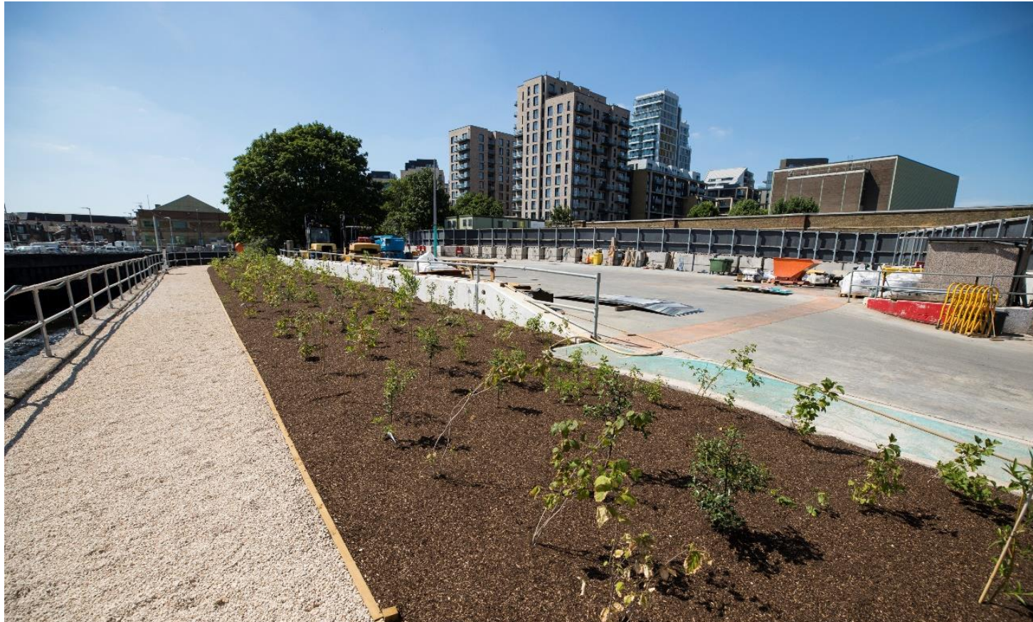
Causeway Island Soft Landscaping complete
