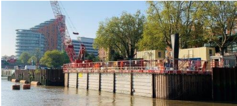
Putney Embankment river wall revealed
