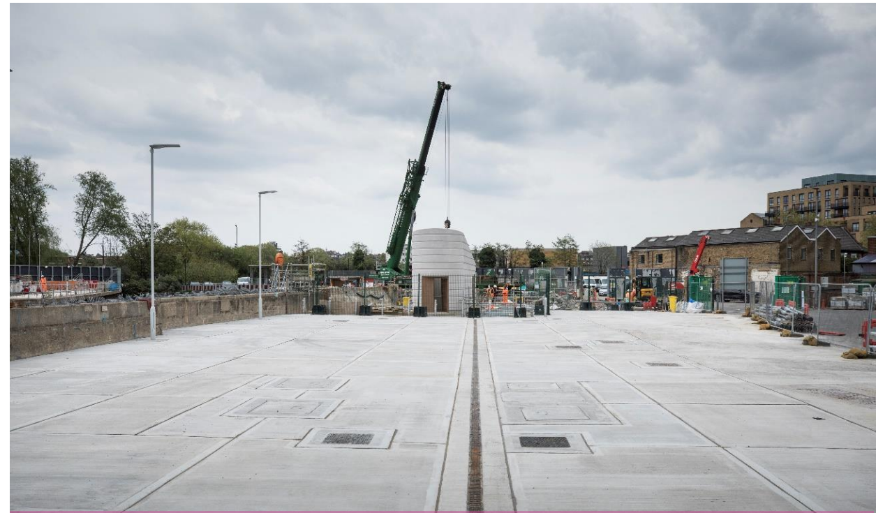
Area A1 Completed paving works and hand back to council
