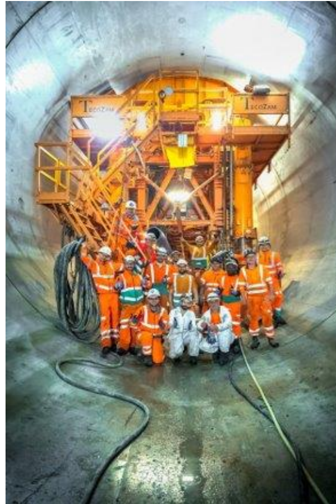
Completion of secondary lining on Central
