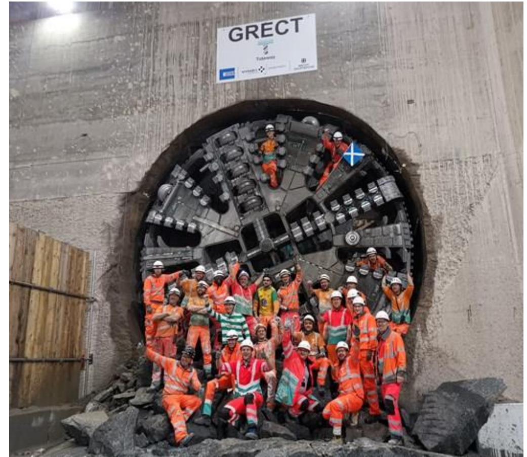
TBM Annie breaks into shaft at Chambers Wharf
