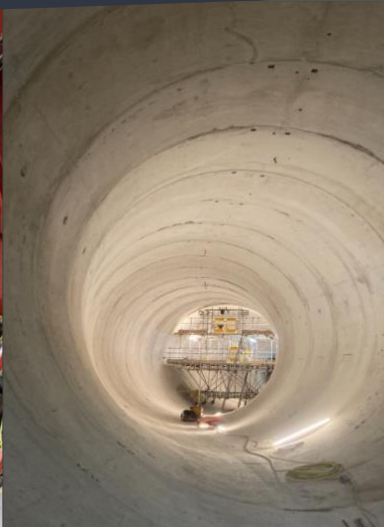
Tunnel after secondary lining (credit: Tideway West)
