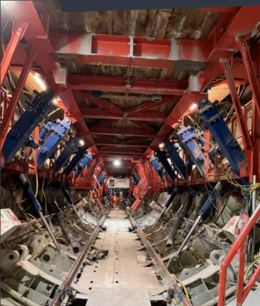
Tunnel Secondary Lining shutter (credit: Tideway West)
