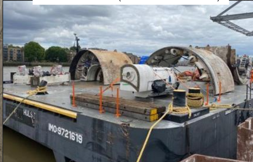
TBM removal, barge loading (Chambers Wharf)
