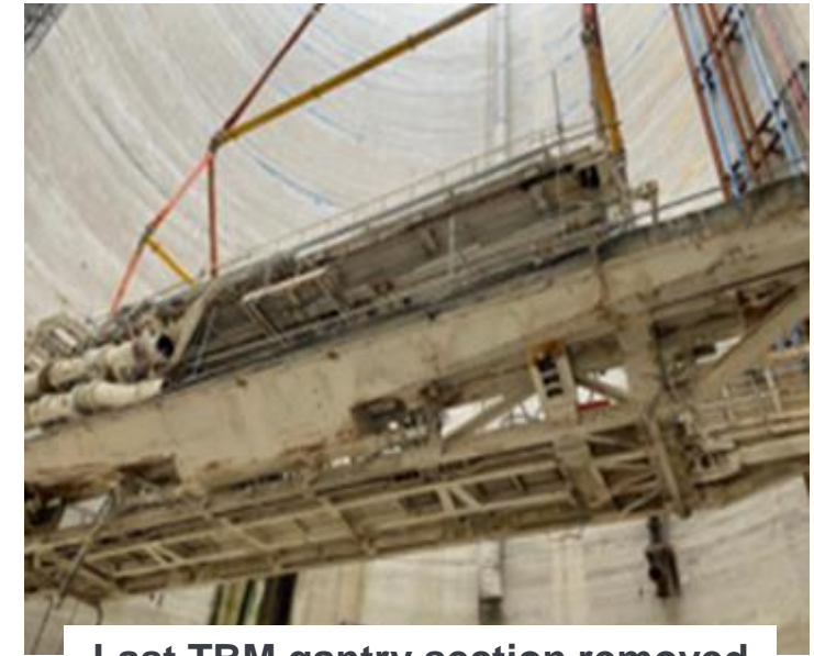
Last TBM gantry section removed from Abbey Mills
