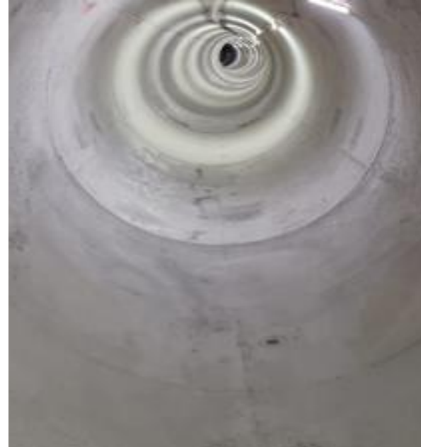
Completed section of secondary lining
