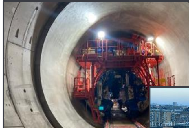
Shutter positioned in the tunnel
