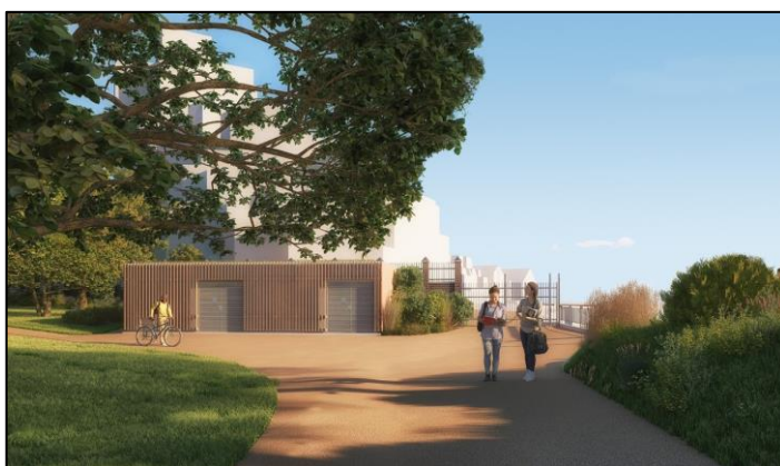
Electrical and mechanical kiosk
