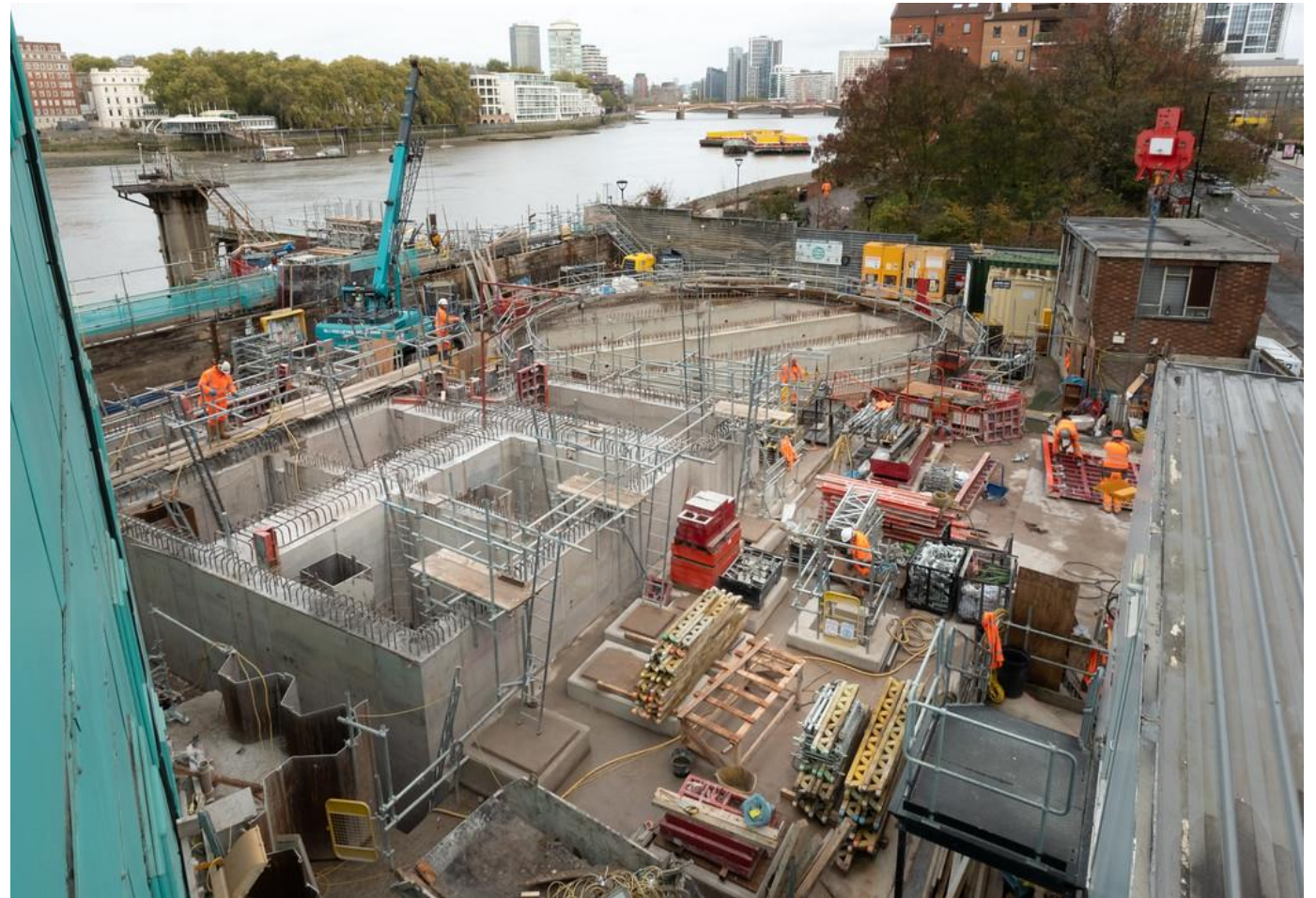
SWSR IC excavation
