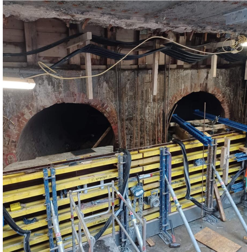
Connection of PS IC to existing Pumping Station
