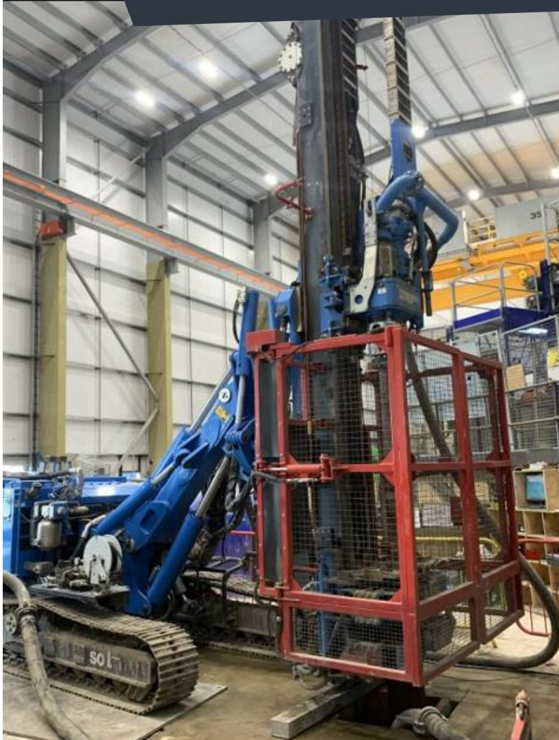
Installation of dewatering wells using drilling rig
