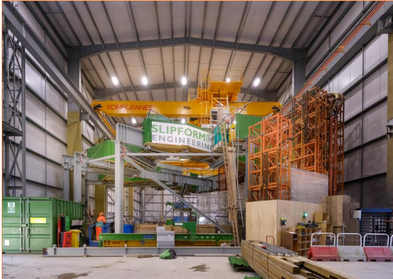
Secondary lining set up under acoustic enclosure at Greenwich
