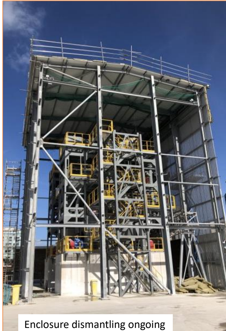
Last elements of Slurry Treatment Plant being removed
