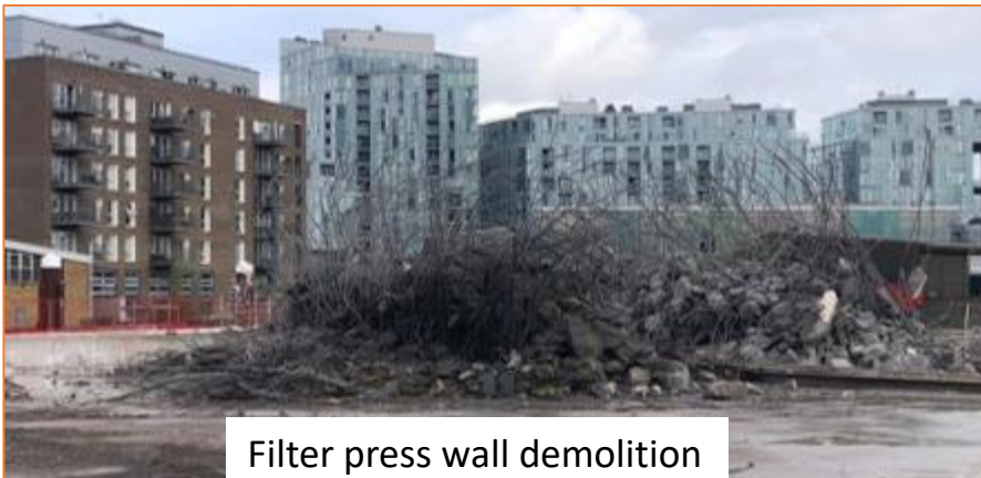
Filter press wall demolition
