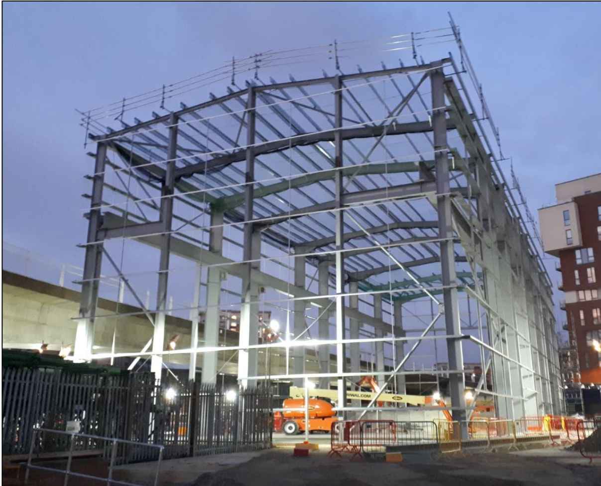
Picture of acoustic enclosure during installation phase, in January 2019
