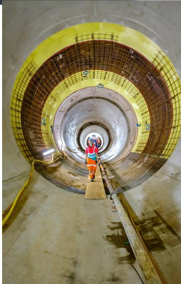
Start of 2 nd lining of Greenwich Connection Tunnel
