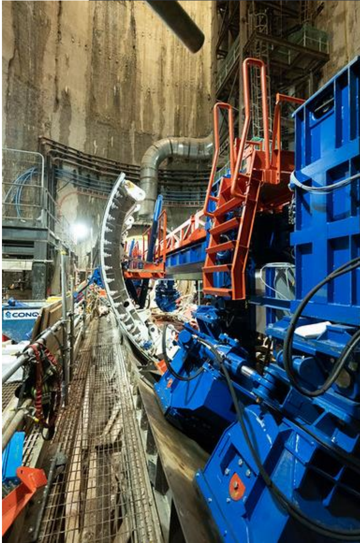
2 nd lining shutter assembled
