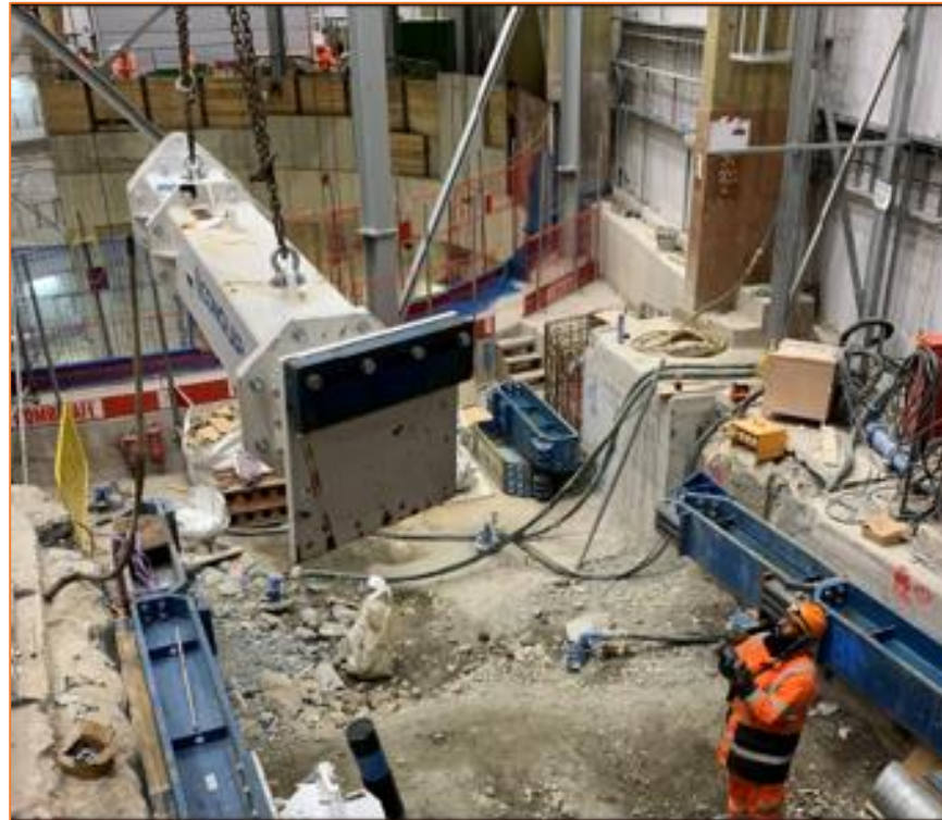
Start of installation of temporary propping (1 st level)
