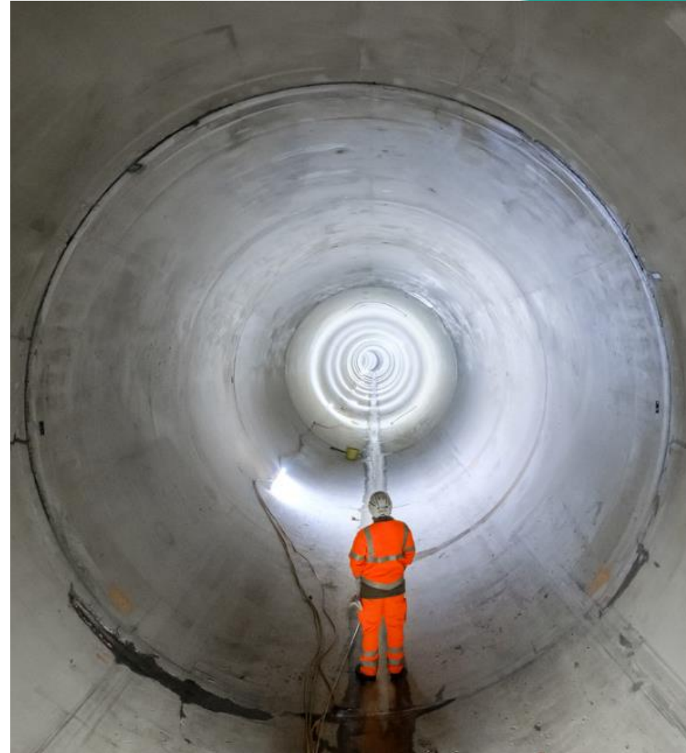
2 nd lining of Greenwich Connection Tunnel – after launch
