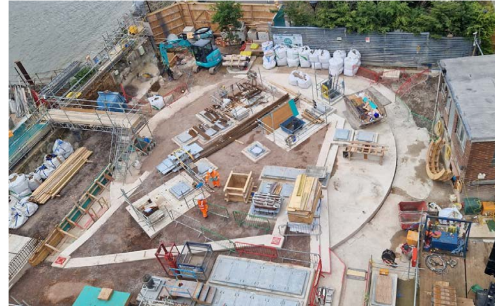
CSO Shaft closed and sub-grade ongoing ahead of asphalt
